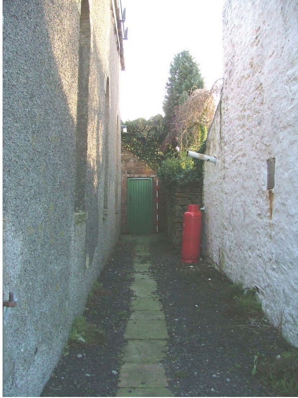
Plate 11 – Alleyway down side of chapel provides access to outbuildings and school room
