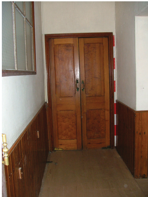
Plate 16 – Doors into main body of chapel from lobby (RH side)
