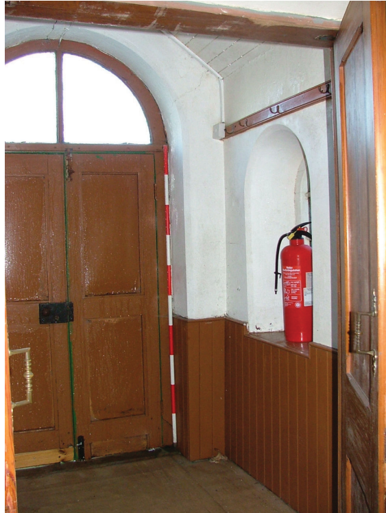
Plate 15 – Interior of porch showing inside of main doors
