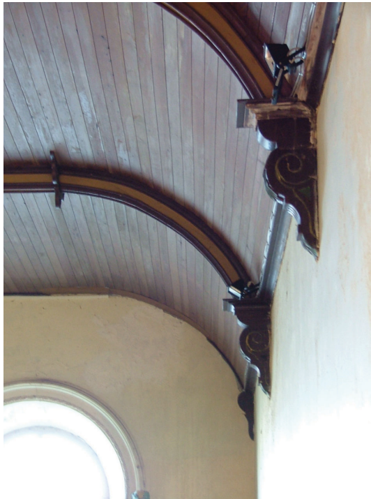
Plate 22 – Detail of timber ceiling
