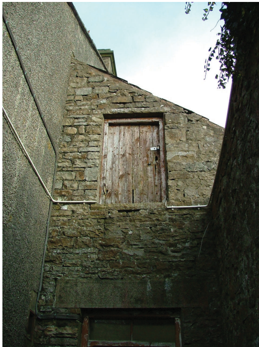
Plate 12 – Doorway to attic space above school room
