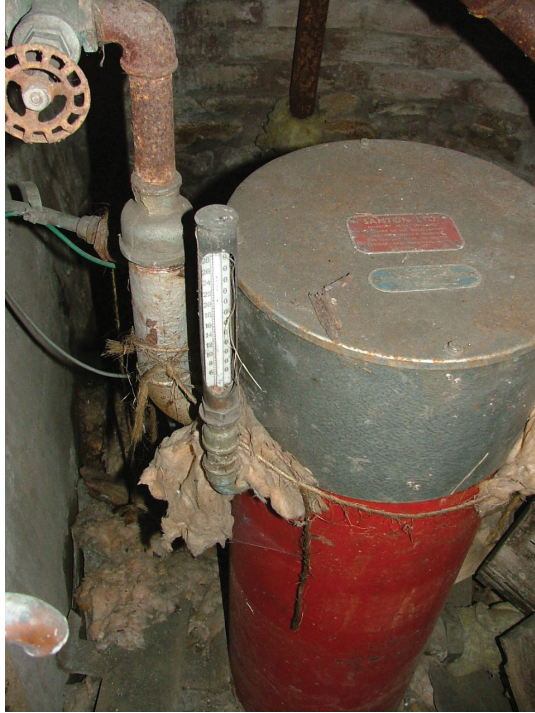
Plate 25 – Boiler Cellar beneath school room
