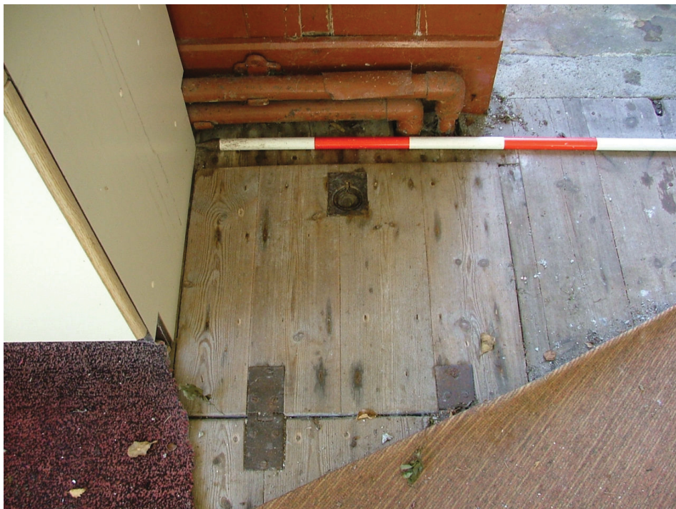
Plate 24 – Hatch in floor of school room provides access to boiler
