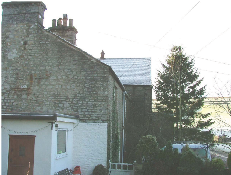
Plate 8 – North-east elevation, largely obscured by the adjoining cottage
