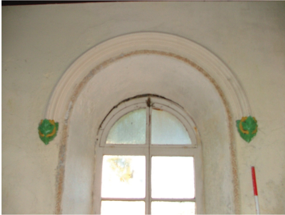
Plate 23 – Detail of decorative window surrounds
