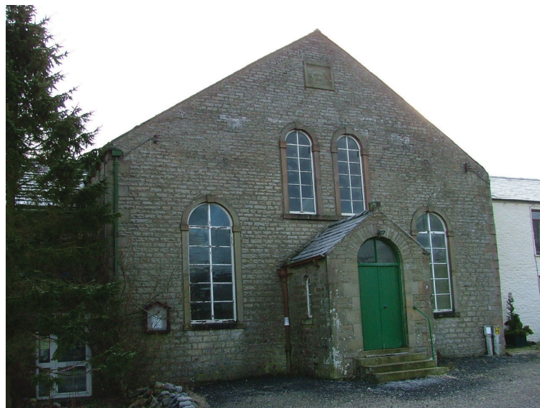
Plate 2 – North-west elevation of Gatehead Chapel
