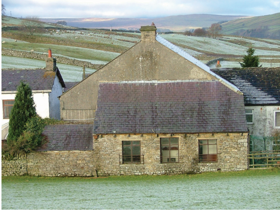
Plate 9 – South-east elevation showing the school room and outbuilding to the rear of the chapel
