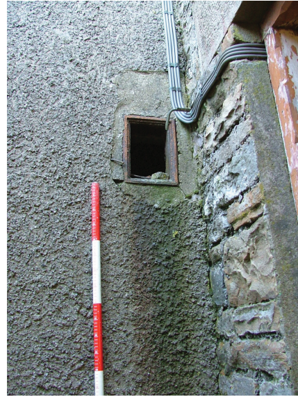
Plate 14 – Iron casing, south-east elevation
