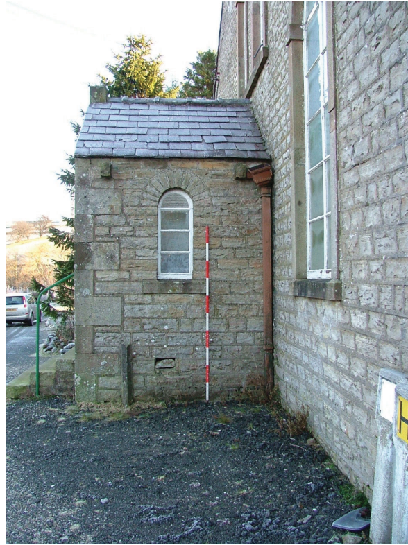
Plate 5 – South-west facing elevation of porch
