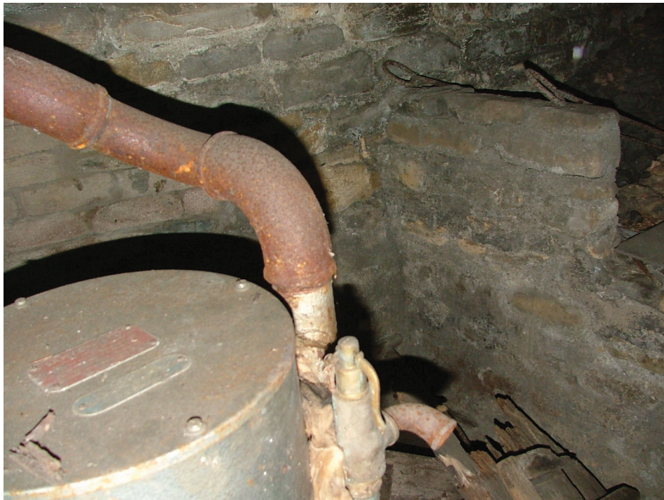
Plate 26 – Brick walls in the cellar and top of boiler
