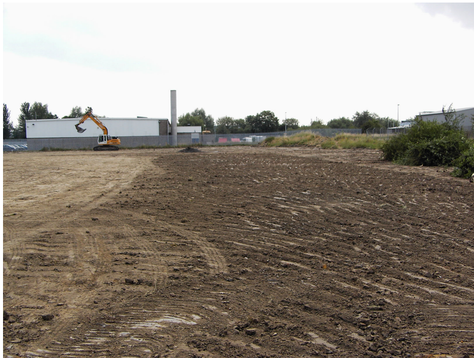
Plate 2. The development site after the topsoil strip, looking south.
