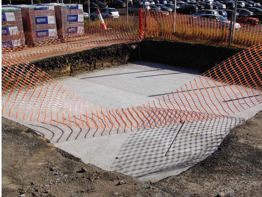
Plate 6. Southern sub-station, looking north-east.
