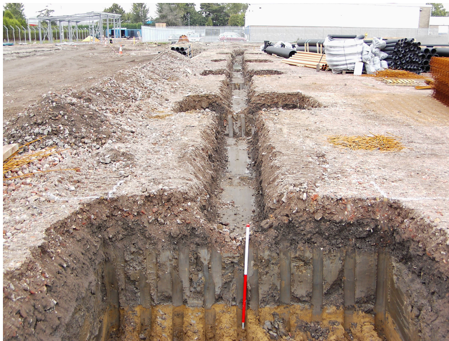
Plate 4. The excavation of the eastern extents of Units 14-19, looking south.
