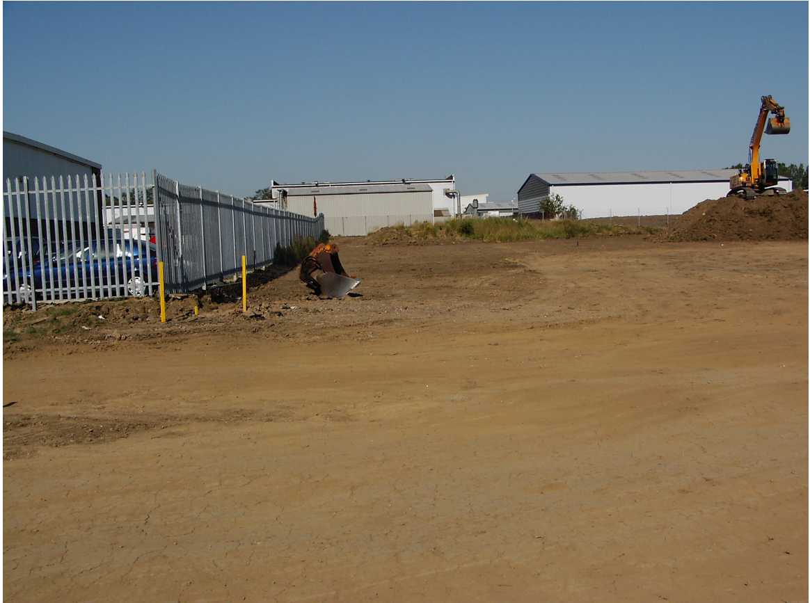
Plate 1. The site, looking west, during topsoil strip.
