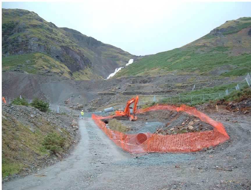
Plate 4: Photograph showing the new location of the stream (culvert) and road to the right
