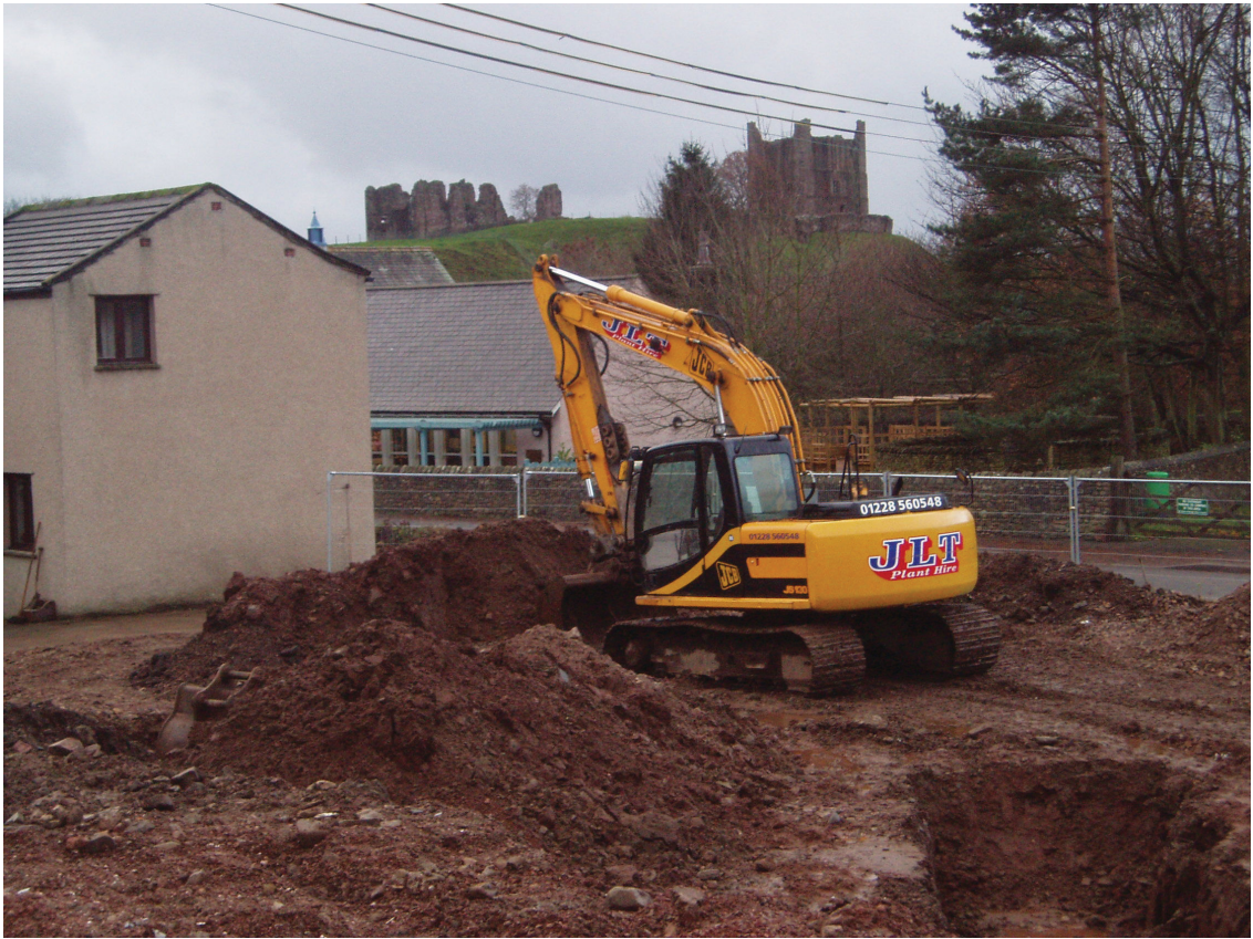
Plate 5: General working shot on site, showing the proximity of Brough Castle.
