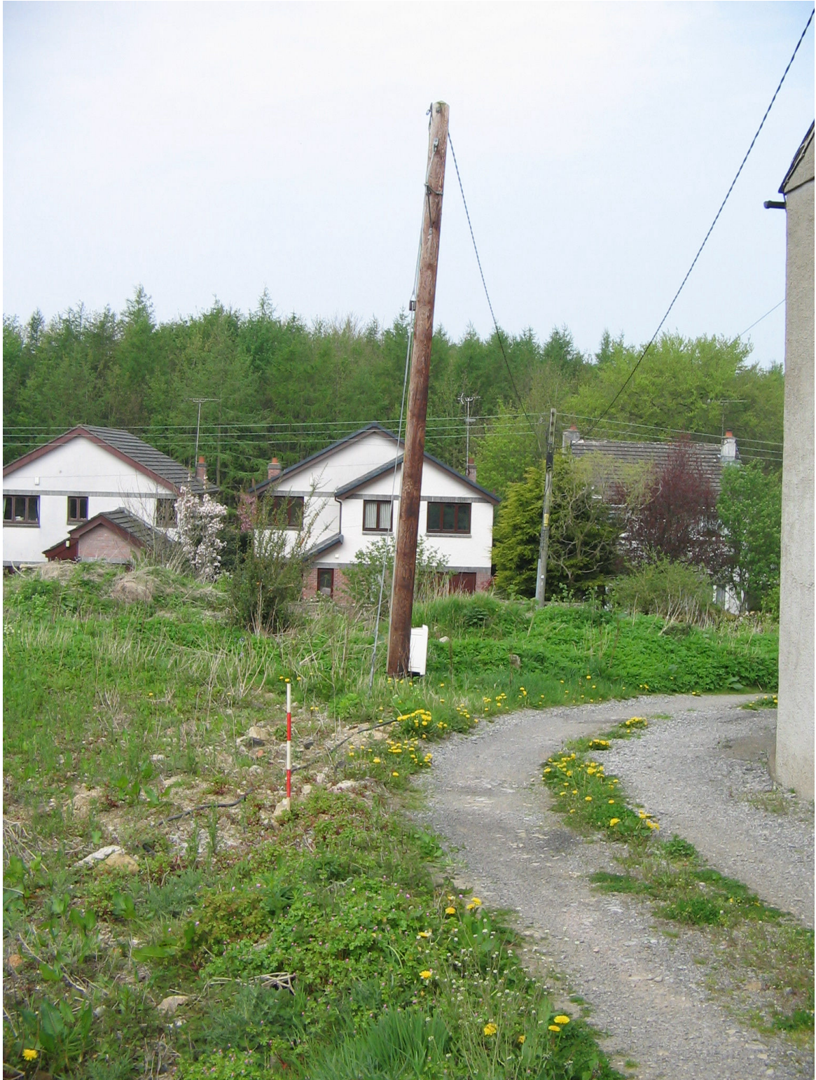
Plate 5: Electricity pole on the northeastern edge of development area, facing northwest.
