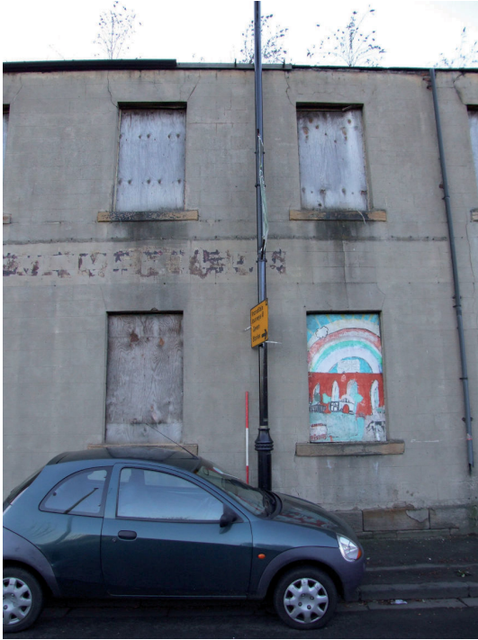
17.) View of elevation 'A2', east-facing.
