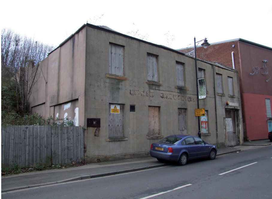
3.) General view of complex front, east-facing.
