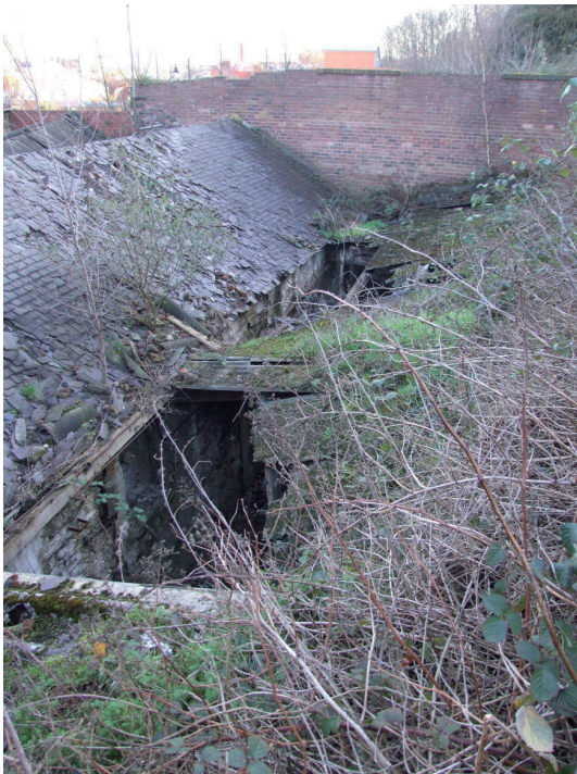
10.) View of complex rear 'C3', northwest-facing.
