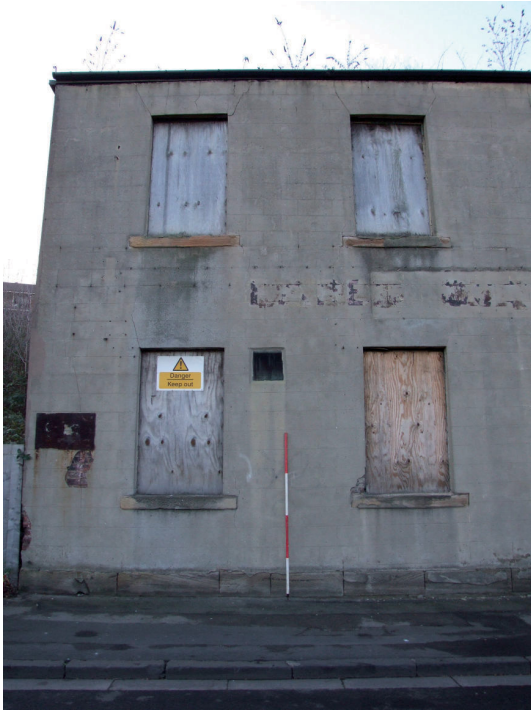
15.) View of elevation 'A1', east-facing.
