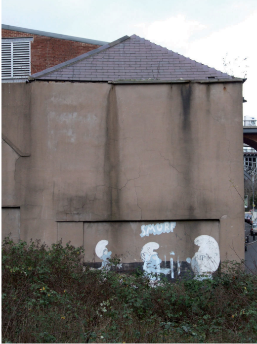
5.) View of Elevation 'A3', south-facing.
