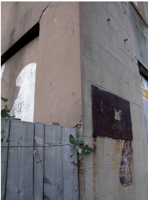
14.) View of the south-east corner of building A, southeast-facing.
