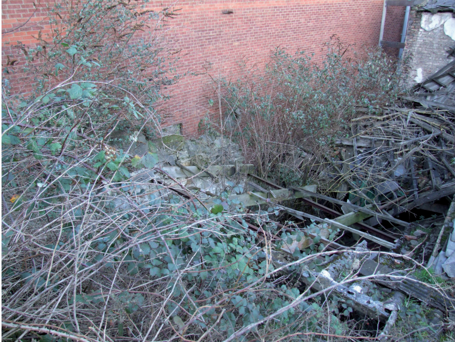
11.) View of complex rear 'C4' and B, south-facing.
