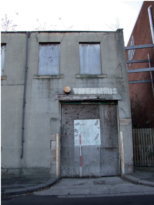
18.) View of elevation 'B1', east-facing.
