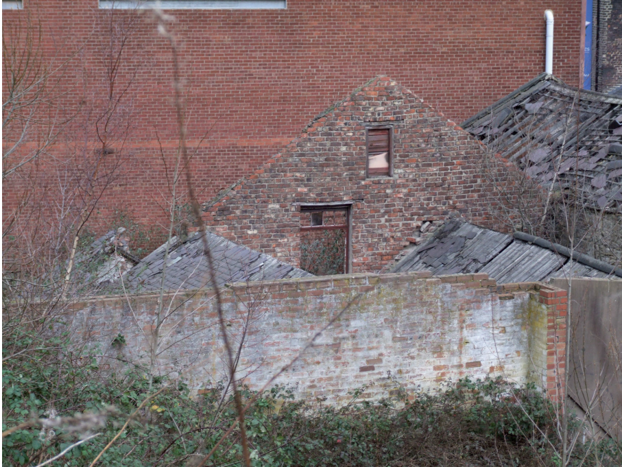
7.) View of Elevation 'C2', south-facing.
