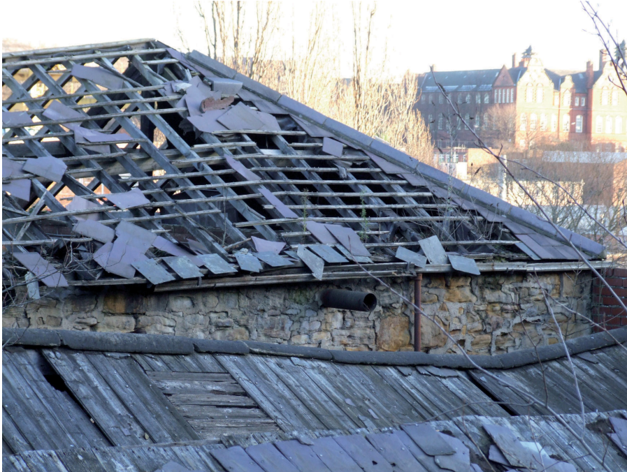
13.) Close up view of rear stone wall of building A, west-facing.
