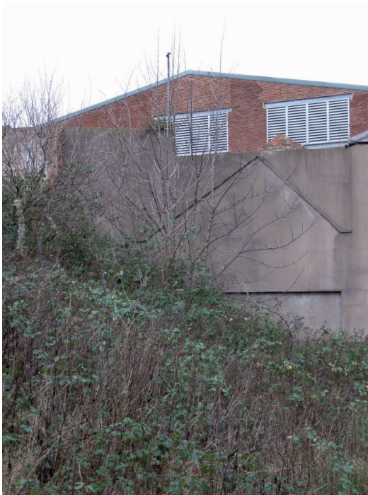
6.) View of Elevation 'C1', south-facing.
