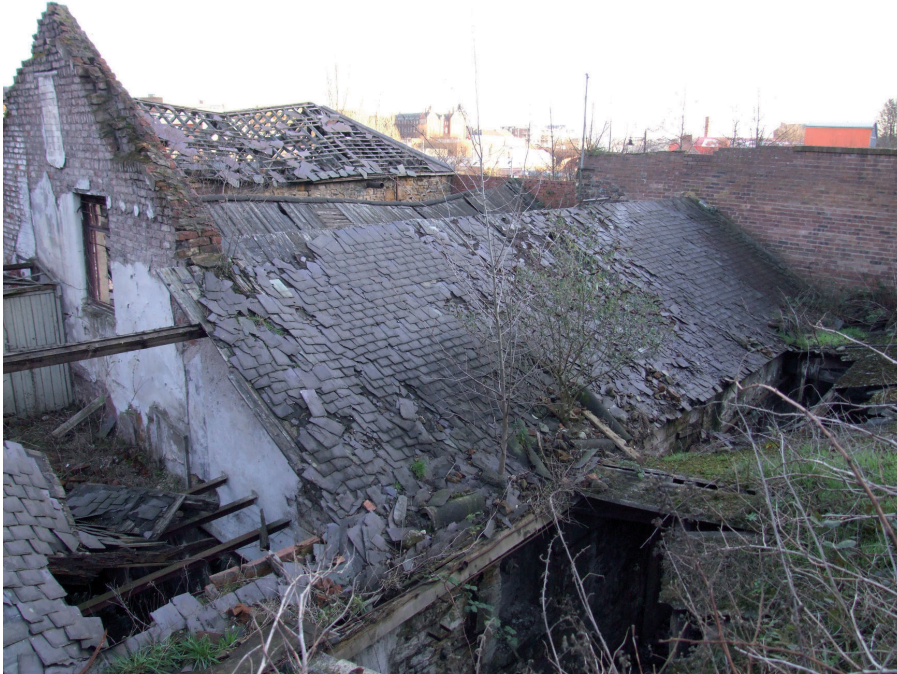
9.) View of complex rear 'C3', northwest-facing.
