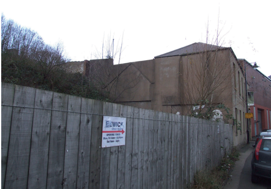
4.) General view of south elevation, south-facing.
