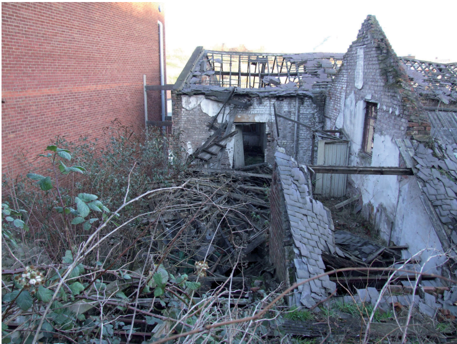
8.) View of complex rear 'C4' and B, west-facing.
