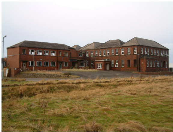
Plate 7: View of extant office buildings
