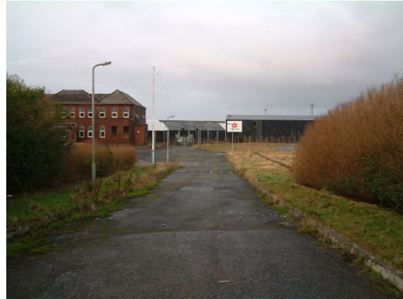
Plate 6: View of track way leading to bridge over the railway lines
