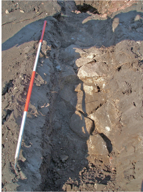
Plate 5: Broken Sandstone Capstones of Culvert Feature [105] in Trench 6, Facing East.
