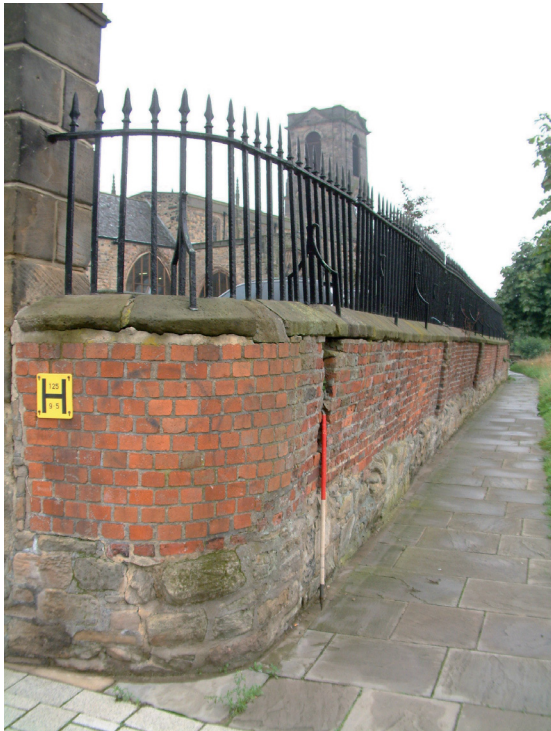
Plate 2. The section of boundary wall to be rebuilt, looking southwest.
