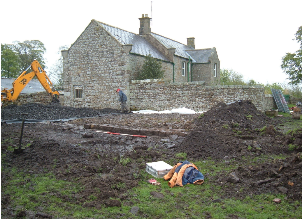
Plate 1: Excavation area, looking northeast towards Carraw Farm.
