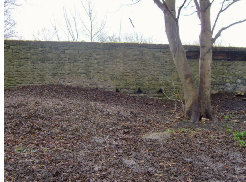
Plate 15: View of northern tithe barn wall from the north
