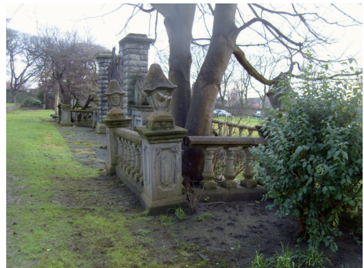
Plate 19: View of Whitburn Hall garden features facing east
