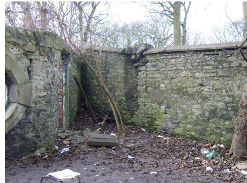
Plate 13: View of boundary between oval featured wall and Rector's boundary wall
