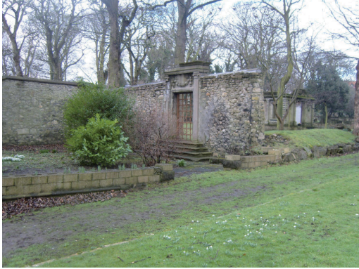
Plate 20: View of wall at north of development site from south-west
