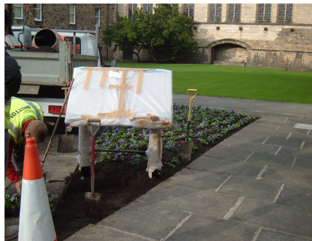
Plate 3: The Site After Works
