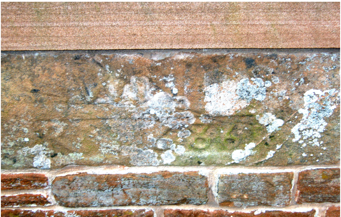
Plate 5: Re-used door/window lintel from the original school building, constructed into the fabric of the later modern school, W (William) N (Nicholson) 1686
