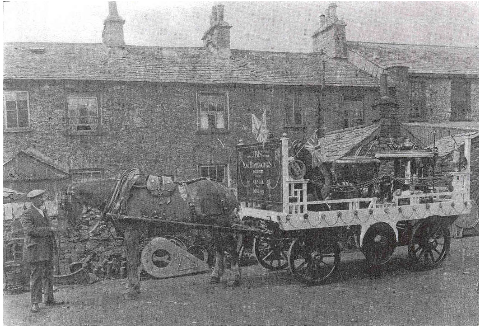
Plate 5: IBIS float standing in the yard. The buildings that can be seen form the back of Ann Street. The photograph is probably early 20 th century. (From Duff, 1997).
