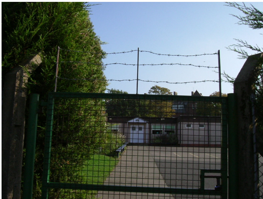
Plate 2: The temporary classrooms, image taken from the north
