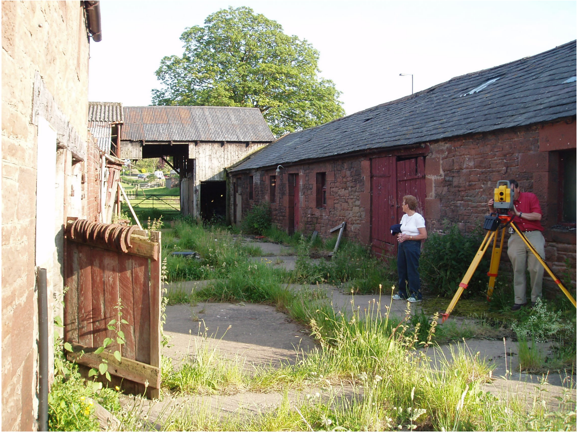
Plate 6: Looking southwest down the range of buildings, showing the overgrown concrete yard and the slate roofs on the buildings that front the road.
