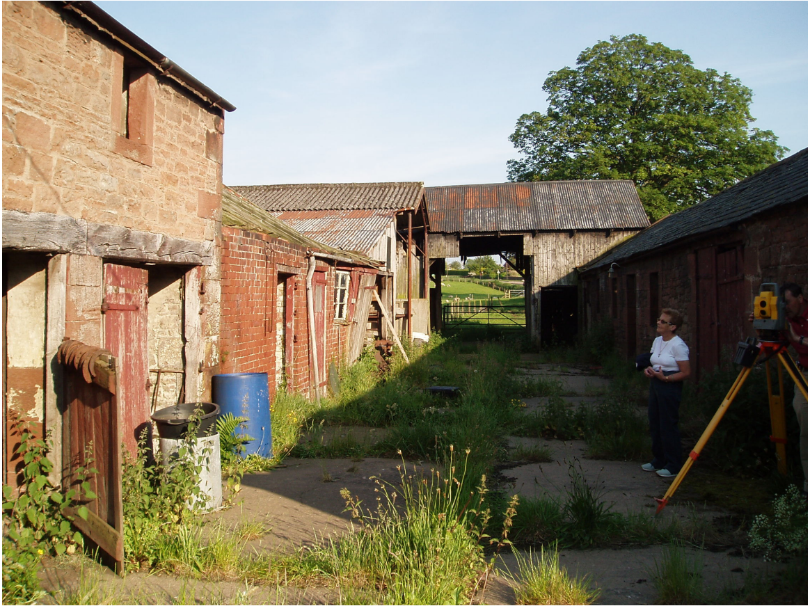
Plate 5: Looking southeast down the range of buildings to the later addition of the plank and corrugated roof barn at the end.
