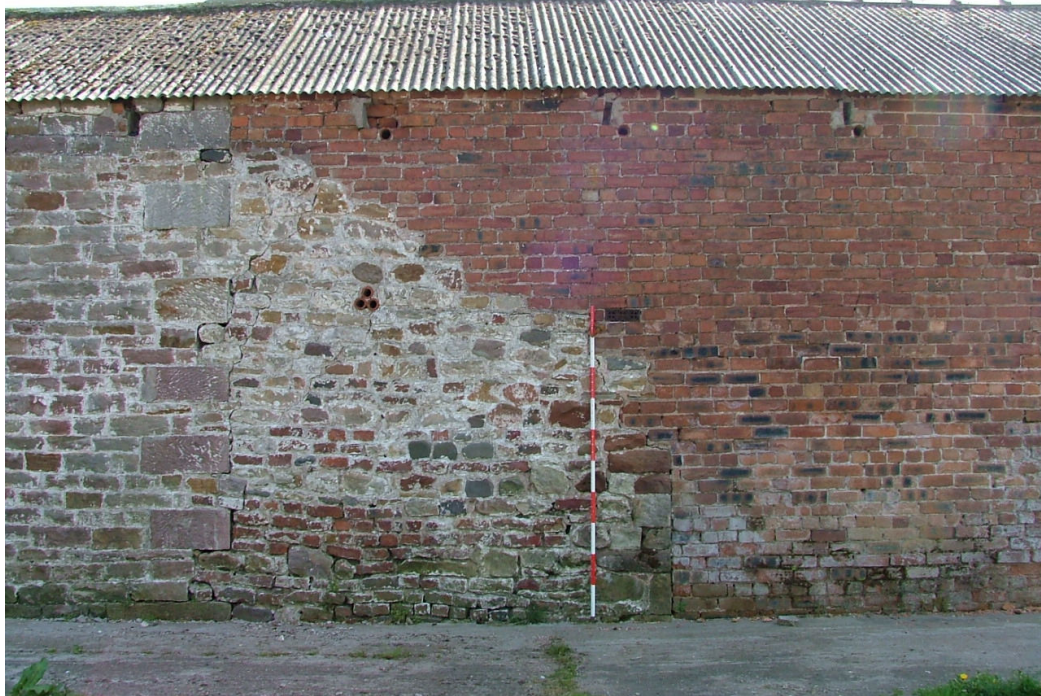
Plate 6 – Possible lean-to, west elevation of Building A
