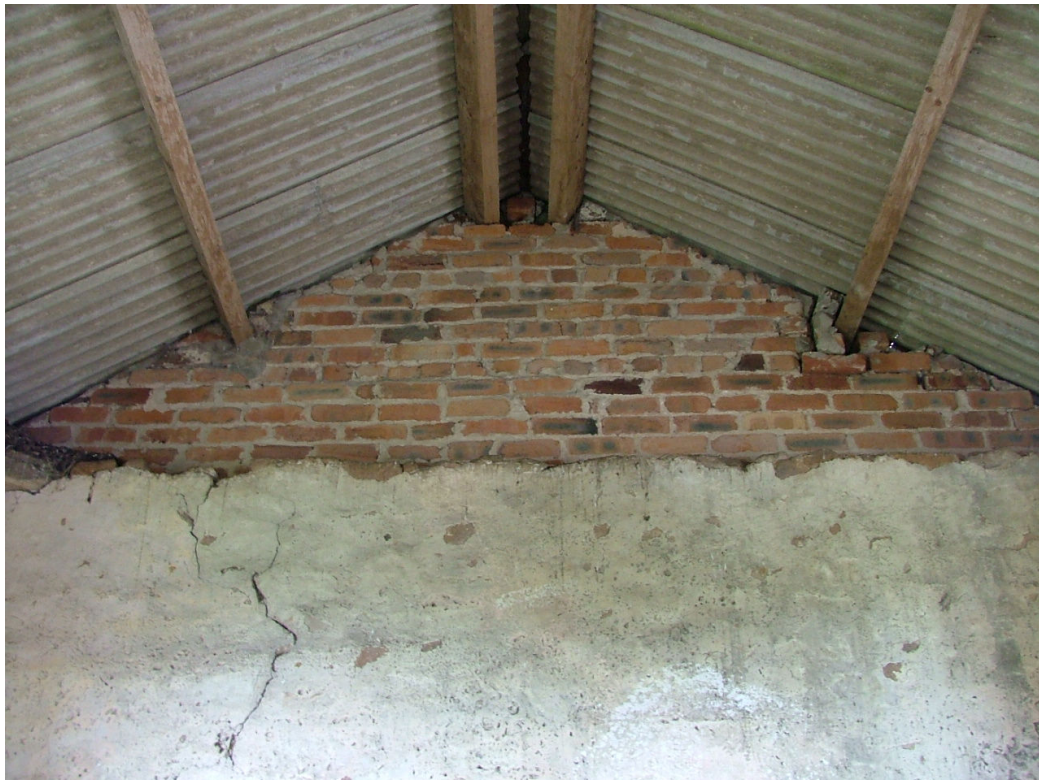
Plate 17 – Interior of Building A, heightened wall between masonry section and brick extension
