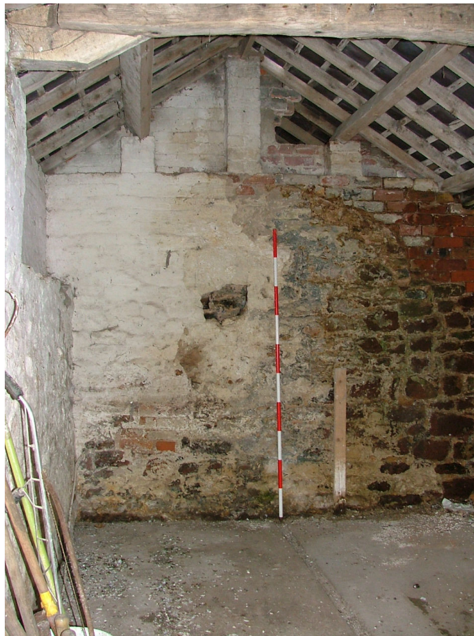
Plate 31 – Interior of Building C showing masonry and brick dividing wall
