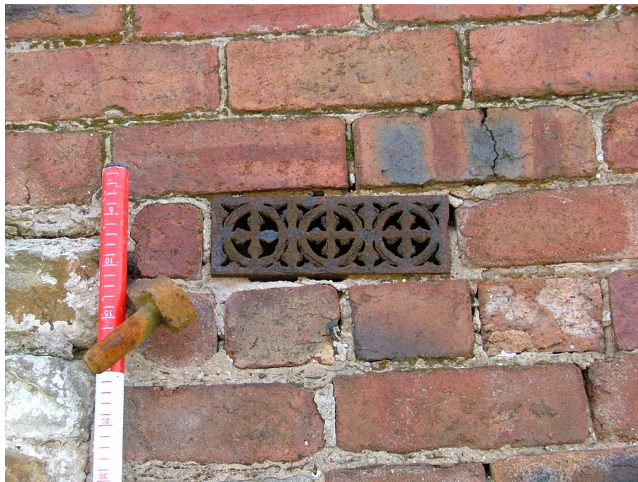
Plate 8 – Decorative iron ventilation plate, southern end of west elevation of Building A (red section of ranging pole measures 20cm)
