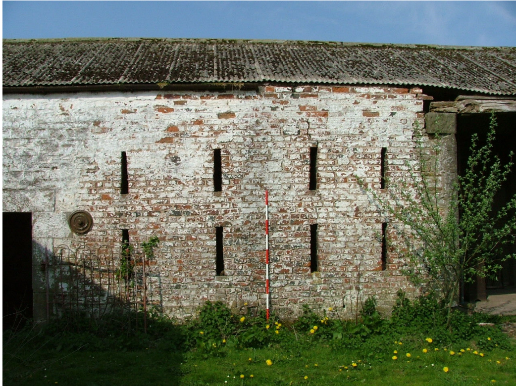
Plate 11 – Ventilation slits and tie-plate, eastern elevation of Building A
