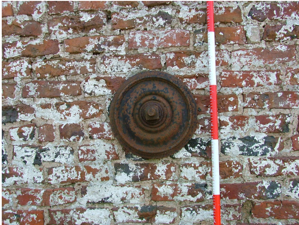
Plate 4 – Circular iron tie plate, western elevation of Building A (the ranging pole is divided into 20cm sections)
