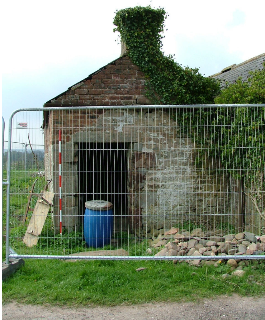
Plate 28 – Northern elevation of Building C showing earlier gable end, doorway and chimney
