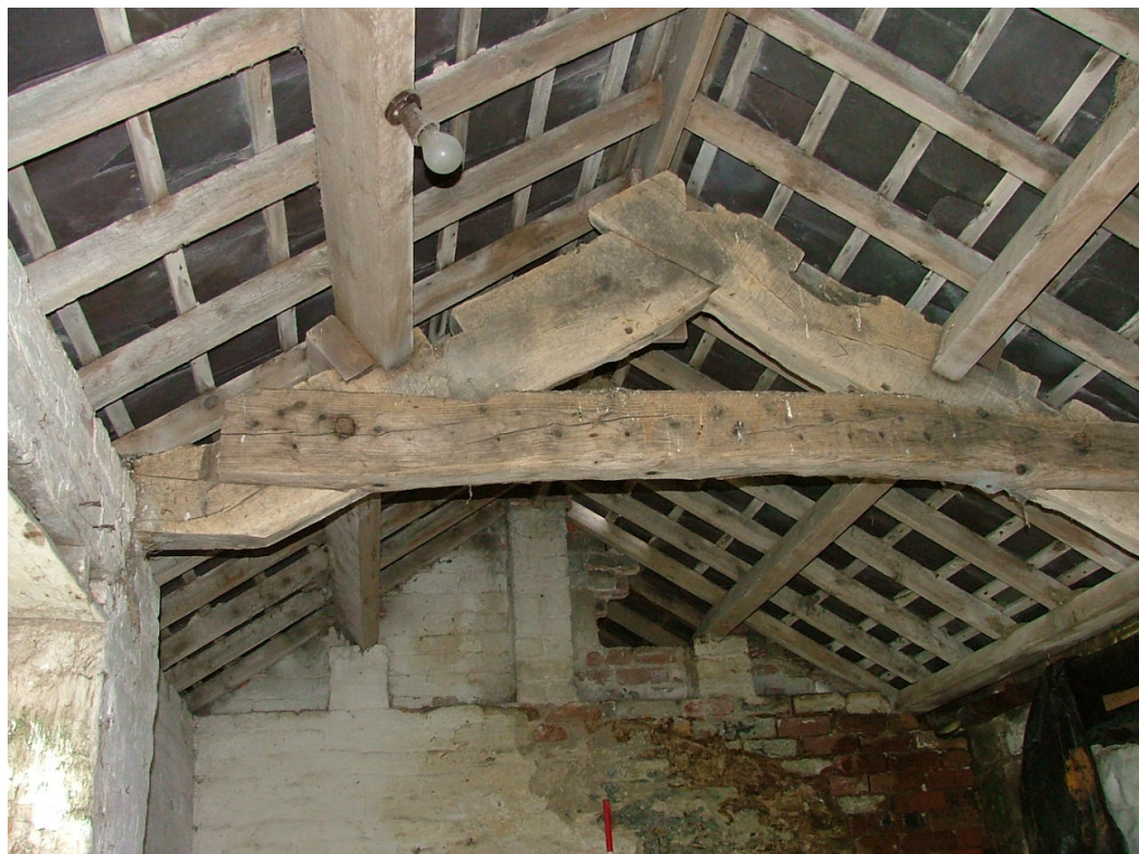
Plate 33 – Collar beam truss, northern room of Building C
