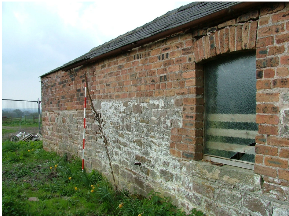
Plate 27 – East elevation of Building C, the change in masonry can be observed close to the ranging pole
