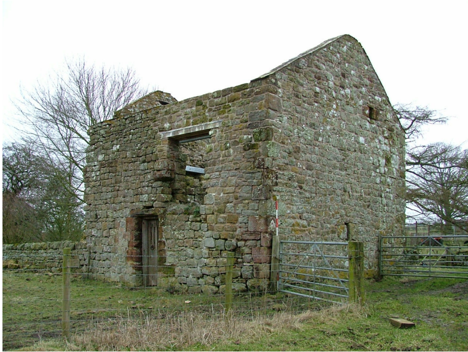
Plate 3 - 'Vicar's Pele', Upper Denton, as seen from the north-west
