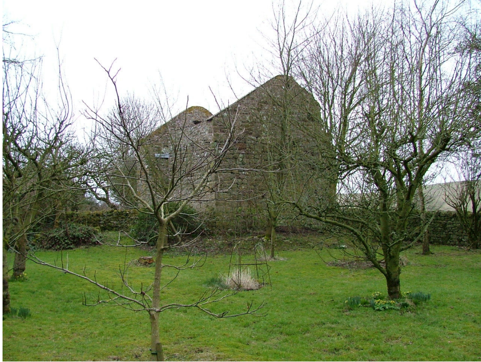
Plate 6 – Eastern elevation of the bastle house as seen from the garden of Low Town Farm
