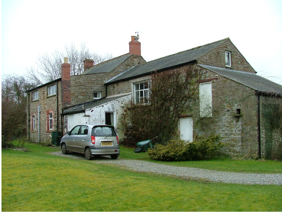
Plate 4 – Northern elevation of Low Town Farm from west
