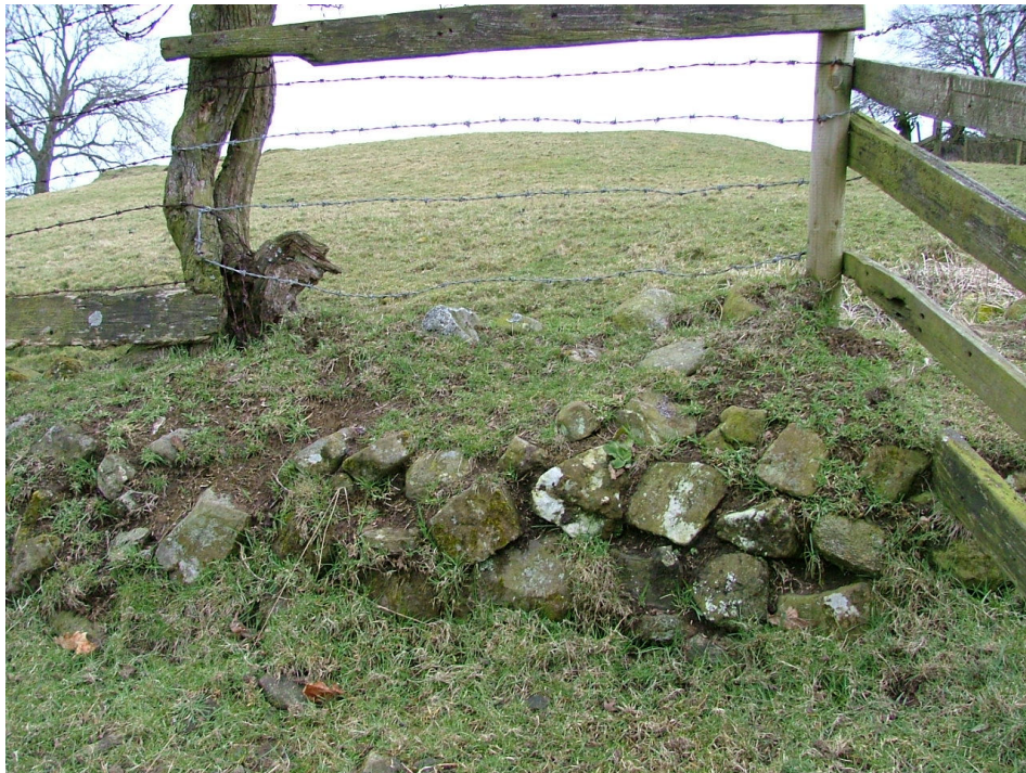
Plate 12 – Part of the hedge-bank field boundary in the field to the north of Low Town Farm. Constructed from earth and rubble masonry with hawthorn bushes planted on top
