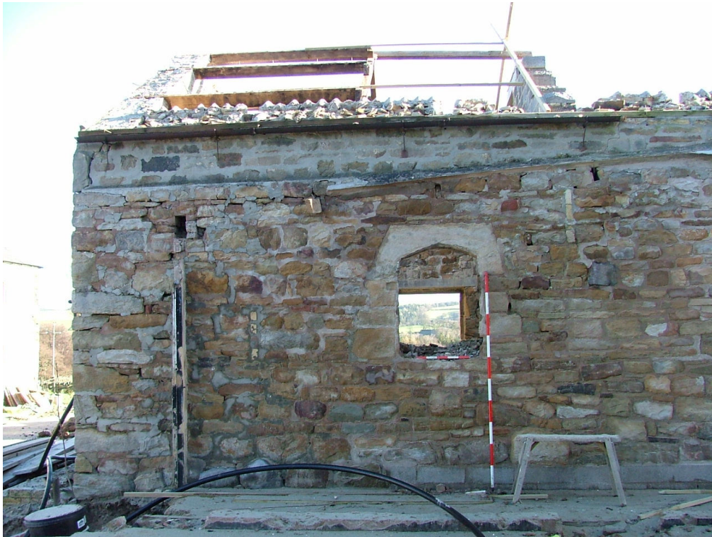
Plate 6 – North end of west elevation (Large scale = 2 metres, small scale = 0.50 metres)
