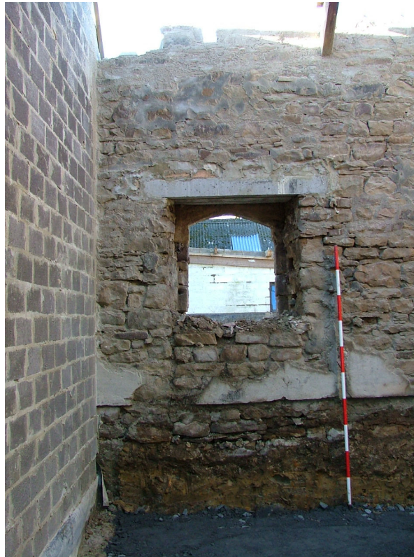
Plate 14 – West elevation, interior of window
