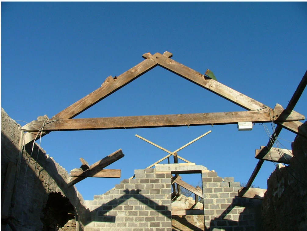
Plate 13 – View looking north of remaining roof trusses
