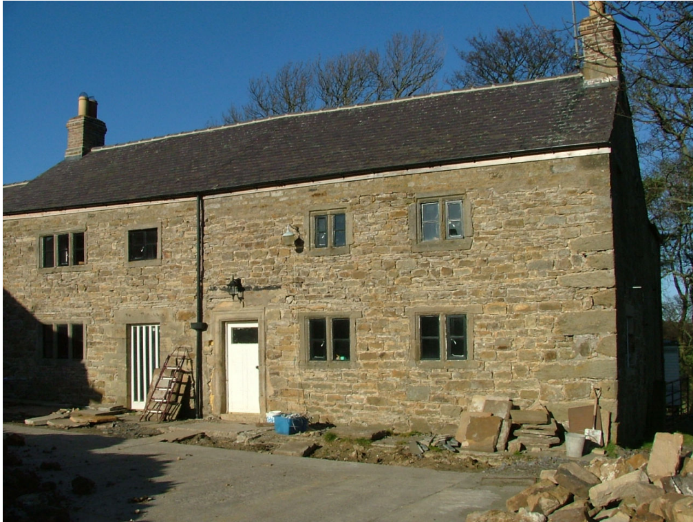
Plate 18 – South elevation of farmhouse
