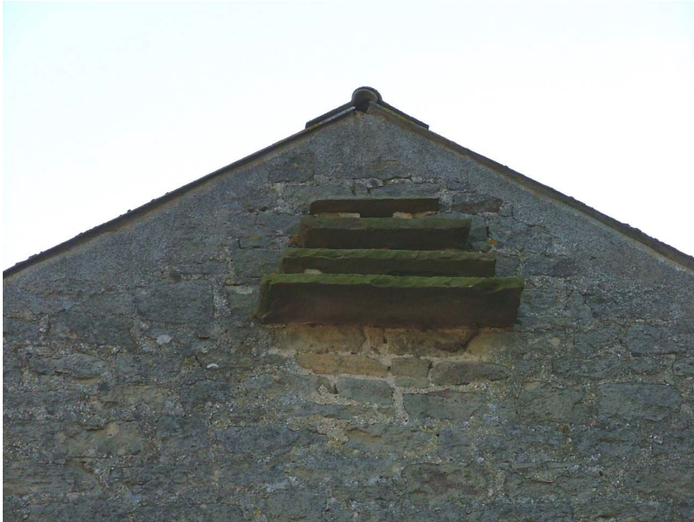
Plate 22 – Nesting boxes, north gable of hay barn
