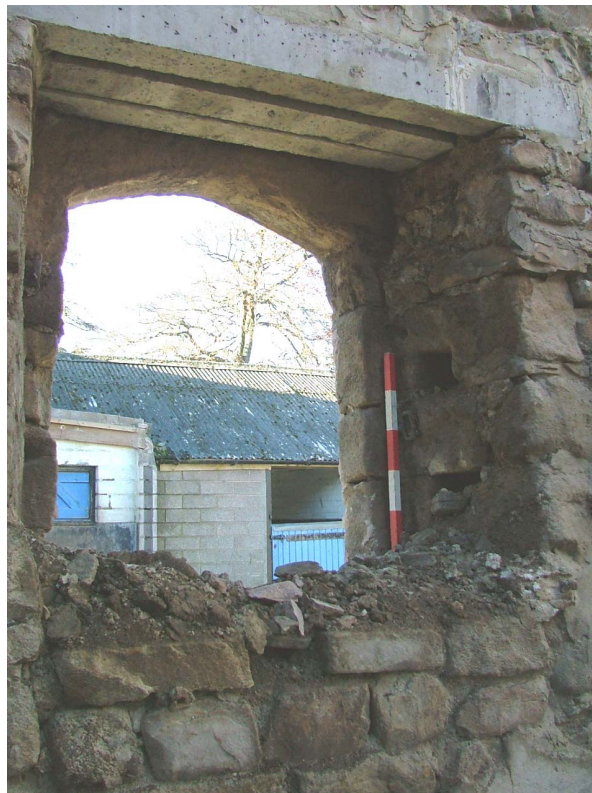
Plate 15 – Interior of window, west elevation, showing possible holes for metal or wooden bars? (Scale = 0.50 metres)
