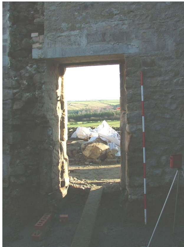
Plate 11 – View looking east showing scarring of former cross-wall (left of photograph)
