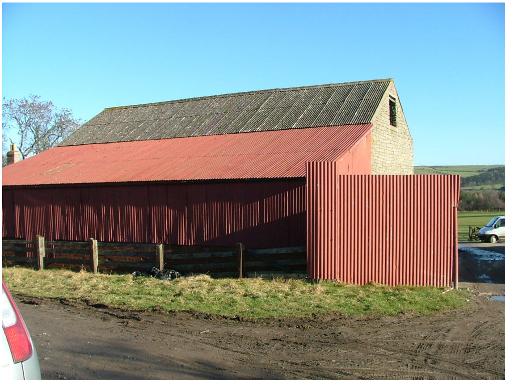
Plate 25 – Corrugated sheet building against the west elevation of hay barn
