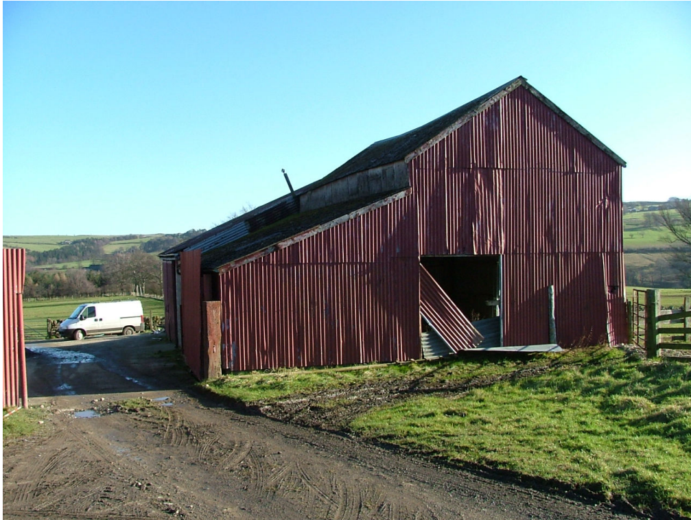
Plate 24 – Corrugated iron sheet building, south side of site
