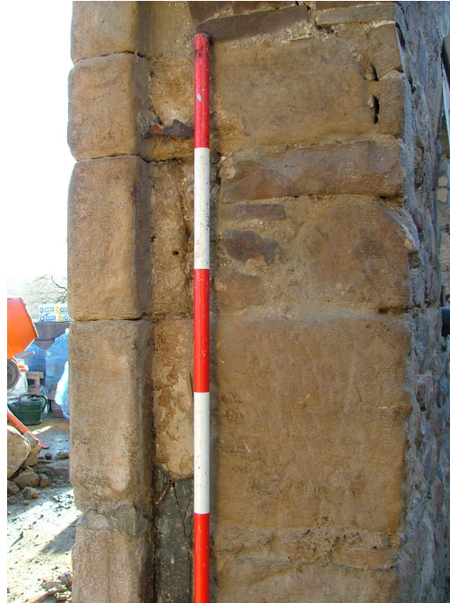
Plate 16 – Detail of doorjamb, east elevation
