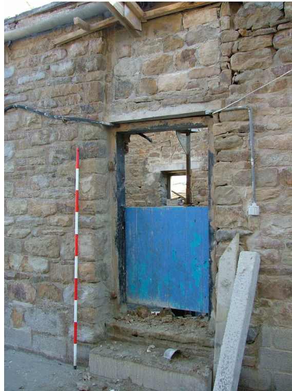
Plate 8 – Doorway, west elevation
