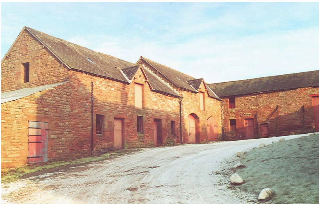
Plate 1 – South facing elevation of Building ‘A’ (left side of photograph)
