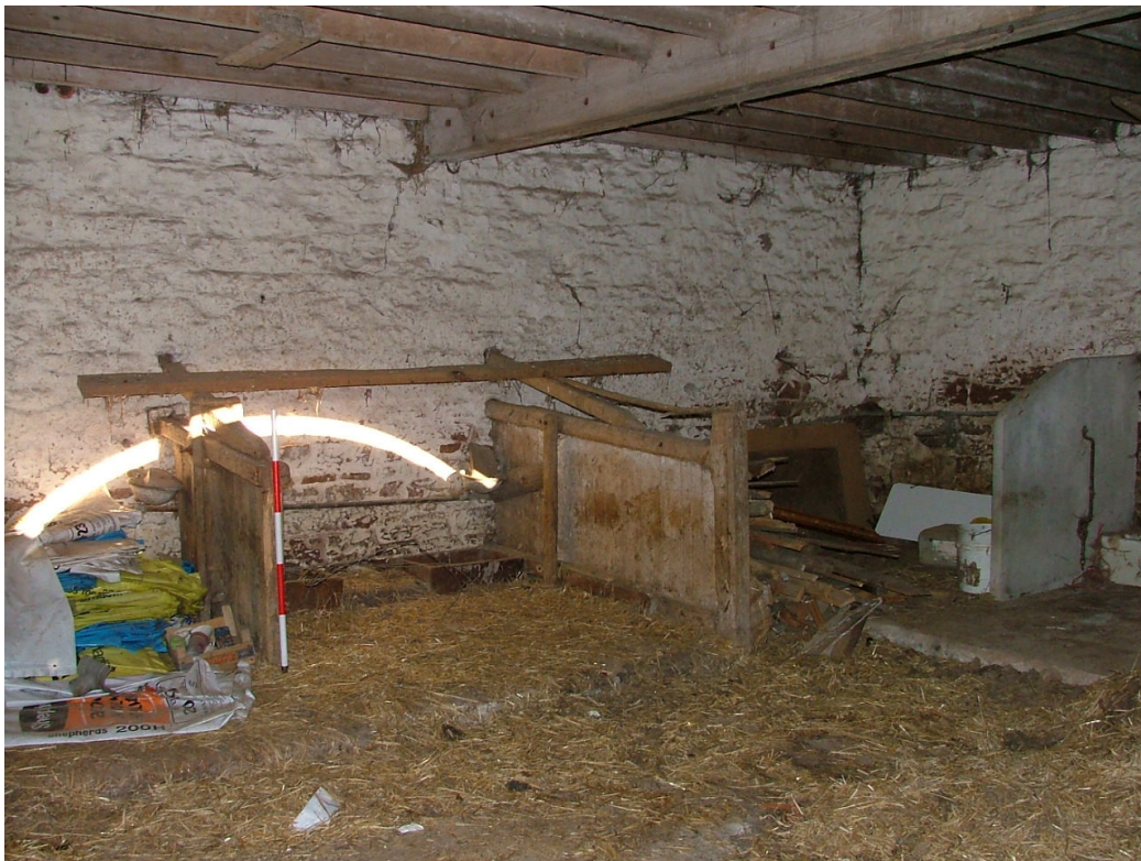
Plate 14 – Interior of cart shed, Building A
