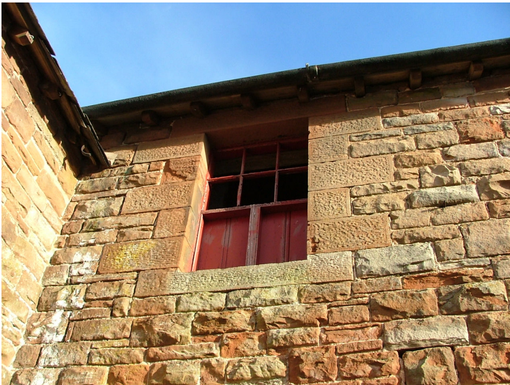
Plate 23 – First floor window, western elevation of Building B
