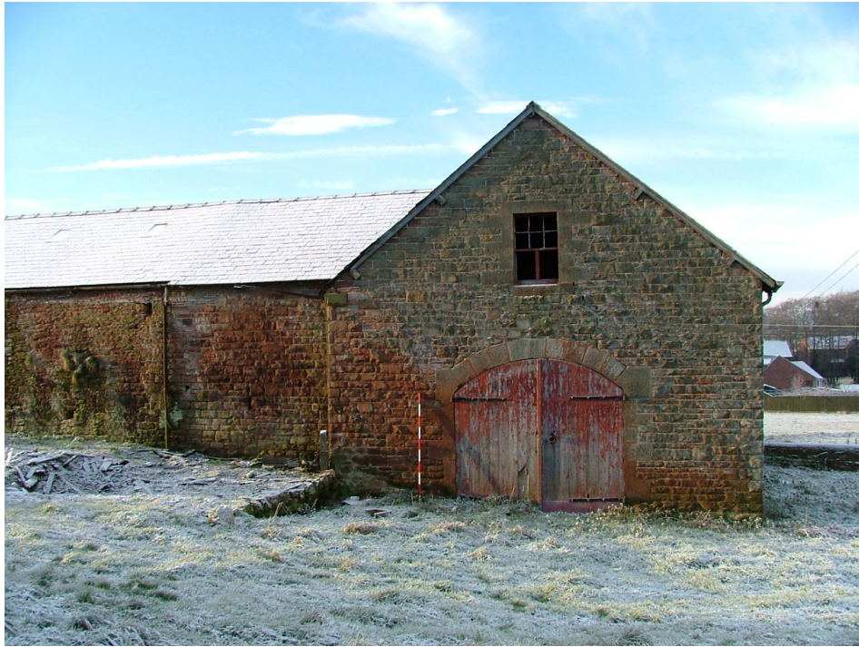
Plate 7 – Eastern gable end of Building A
