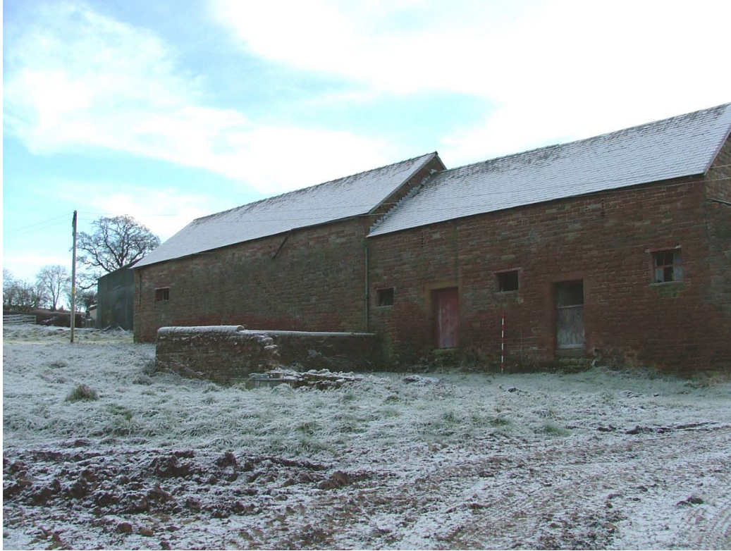
Plate 6 – Northern elevation of Building A
