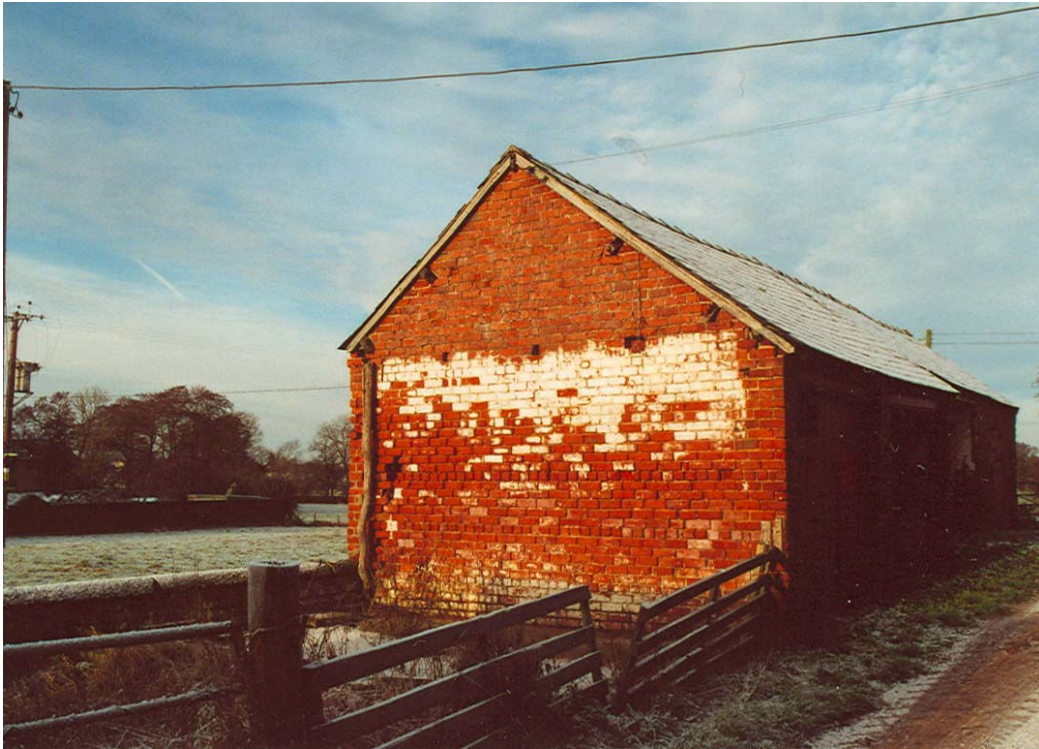
Plate 25 – Brick-built building, western side of site
