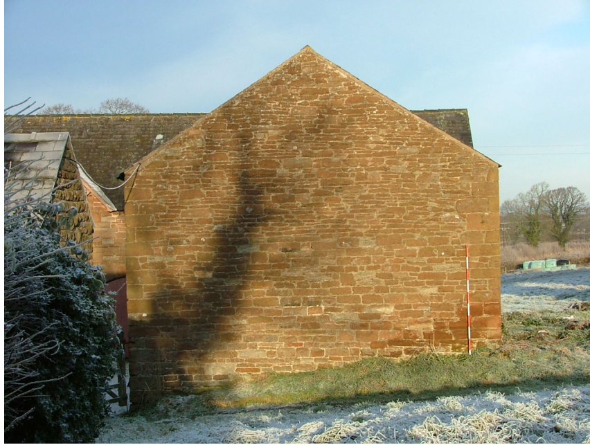
Plate 10 – Southern gable end of Building B
