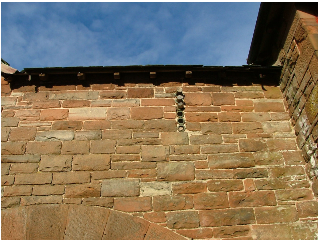
Plate 5 – Detail of ventilation slit, southern elevation of Building A
