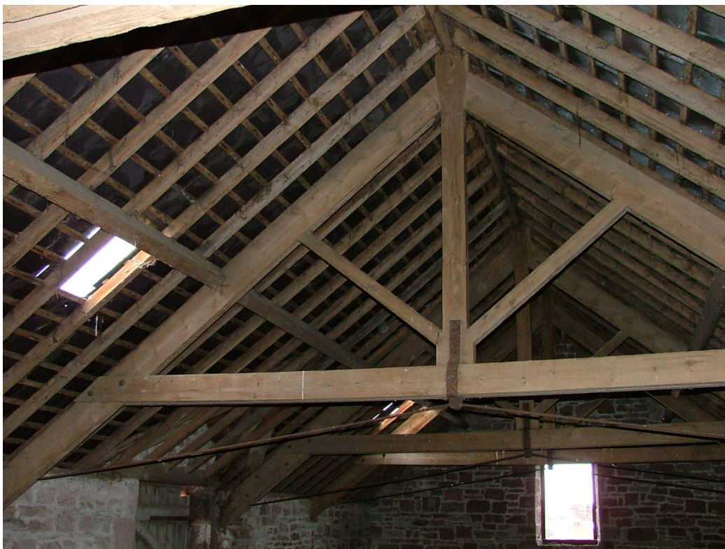
Plate 17 – Detail of roof structure, first floor of Building A
