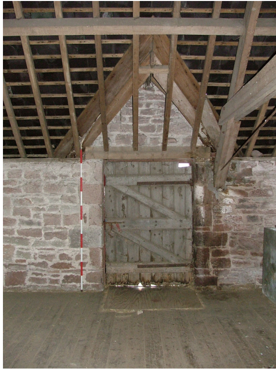
Plate 18 – Detail of gabled dormer with pitching door
