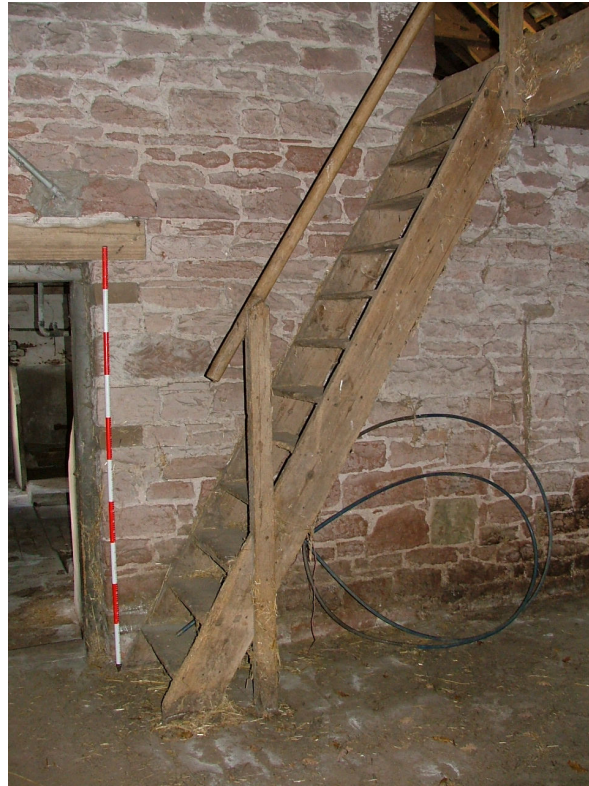
Plate 13 – Wooden stairs to hayloft, cart shed in Building A
