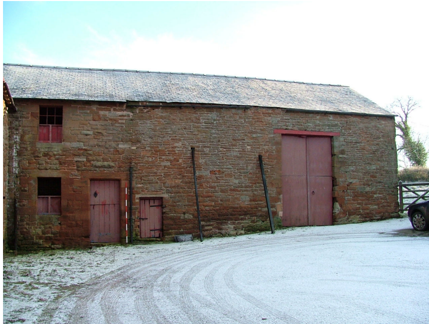
Plate 8 – Western elevation of Building B
