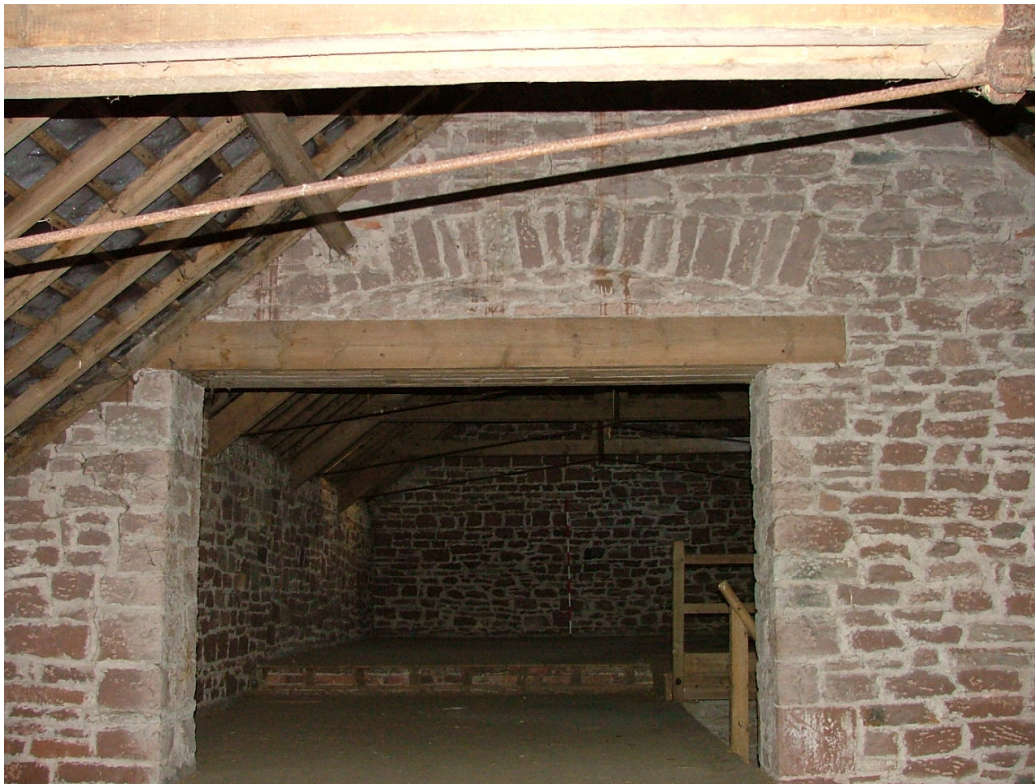
Plate 16 – Masonry gable wall, first floor of Building A showing arched stonework
