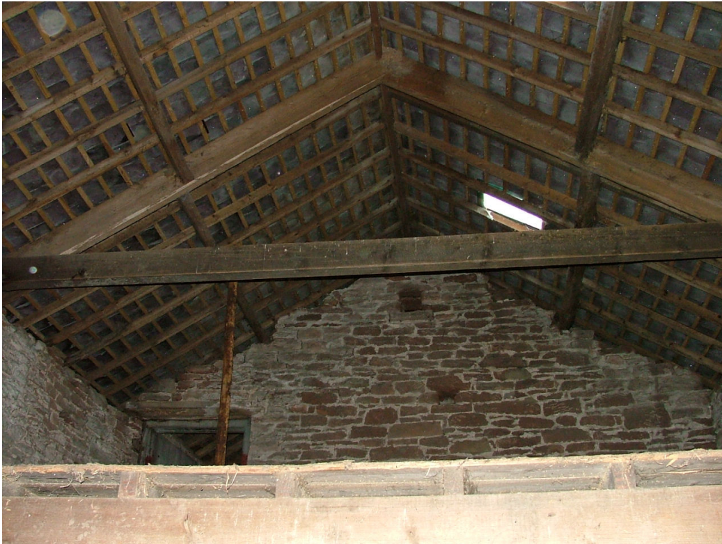
Plate 22 – Roof structure, Building B
