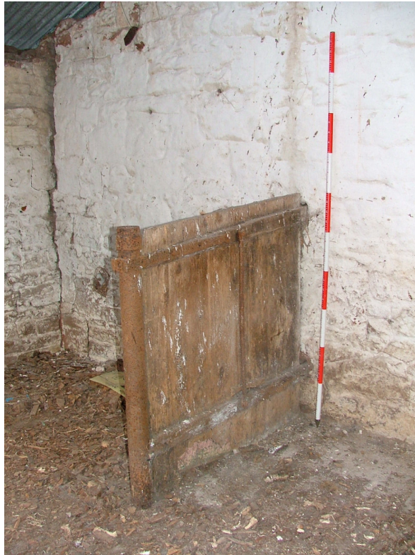
Plate 11 – Timber stall divider, lean-to at west end of range (Building A)
