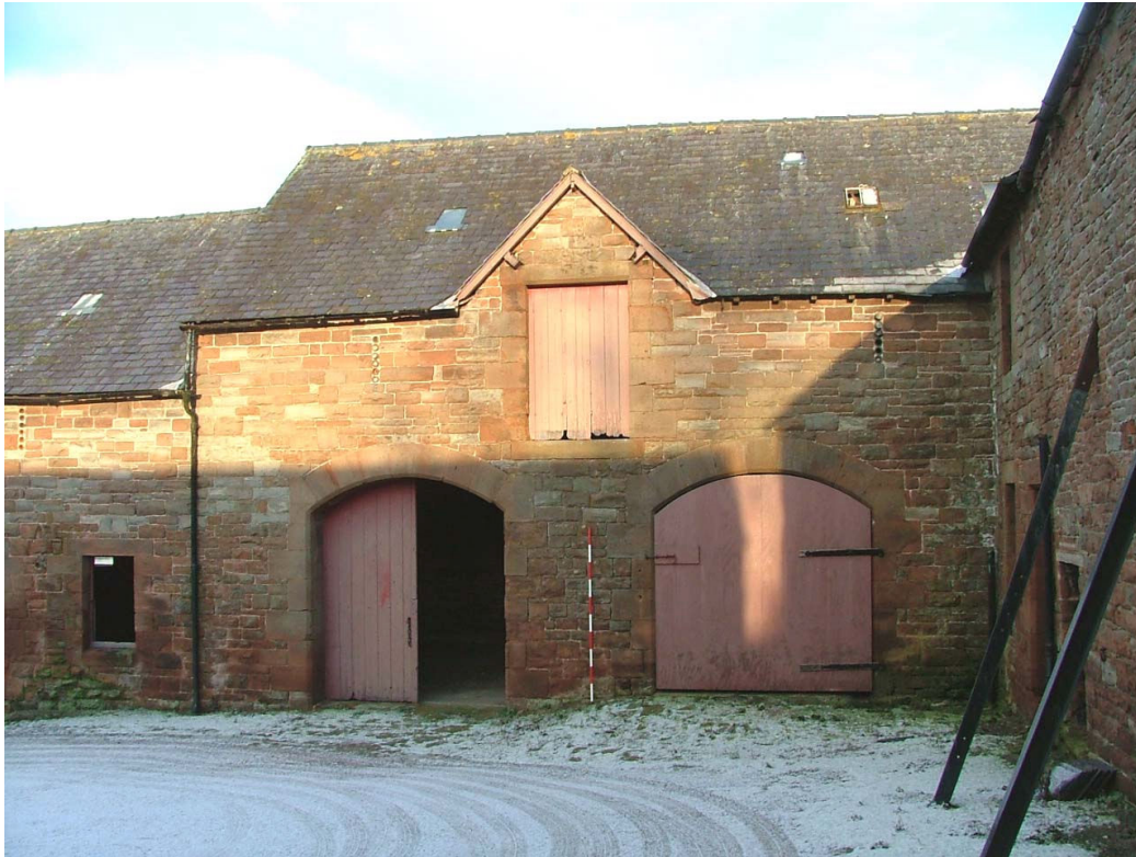
Plate 4 – Southern elevation of Building A, cart doorways
