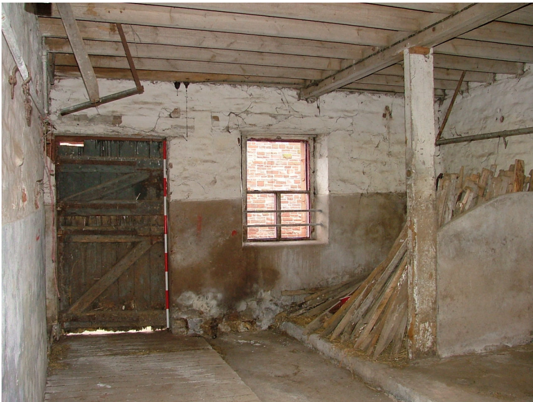
Plate 12 – Interior of byre
