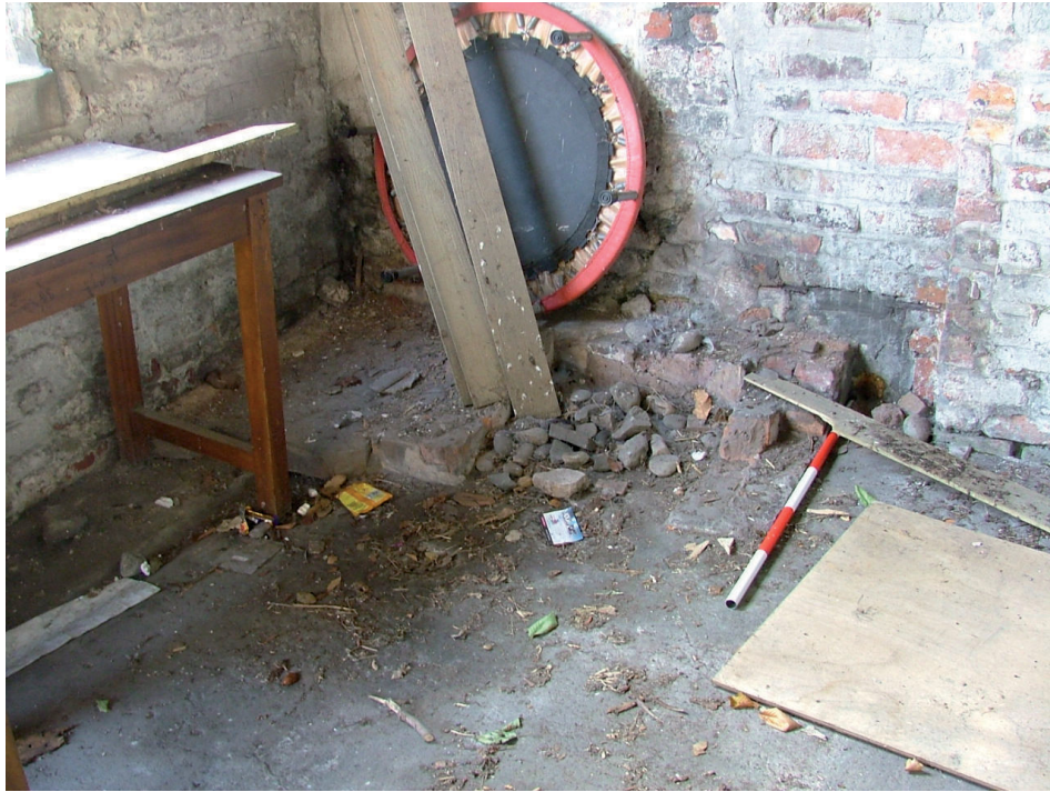
Plate 12 – Remains of brick-built structure with small blocked aperture in wall
