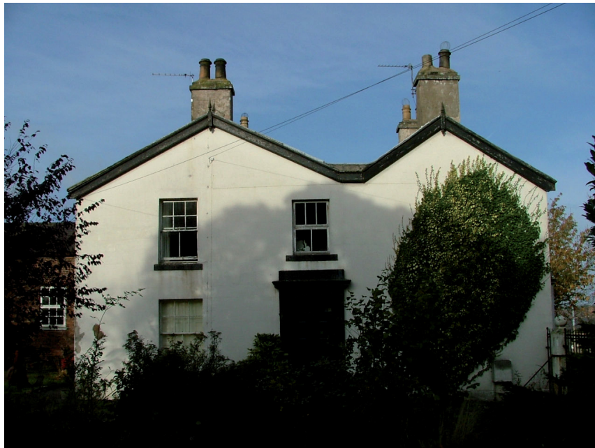
Plate 21 – East elevation of house
