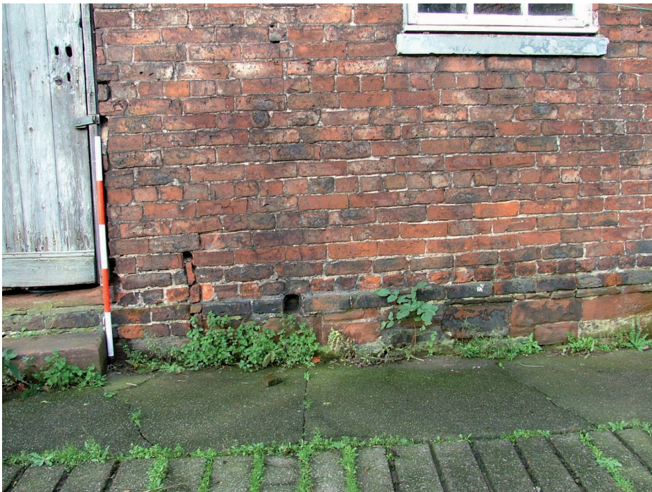
Plate 5 – Sandstone plinth, northern end of east elevation
