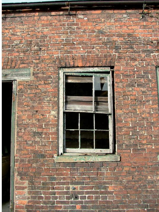
Plate 4 – Window in east elevation, possible original window frame?
