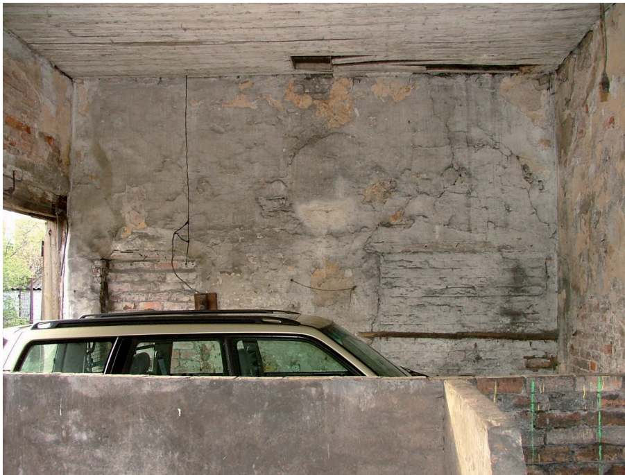
Plate 14 – Central interior wall (looking southwards) showing the two blocked doorways
