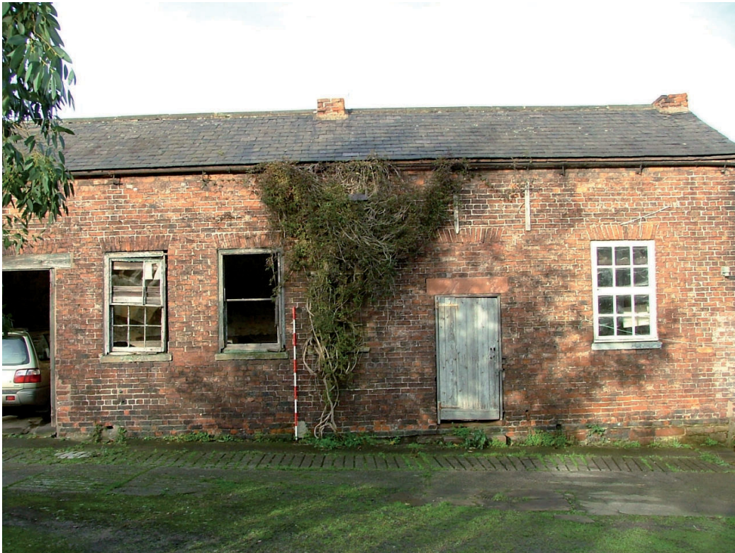
Plate 1 – Northern end of the east facing elevation
