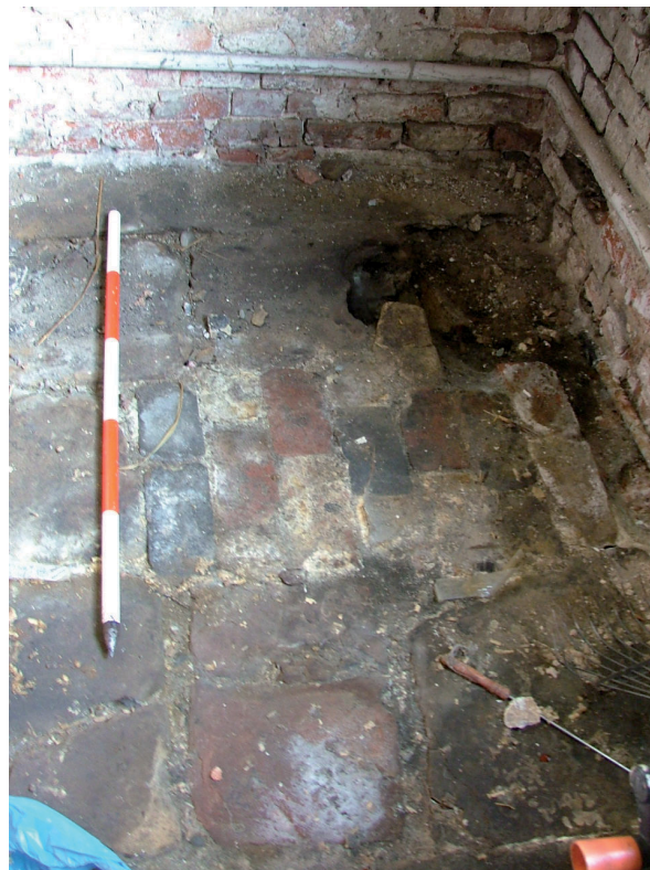
Plate 19 – Brick section of floor
