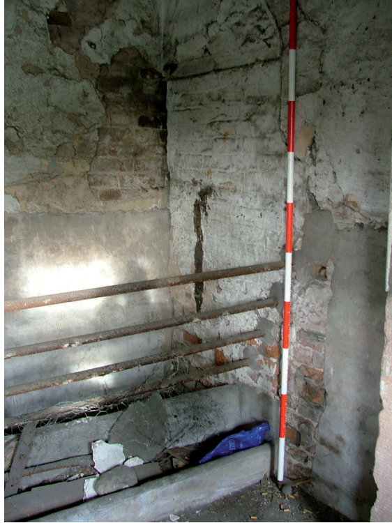
Plate 15 – Concrete feeding trough and blocked doorway
