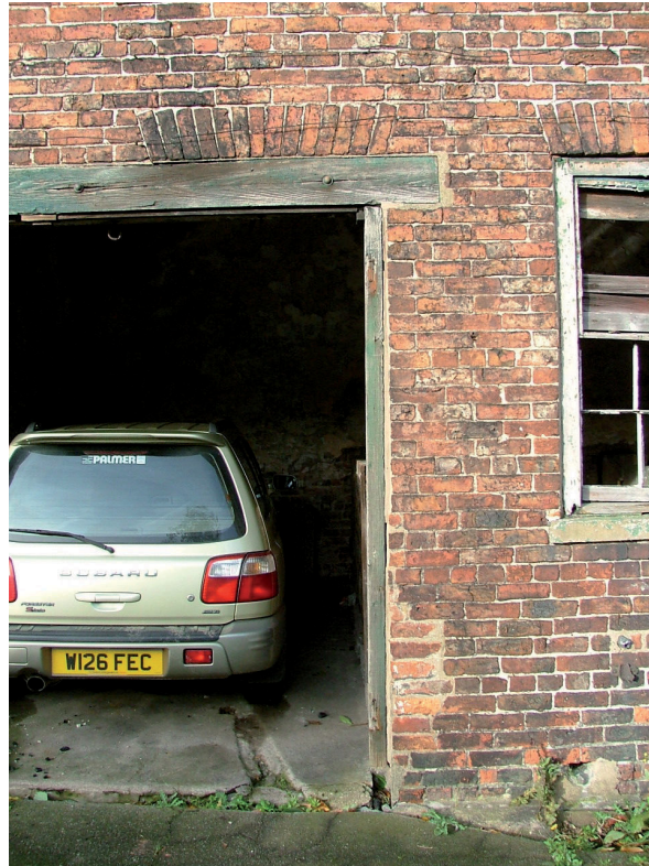
Plate 2 – Evidence for a former window, centre of east elevation
