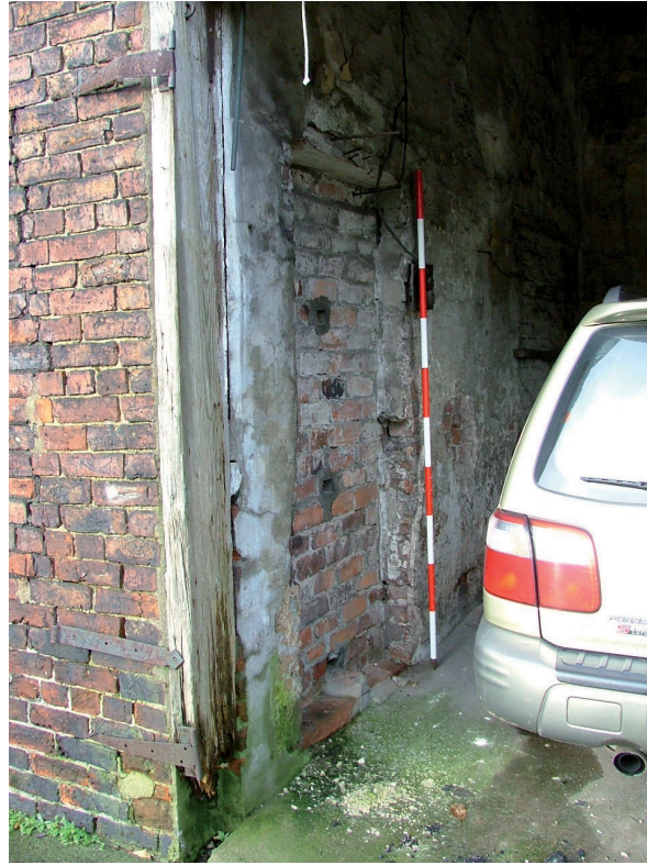
Plate 13 – Blocked doorway, central interior wall
