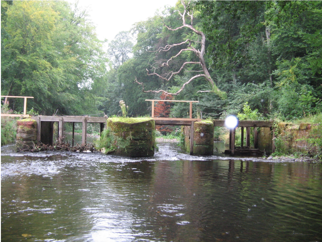
PLATE 11: THE SALMON COOPS, LOOKING NORTH
