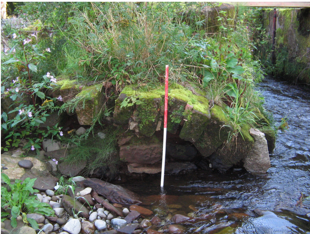
PLATE 10: ARCHED STONWORK AT NORTHERN EXTENT OF CAUSEWAY (AREA 2)
