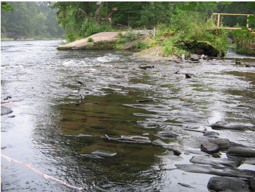
PLATE 12: WEIR AND CAUSEWAY (AREA 2), LOOKING NORTH
