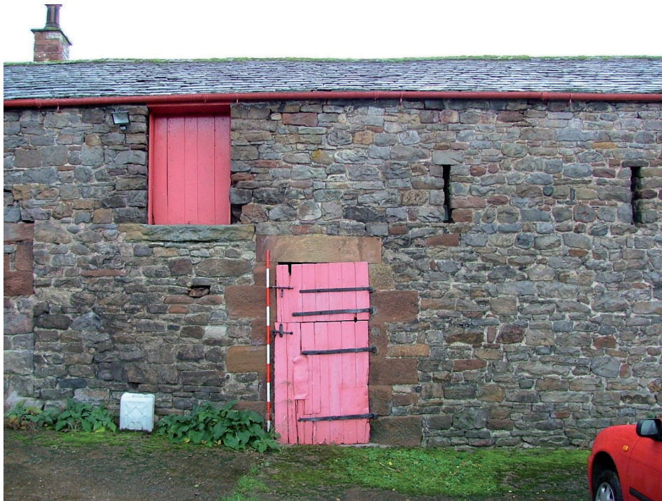
Plate 15 – North elevation of Range B (Building 3)
