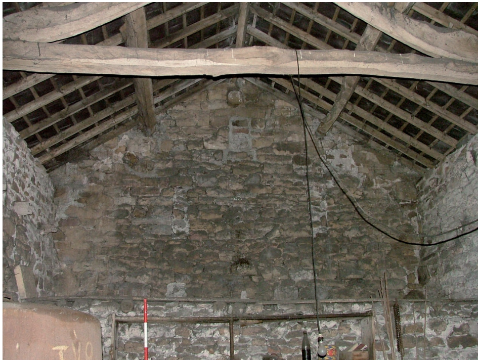
Plate 8 – Interior of Building 1, south elevation
