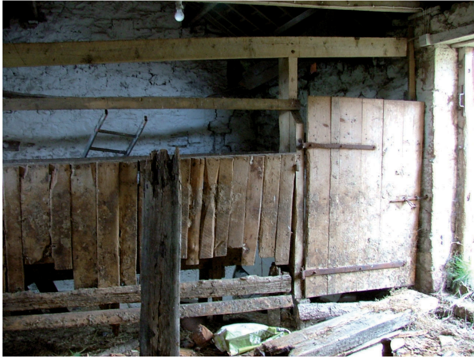
Plate 29 – Timber partition in Building 5 with hay rack and door
