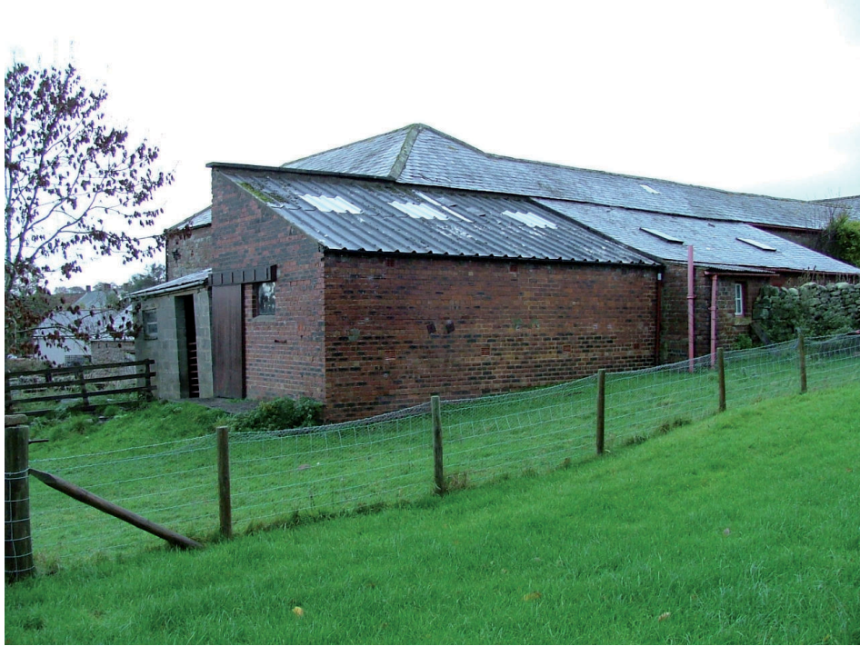
Plate 30 – South elevation of Building 6
