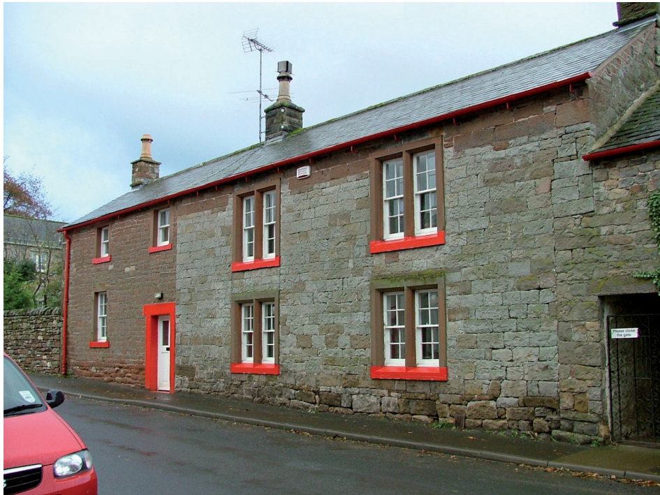
Plate 34 – East elevation of the farmhouse
