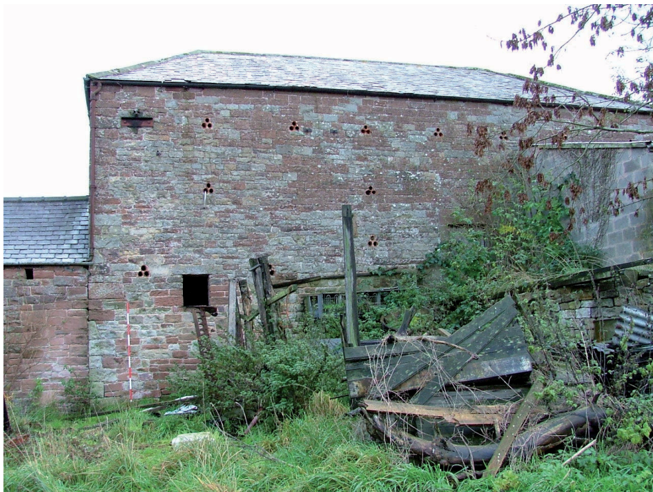
Plate 20 – West elevation of Building 4, masonry wall to the right of photograph retains a ramp (on which Building 7 has been constructed) which may have allowed for the transference of hay into the building from a cart
