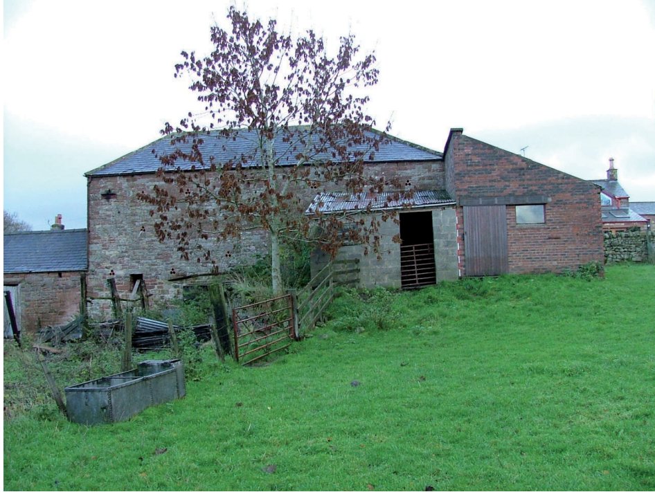
Plate 33 – Western elevations of Buildings 4, 7 and 6
