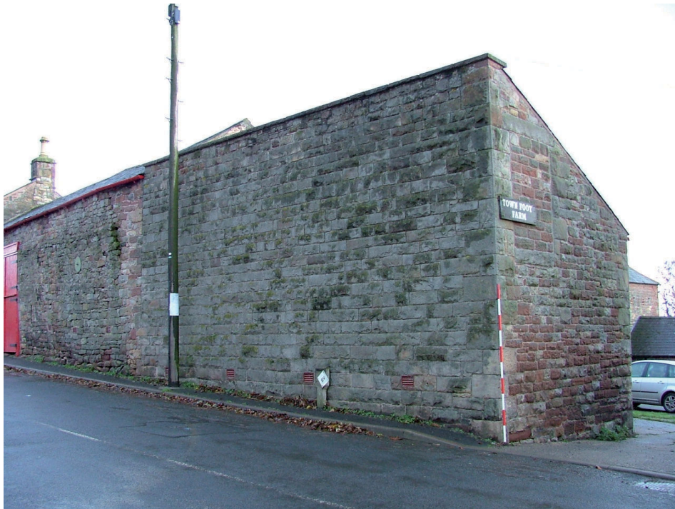
Plate 5 – North and east elevations of Building 2
