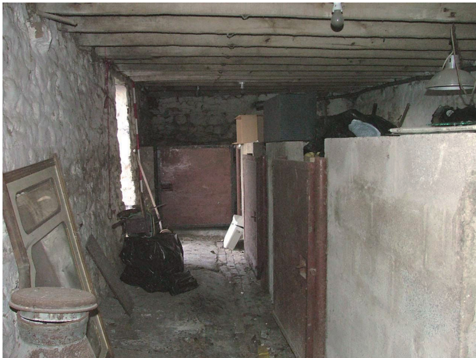
Plate 17 – Interior of Building 3, view looking east showing block work pig sties with iron gates
