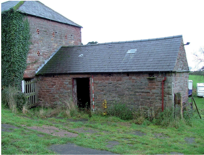
Plate 21 – East elevation of Building 5
