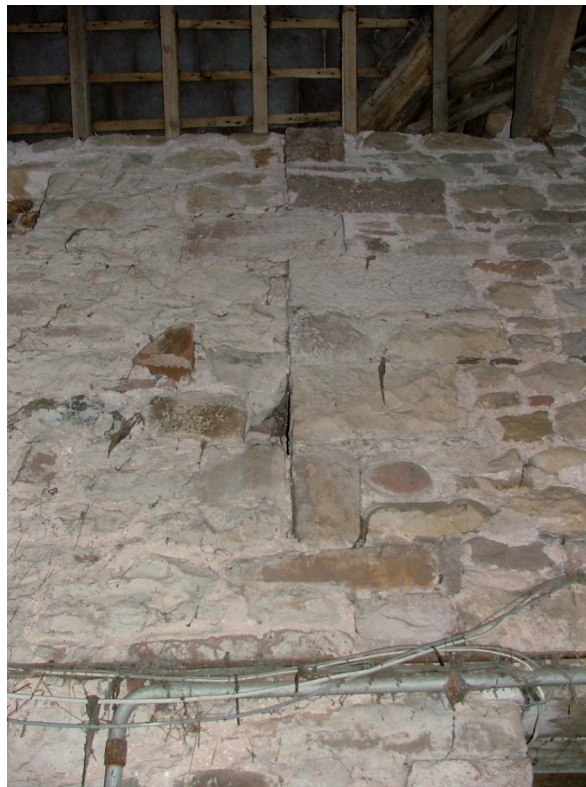
Plate 28 – Quoins of western gable end of Building 3 with the east wall of Building 4 to the left
