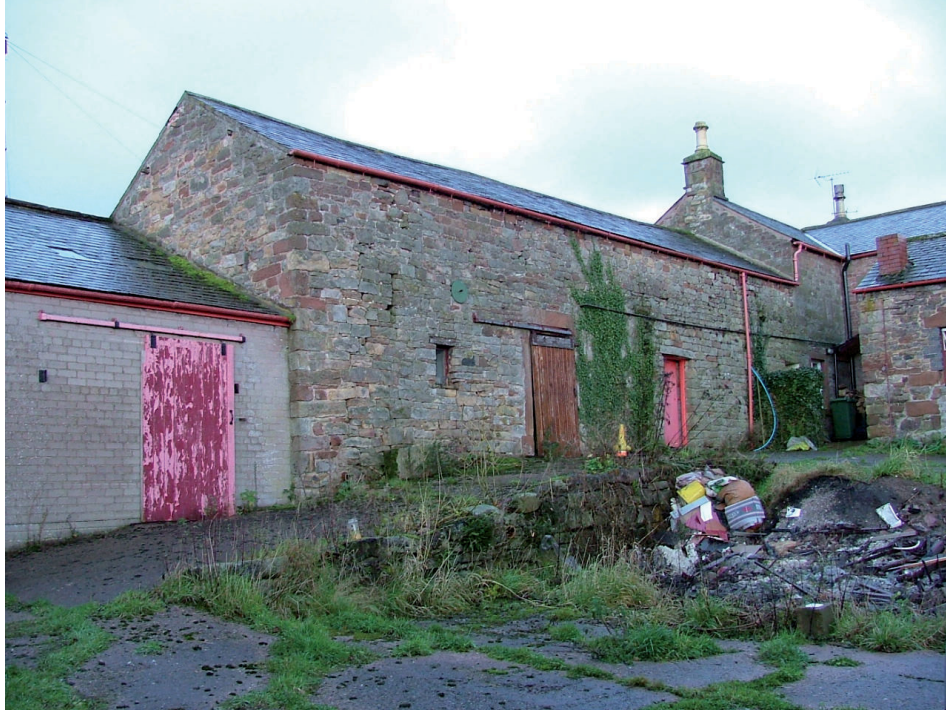
Plate 6 – West elevation of Building 1
