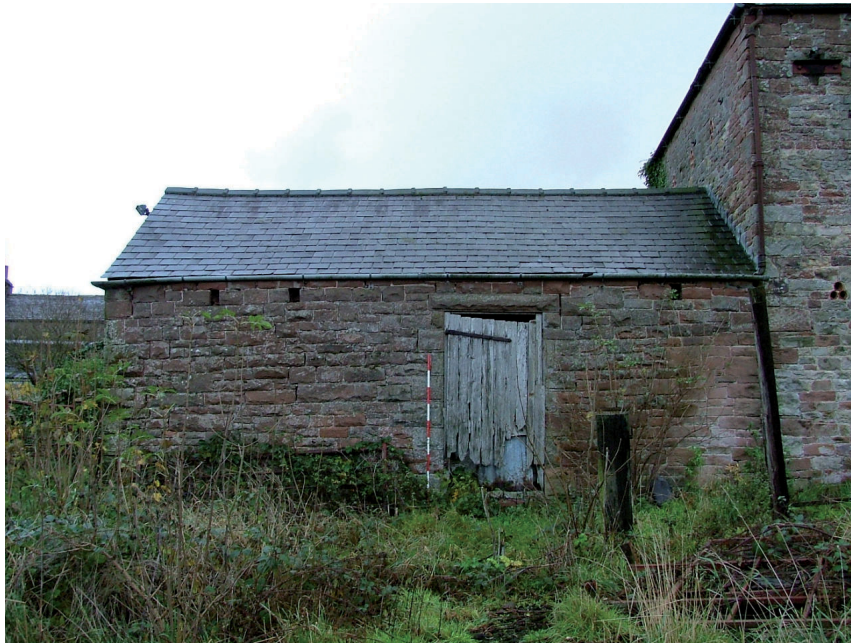
Plate 22 – West elevation of Building 5
