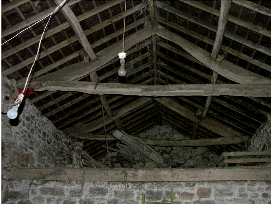
Plate 9 – Detail of roof structure, Building 1
