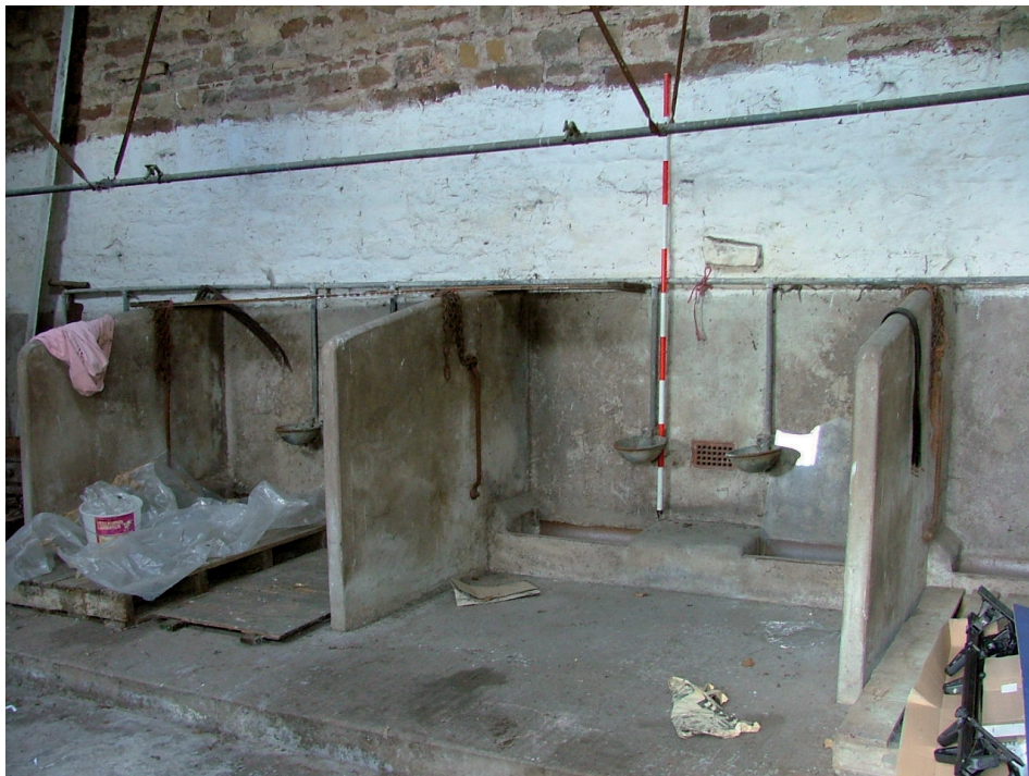
Plate 13 – Interior of Building 2 showing stall divisions, troughs and tethering bars
