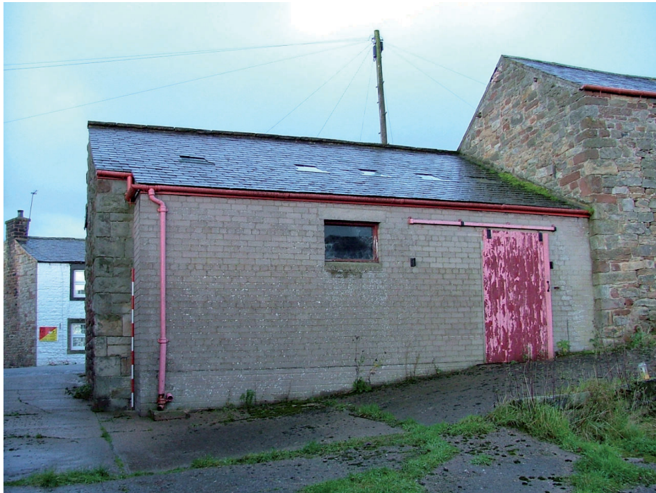
Plate 7 – West elevation of Building 2
