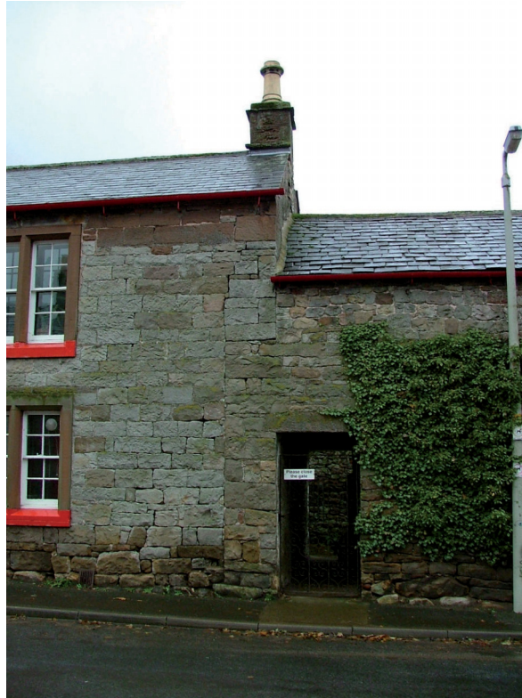
Plate 35 – Construction break between farmhouse and Building 1
