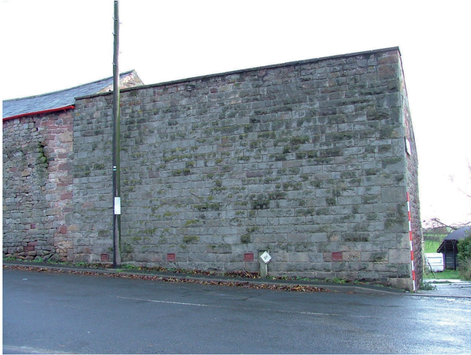
Plate 4 – East elevation of Building 2, Range A
