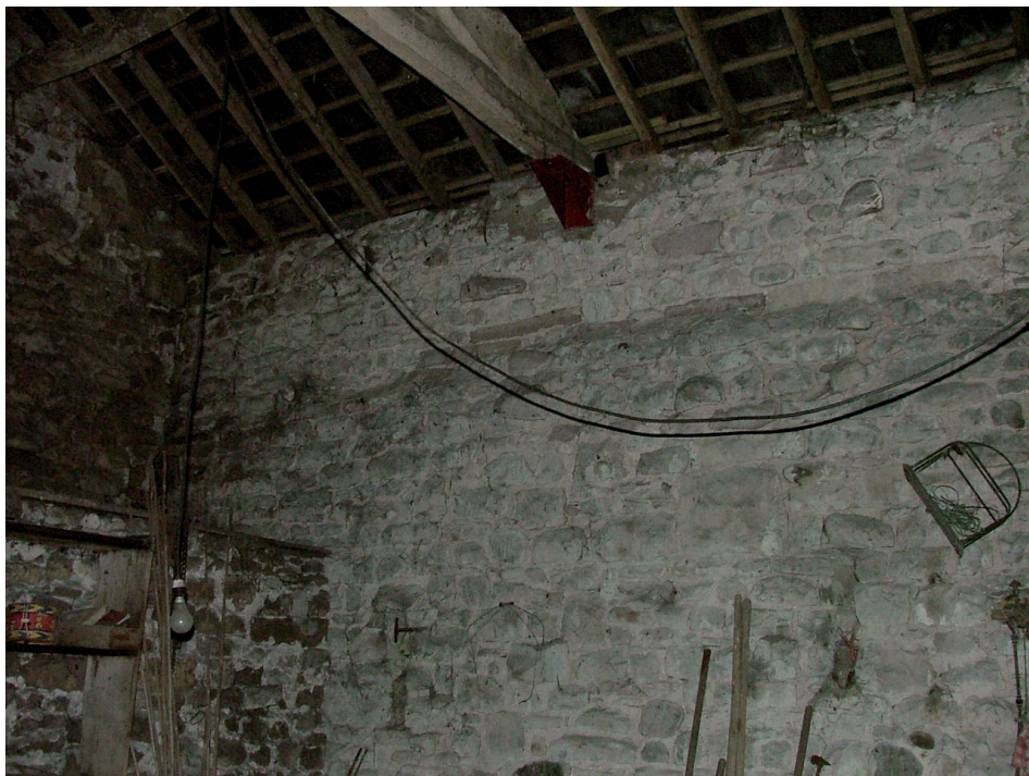
Plate 10 – Interior of Building 1 showing change in masonry (west wall)
