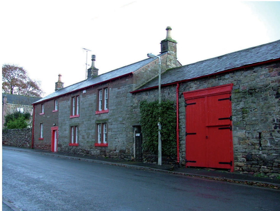
Plate 1 – Townfoot Farm, east facing elevation of farmhouse and part of barn
