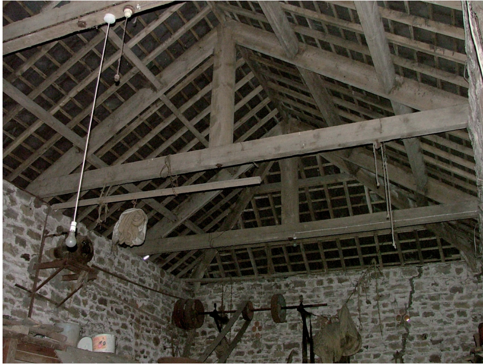
Plate 23 – Roof structure, Building 4
