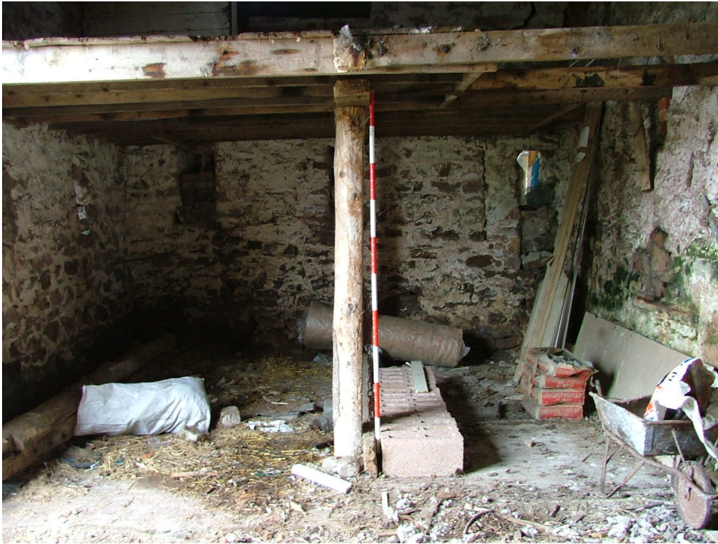
Plate 7 – Timber platform, eastern side of barn
