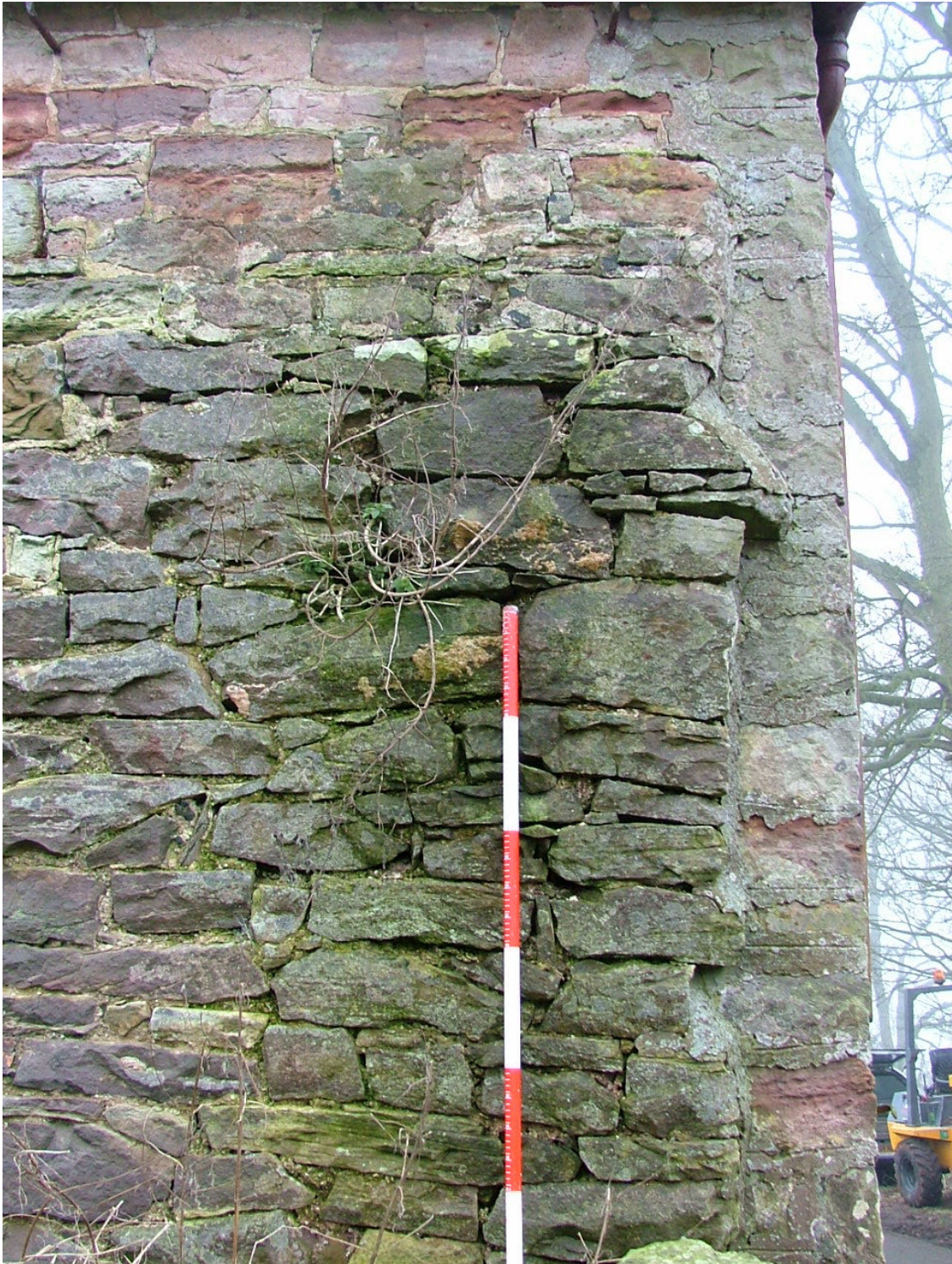
Plate 3 – West end of northern elevation showing change in masonry
