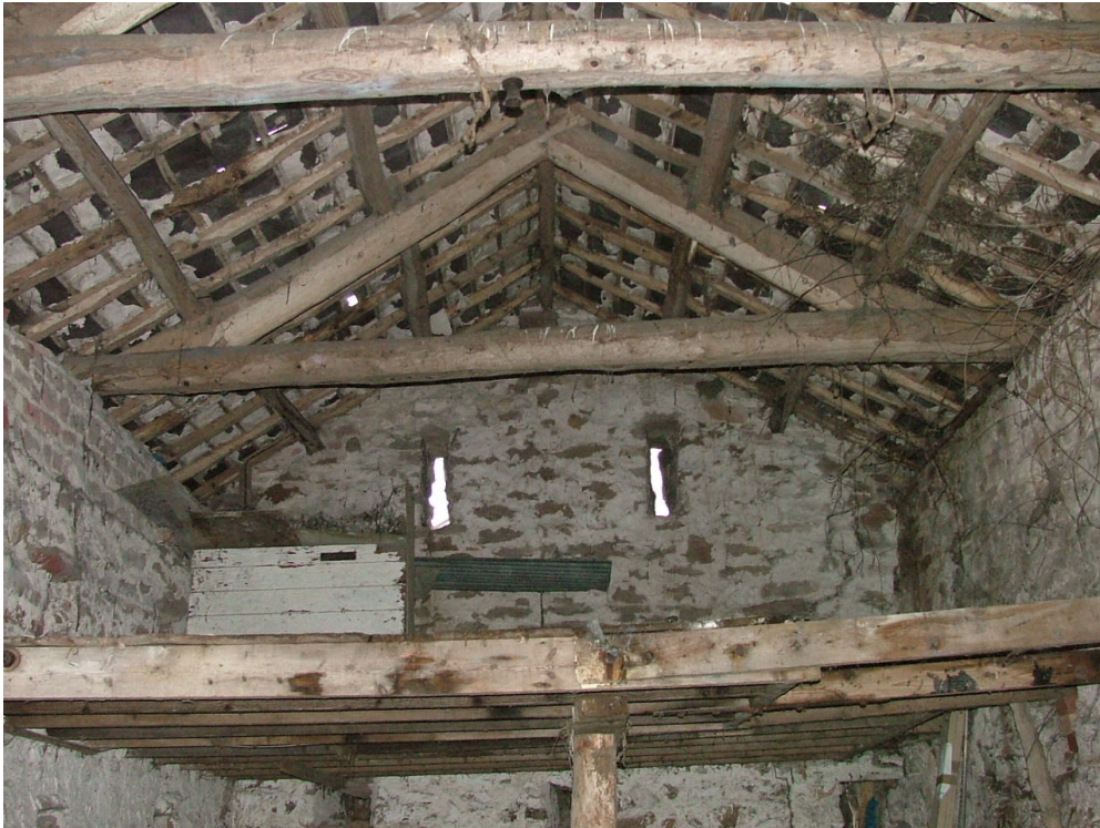
Plate 6 – Interior of the barn looking east
