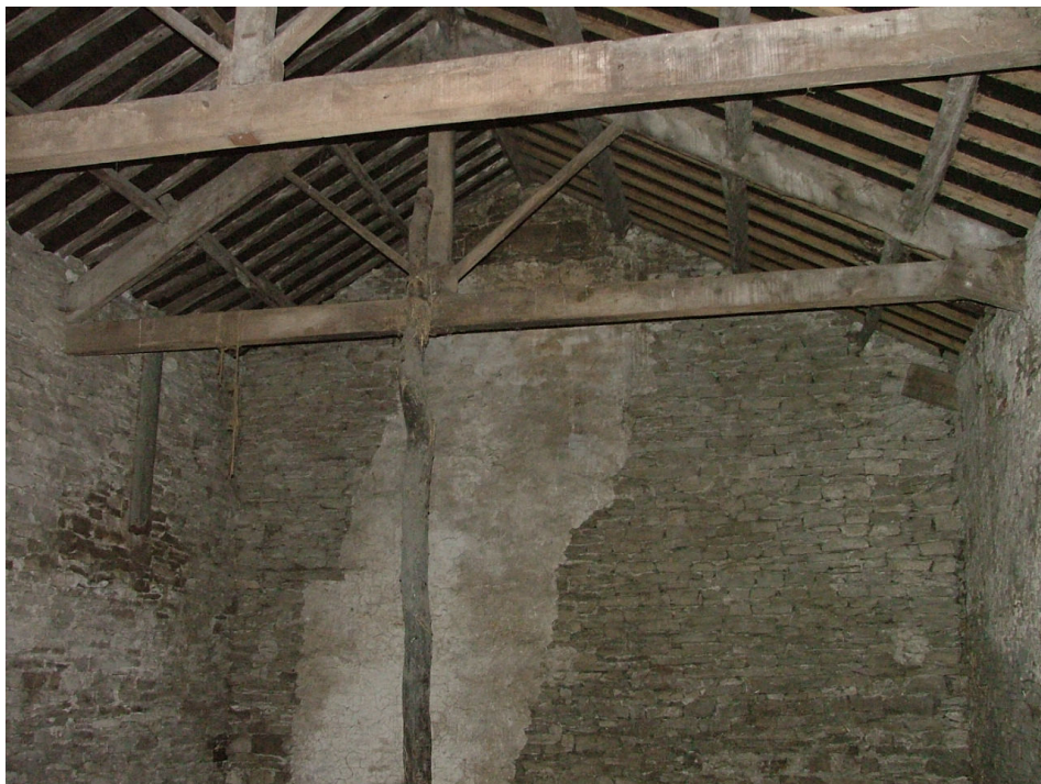
Plate 13 – Vertical tree trunk and plastered section of wall, interior of barn
