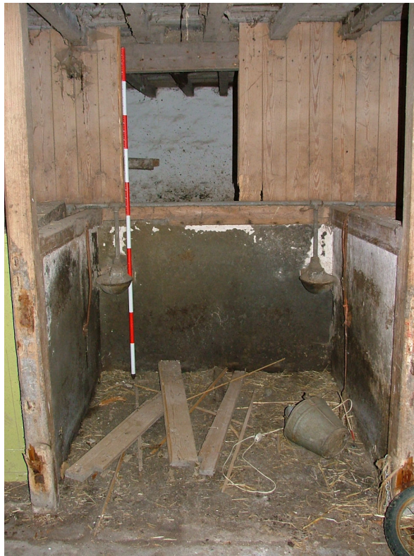
Plate 9 – Stall, showing stone scale boards and metal water troughs
