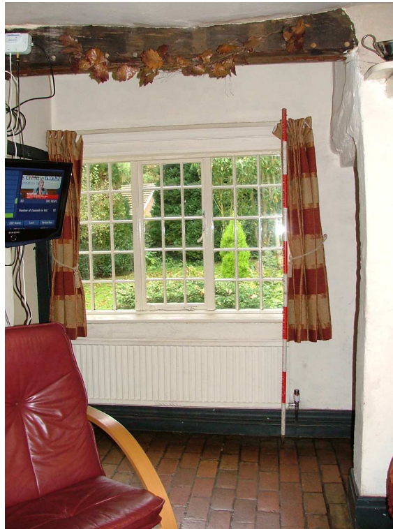
Plate 24 – Internal view of lean-to against west elevation (Scale = 2m)
