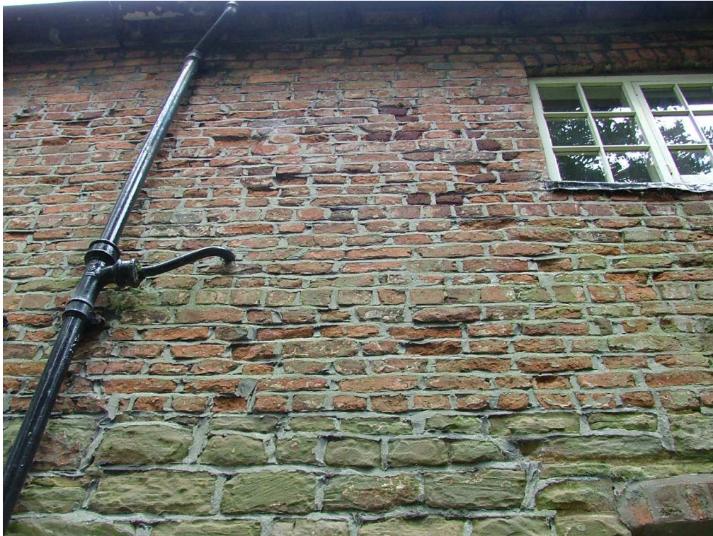
Plate 8 – Detail of the masonry and brickwork, south elevation of cross-wing
