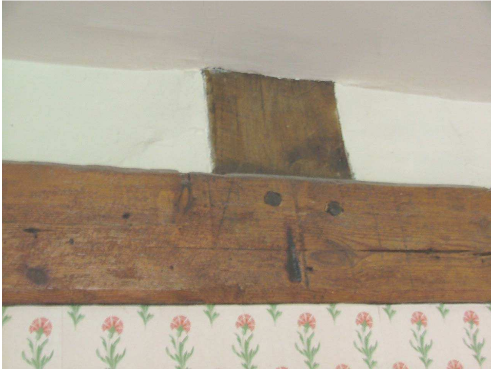
Plate 38 – Base of king-post roof truss in north bedroom showing chamfered edges of tie-beam, peg holes and possible burning from a candle
