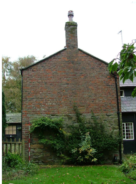
Plate 15 – West elevation of north-west extension (Scale = 2m)
