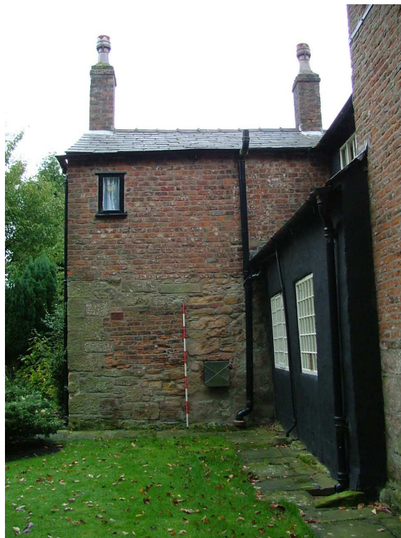
Plate 13 – South elevation of north-west extension showing blocked window at ground floor level (Scale = 2m)
