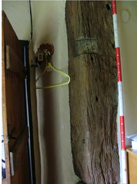
Plate 26 – Vertical timber with carved notch in office, ground floor
