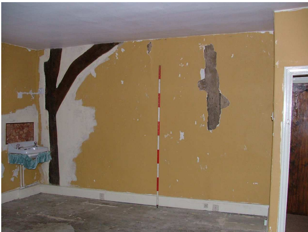
Plate 35 – Wall dividing the two bedrooms in the cross-wing (Scale = 2m)
