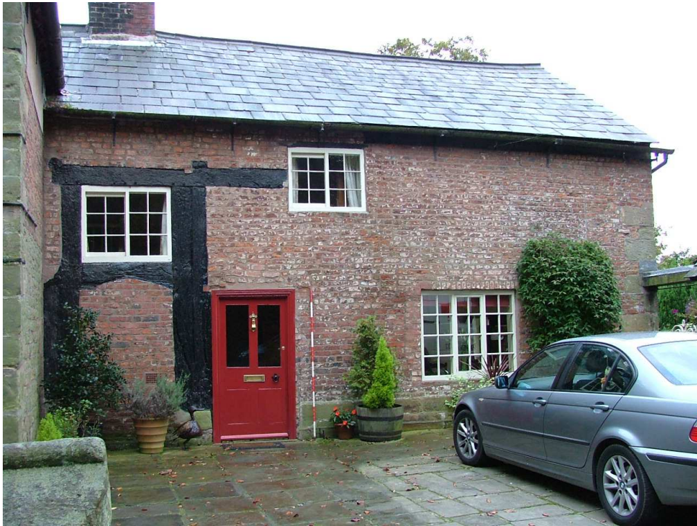
Plate 2 – East elevation of main range of house (Scale = 2m)
