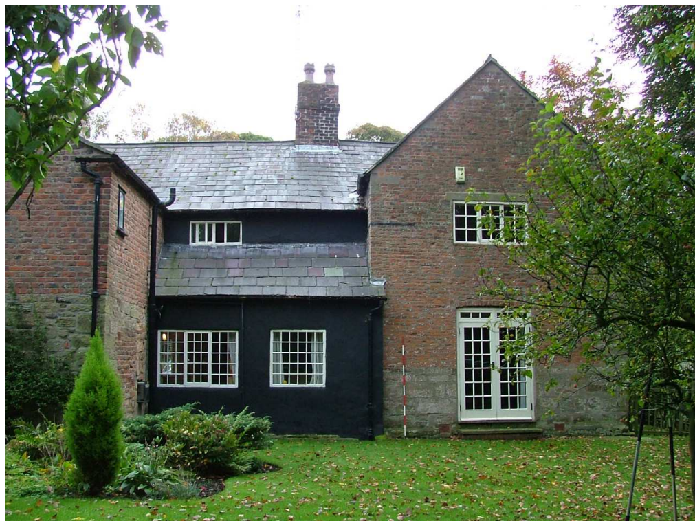
Plate 11 – West elevation showing the single-storey lean-to (Scale = 2m)
