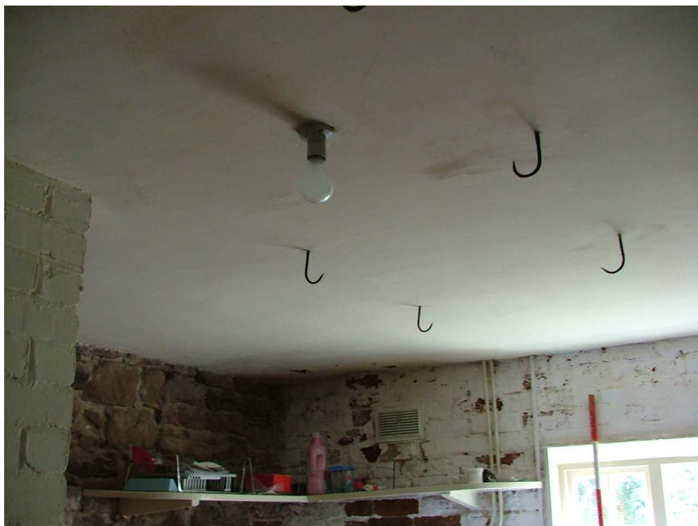
Plate 27 – Ceiling of former dairy or pantry, ground floor of north-west extension
