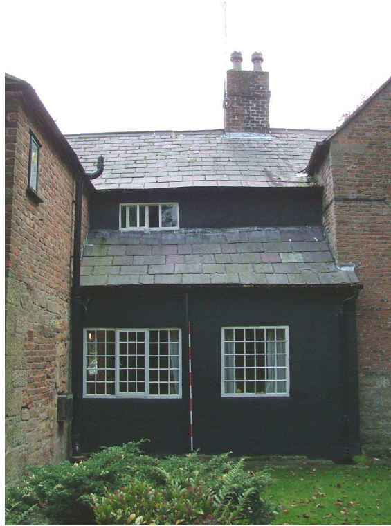
Plate 12 – Single-storey lean-to, west elevation (Scale = 2m)
