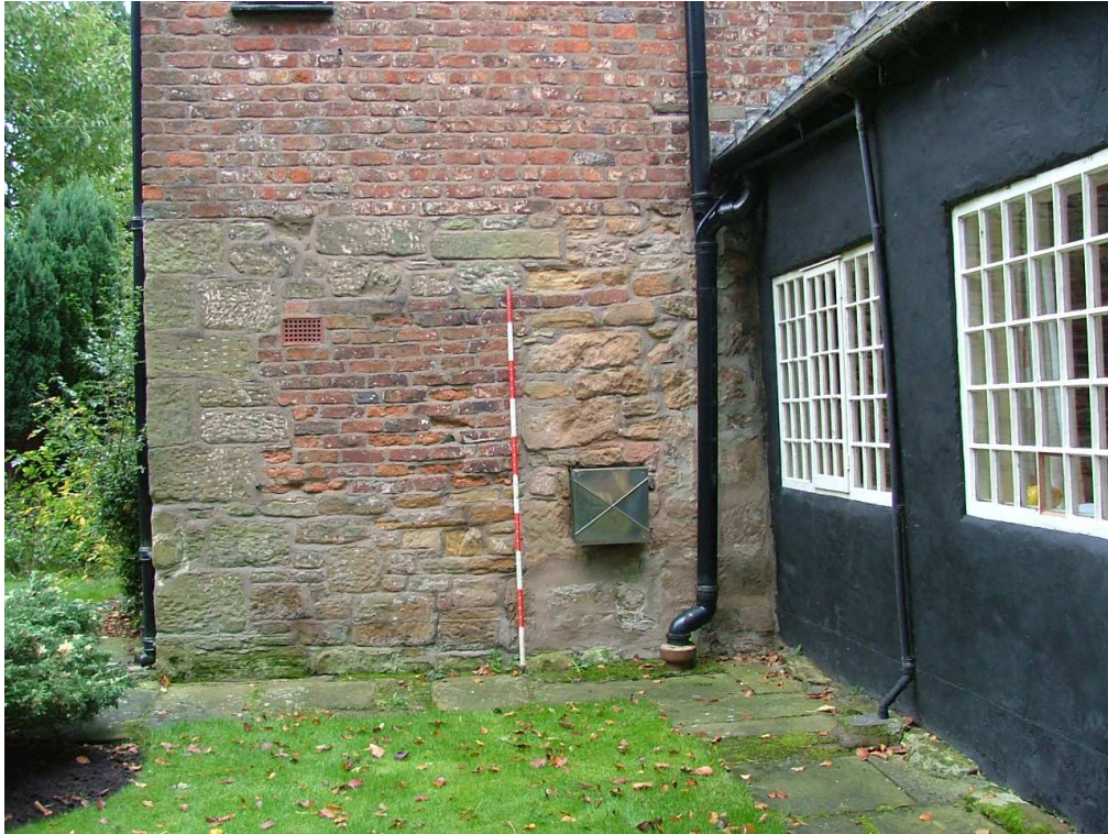
Plate 14 – Detail of blocked window, south elevation of north-west extension (Scale = 2m)
