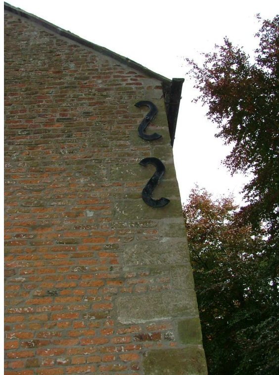
Plate 10 – Detail of the two backward S-shaped tie-plates, west elevation of cross-wing
