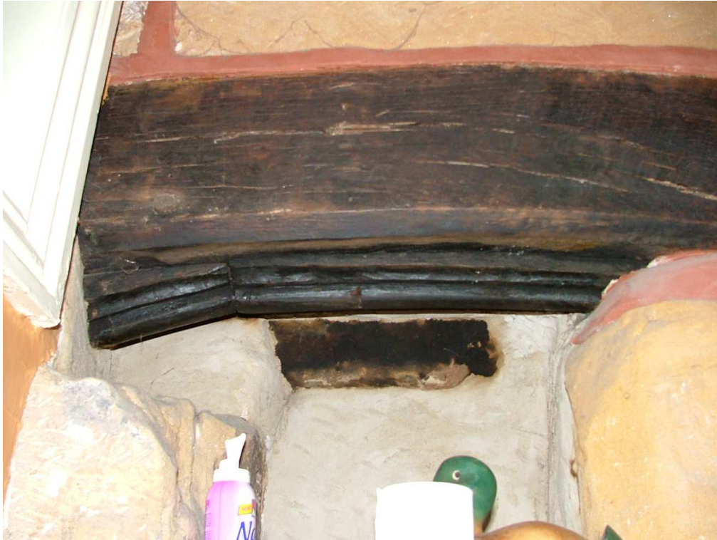
Plate 32 – Detail of decorative moulding on possible ‘spere truss’
