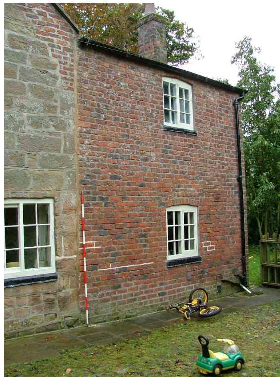
Plate 17 – North elevation of north-west extension (Scale = 2m)
