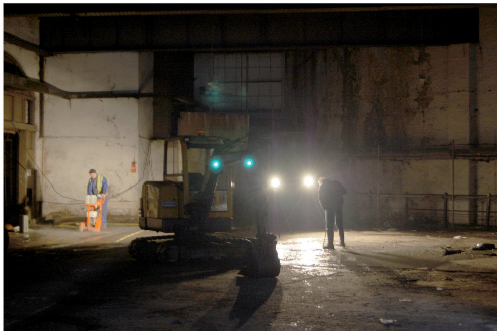
Plate 2: Cutting Trenches 1 and 3
