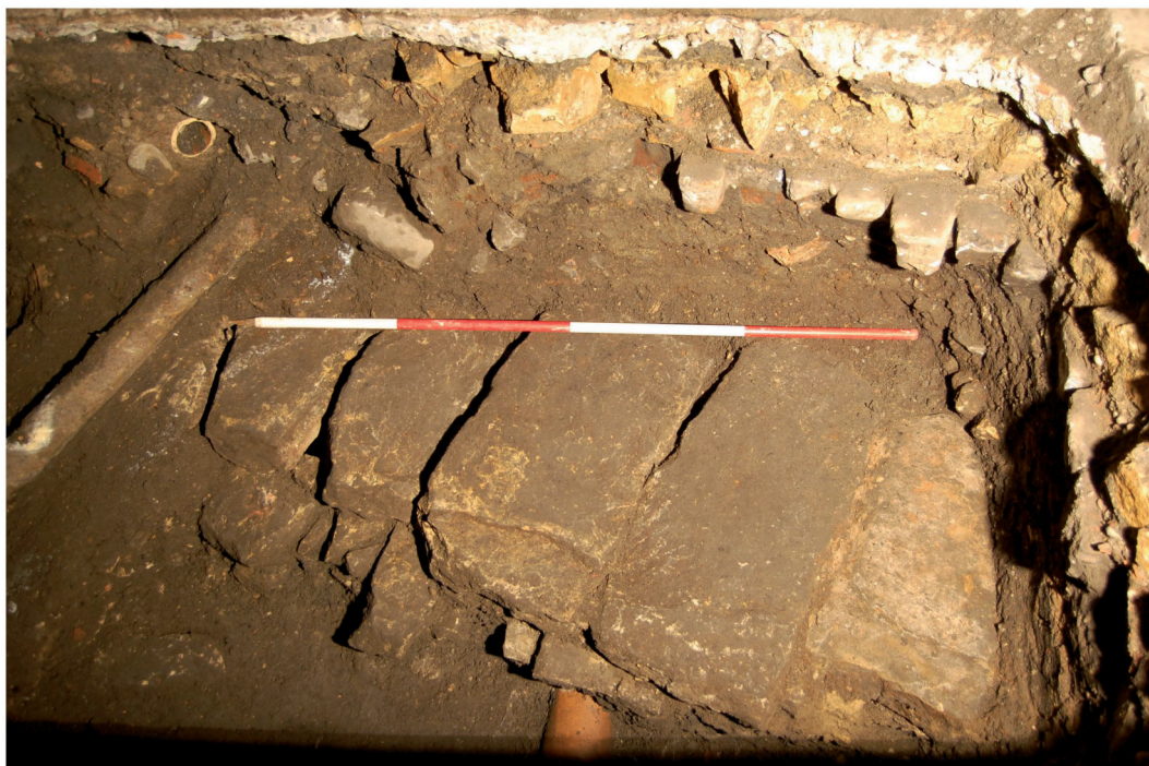
Plate 8: culvert [131], facing south, with setts [124] visible in section.
