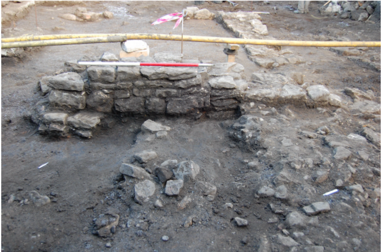
Plate 11. View of the area in the foreground with wall (116) central indicating the edge of Buildings #4/#5.
