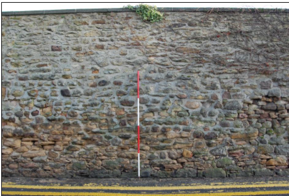
Plate 12. External face of bounding wall before demolition.
