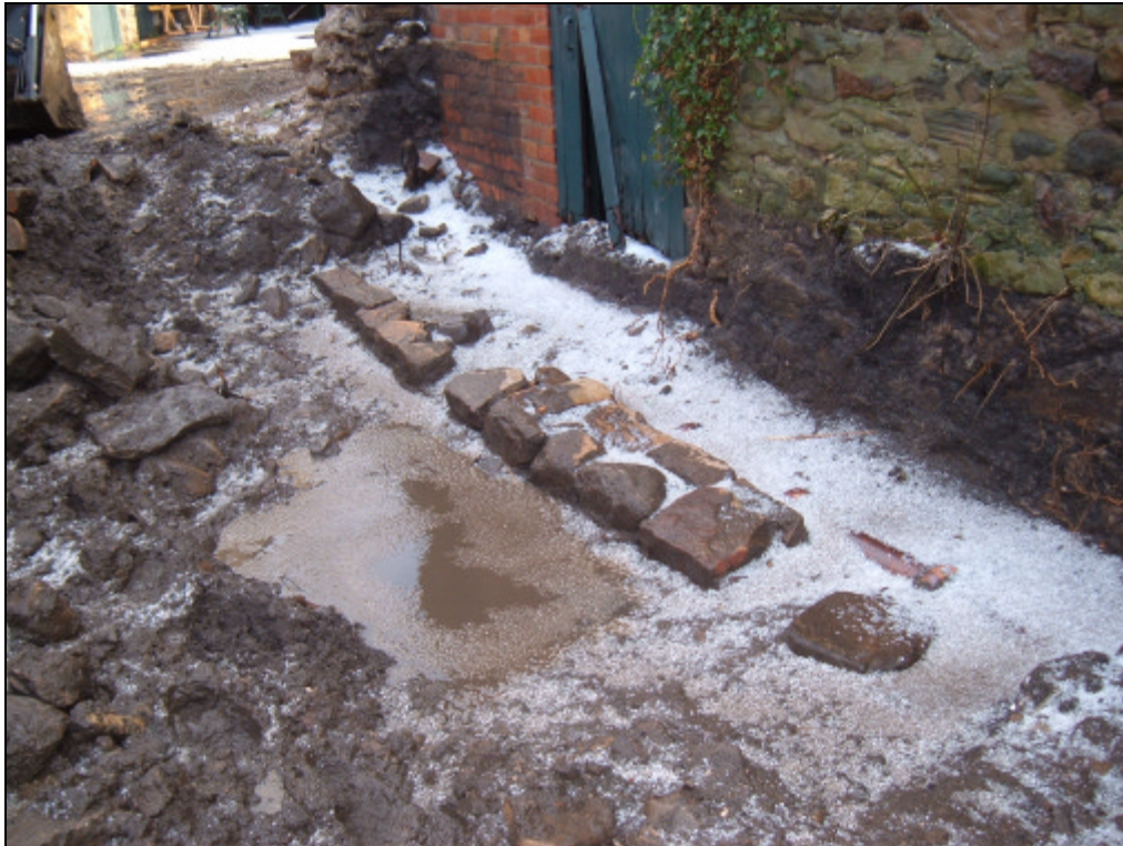
Plate 3. Building #1 (103/104) looking north-east during the watching brief.
