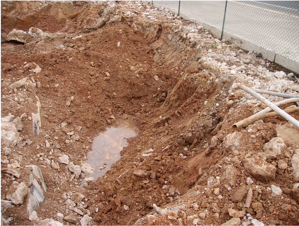
Plate 3: Spilled Fluid in Fuel Tank Pit
