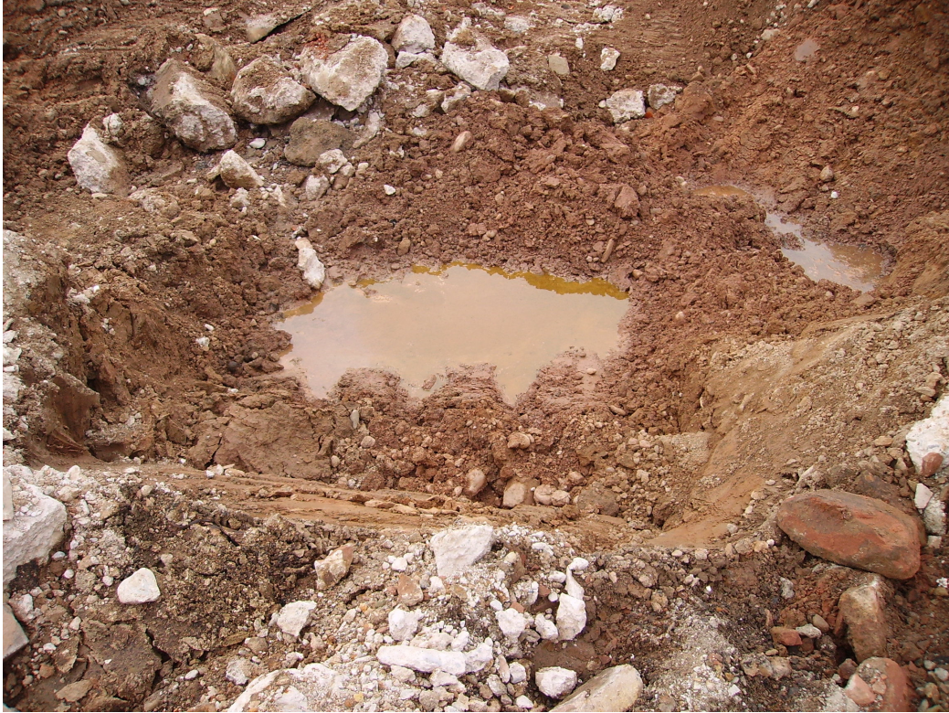
Plate 3. Spilled Fluid in Fuel Tank Pit
