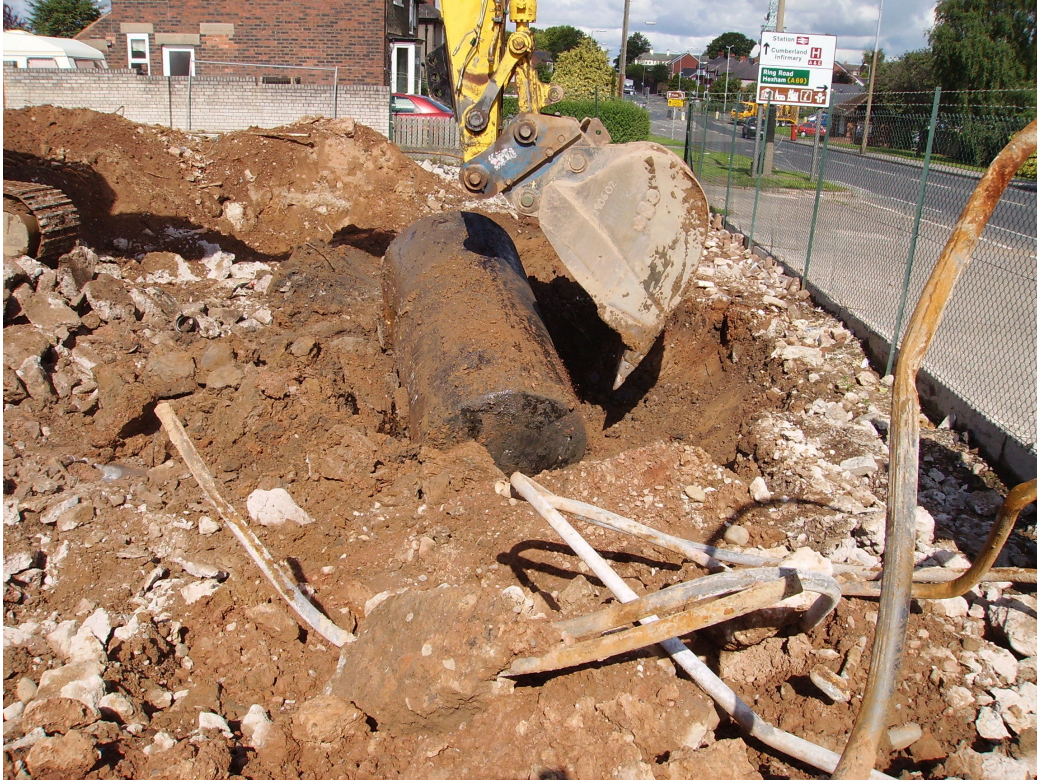
Plate 2. Removal of a Fuel Tank by Mechanical Excavator
