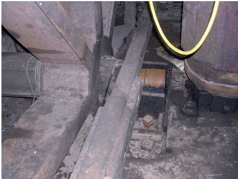
Plate 19: Detail of pit wheel and mounting arrangement at Warwick Mill
