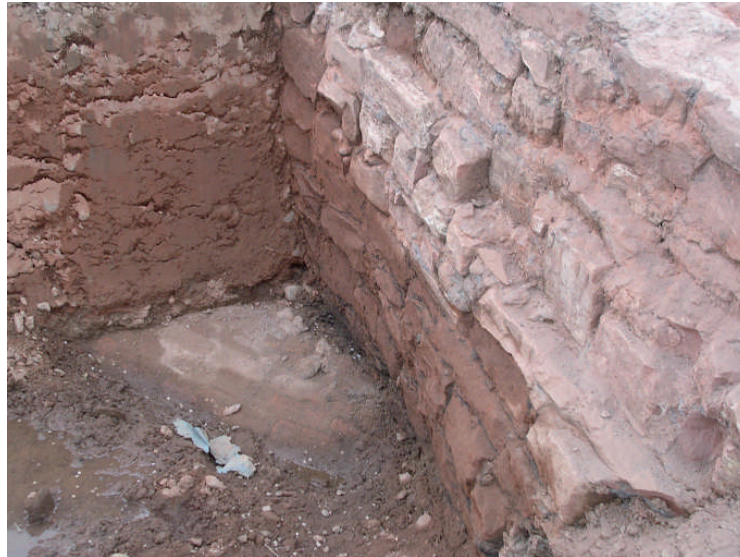
Plate 10: Wall 129 with top of arched culvert exposed at base of trench
