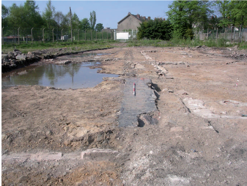
Plate 7: Foundation remains of the northern rolling mill extension
