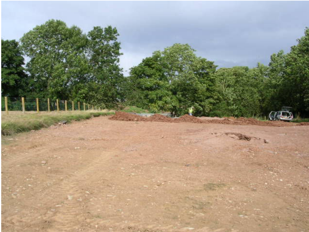
Plate 1: General site shot of stripped central area of site
