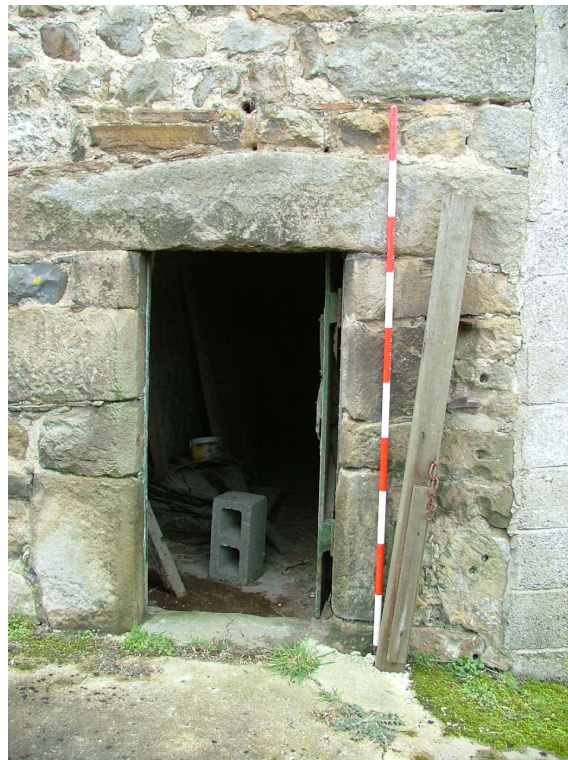
Plate 7 – Doorway to possible root store, NE elevation of Range A
