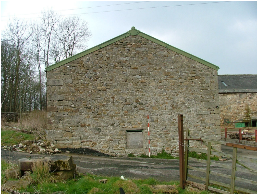
Plate 26 – South-east elevation of Range B
