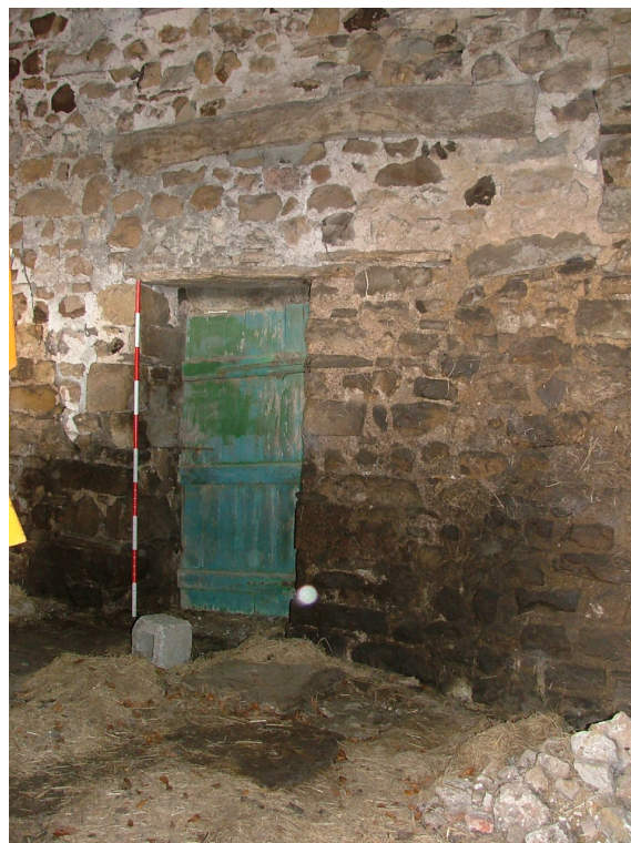
Plate 15 – Timber lintel of former cart doorway, north-west elevation of Range A
