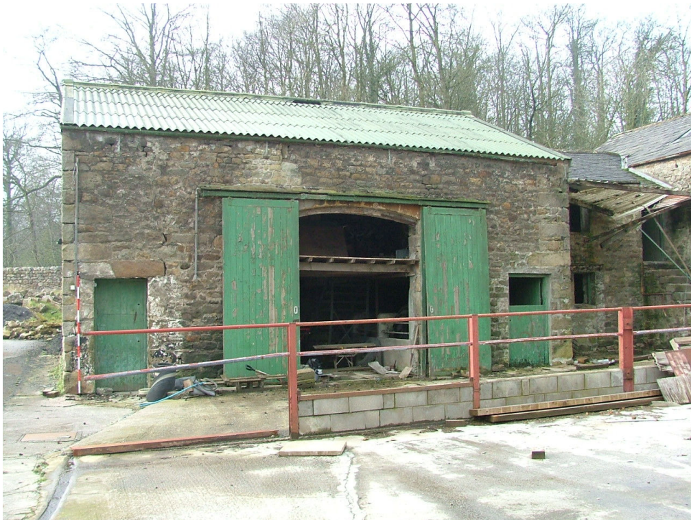
Plate 17 – North-east elevation of Range B
