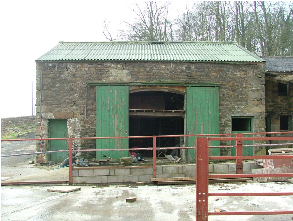
Plate 24 – North-east elevation of barn, Range B
