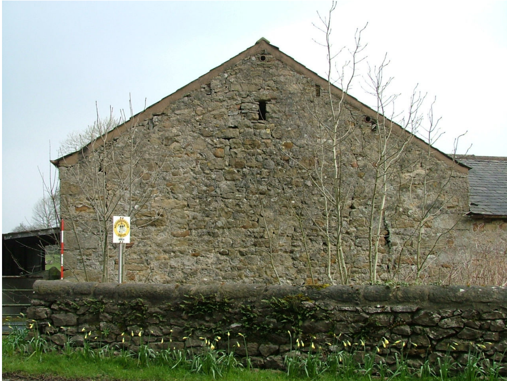
Plate 10 – South-west elevation of Range A as seen from the road
