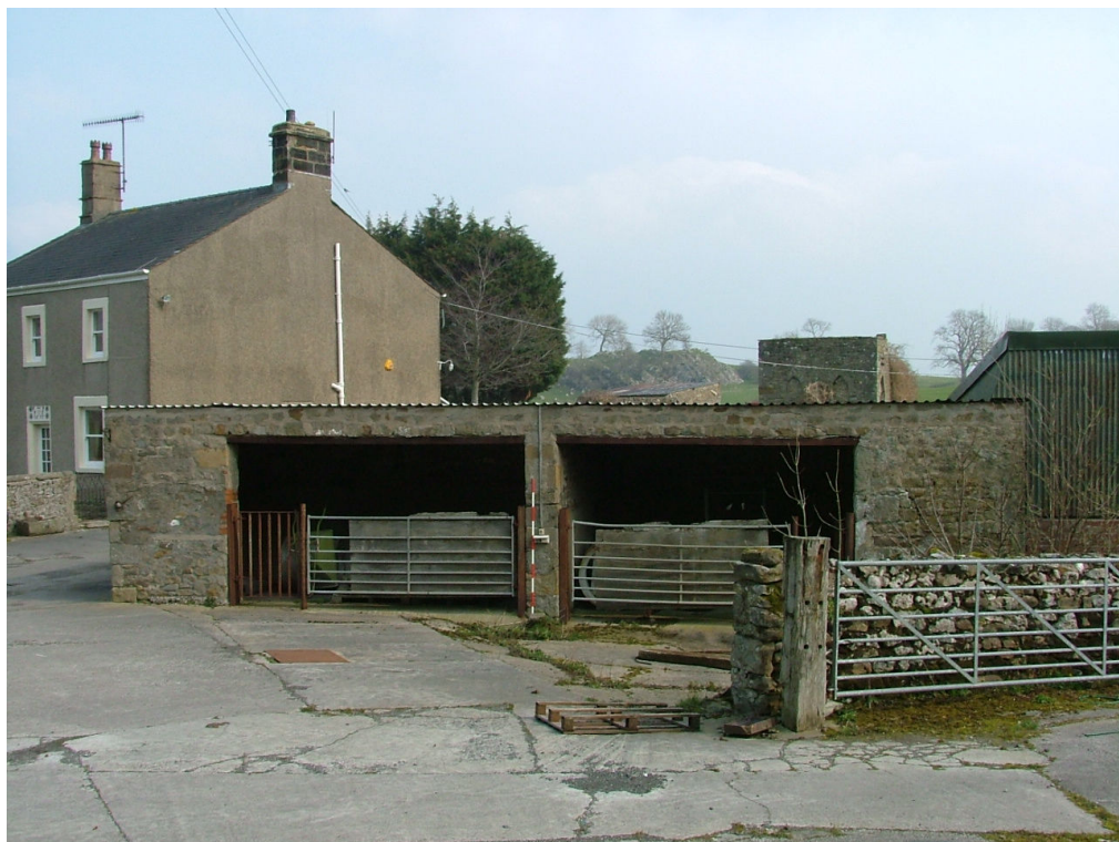
Plate 39 – Building to the south of the farmhouse (view looking east)
