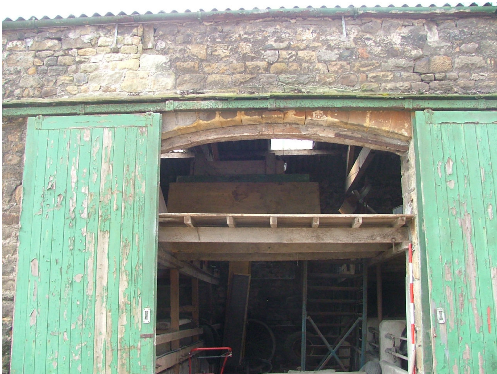
Plate 25 – Detail of arched doorway, north-east elevation of Range B
