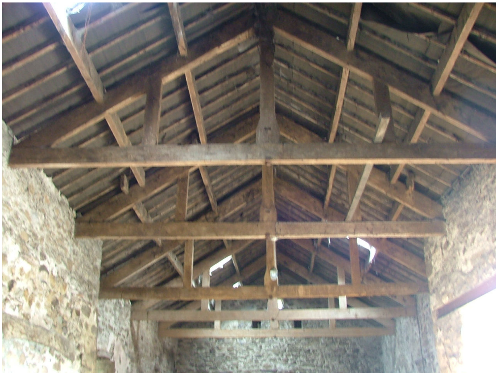
Plate 13 – Roof structure, Range A, looking northwards
