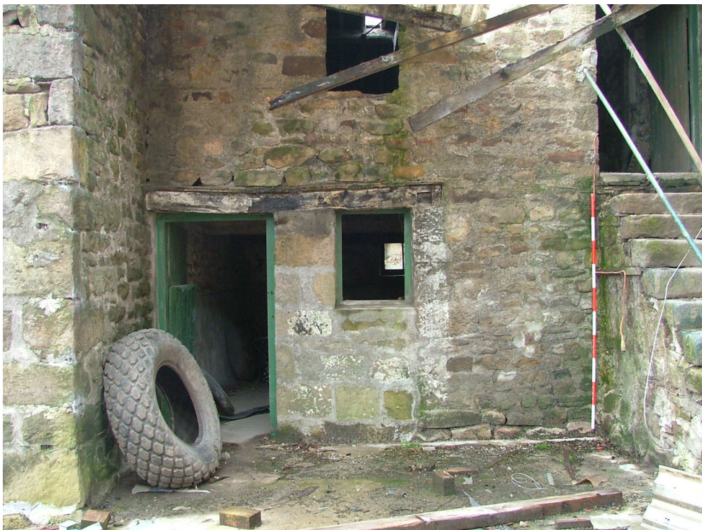
Plate 21 – North-east elevation of cowhouse/granary, Range B
