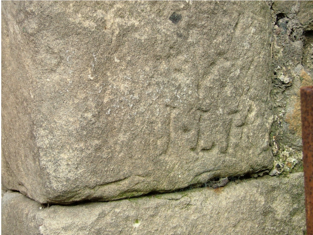
Plate 32 – Initials 'I L H', door jamb, south-east elevation of Range A
