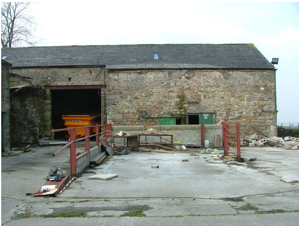
Plate 3 – South-east facing elevation of Range A
