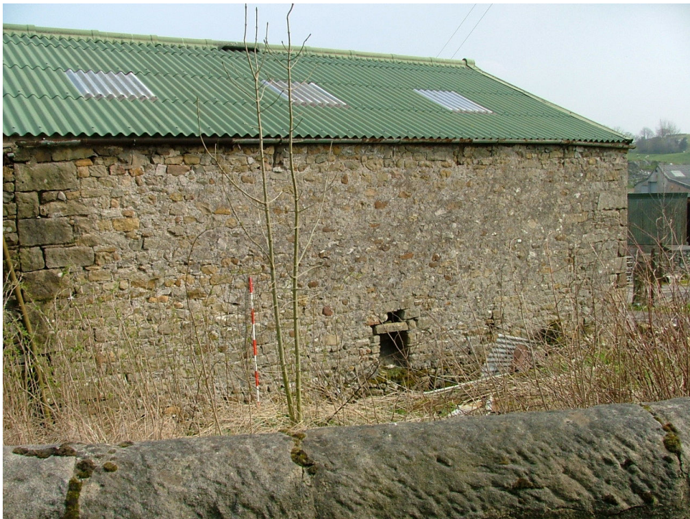
Plate 27 – South-west elevation of Range B, showing aperture mid-way along elevation
