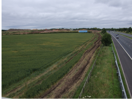
Plate 1: Site from South Facing East
