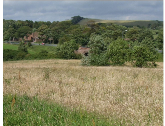
Plate 4: View of Jubilee Bridge from development site
