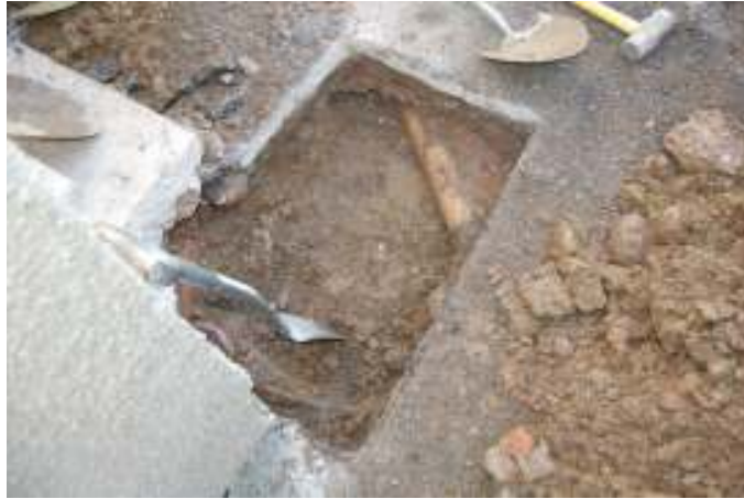
Plate 4: Trench 2, note shallow depth of the trench and the existing ceramic drain, facing north-east
