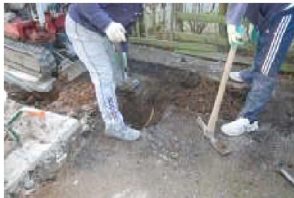
Plate 1: Hand excavation of Trench 1, note yellow gas pipe below tarmac surface
