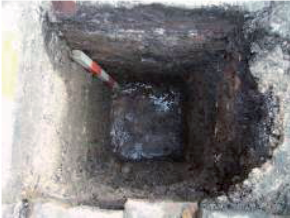
Plate 7: Showing (111) beneath the floor in Trench 1
