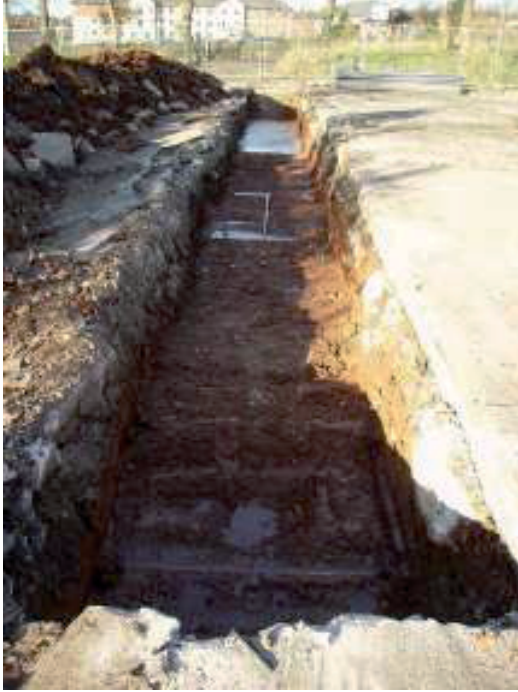
Plate 15: Looking West showing Trench 5.
