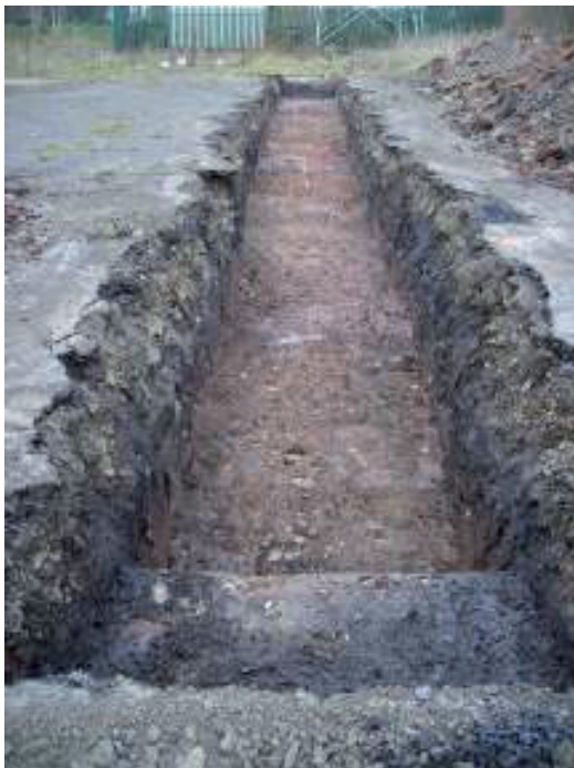
Plate 9: Looking North showing Trench 2.
