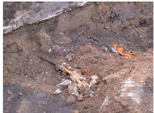
Plate 5: Concrete Footing and Chain from west
