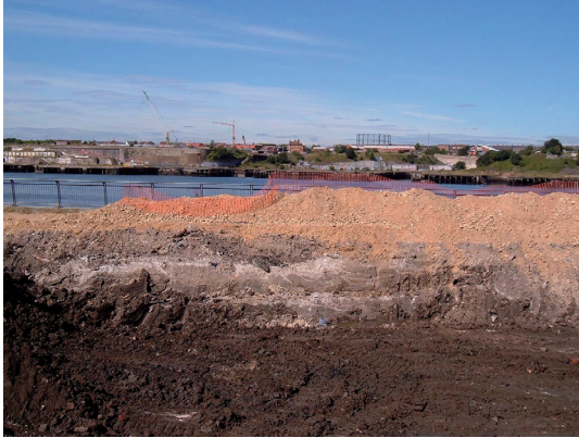
Plate 1: Eastern Concrete Structure from north-west
