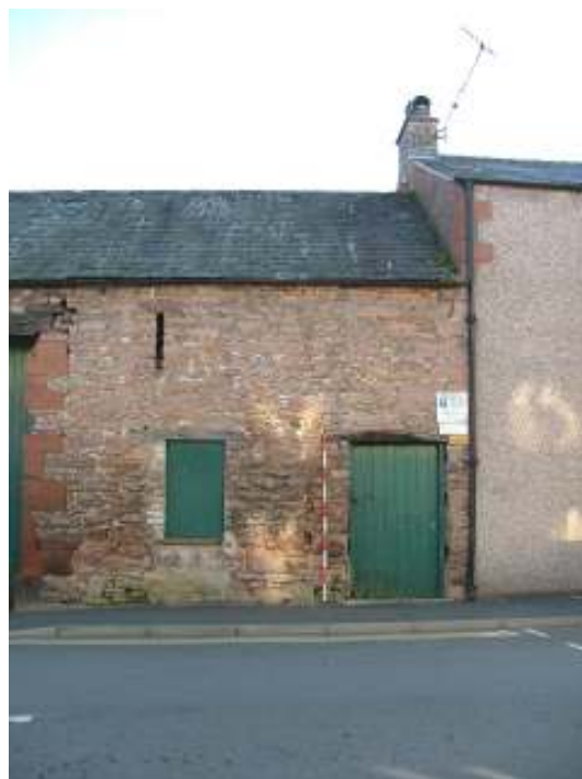
Plate 4 – Doorway, window and ventilation slits, west elevation
