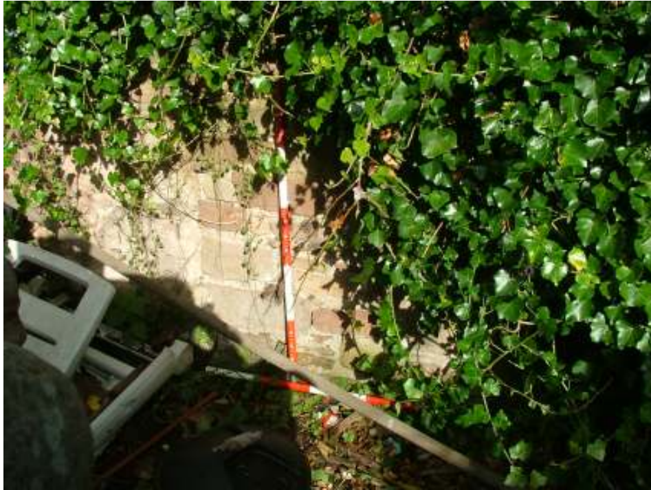
Figure 23 – Vertical construction break (left of ranging pole) possible blocked door in northern boundary wall of garden (Scales = 1m each)
