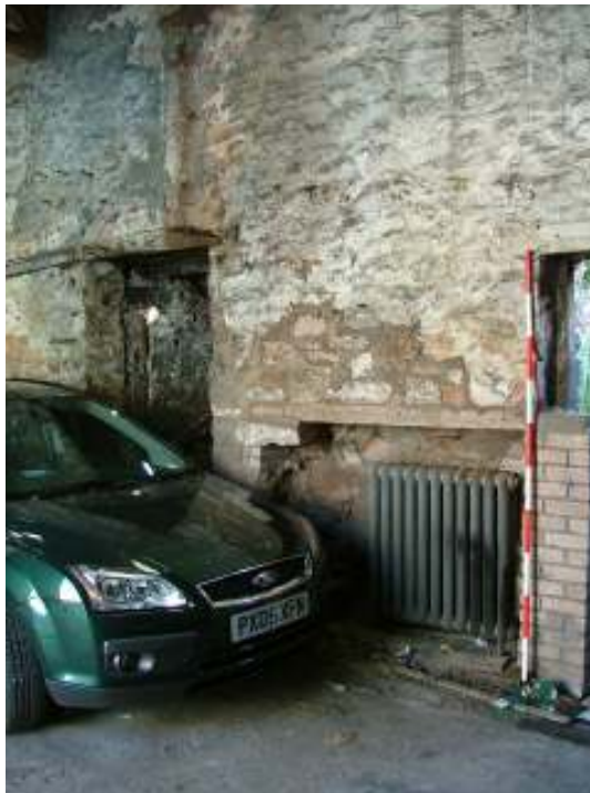
Plate 17 – Radiator inserted into wall in east elevation, to the left of this recess is the entrance to the outshut, above which a brown stain shows the location of the chimney above
