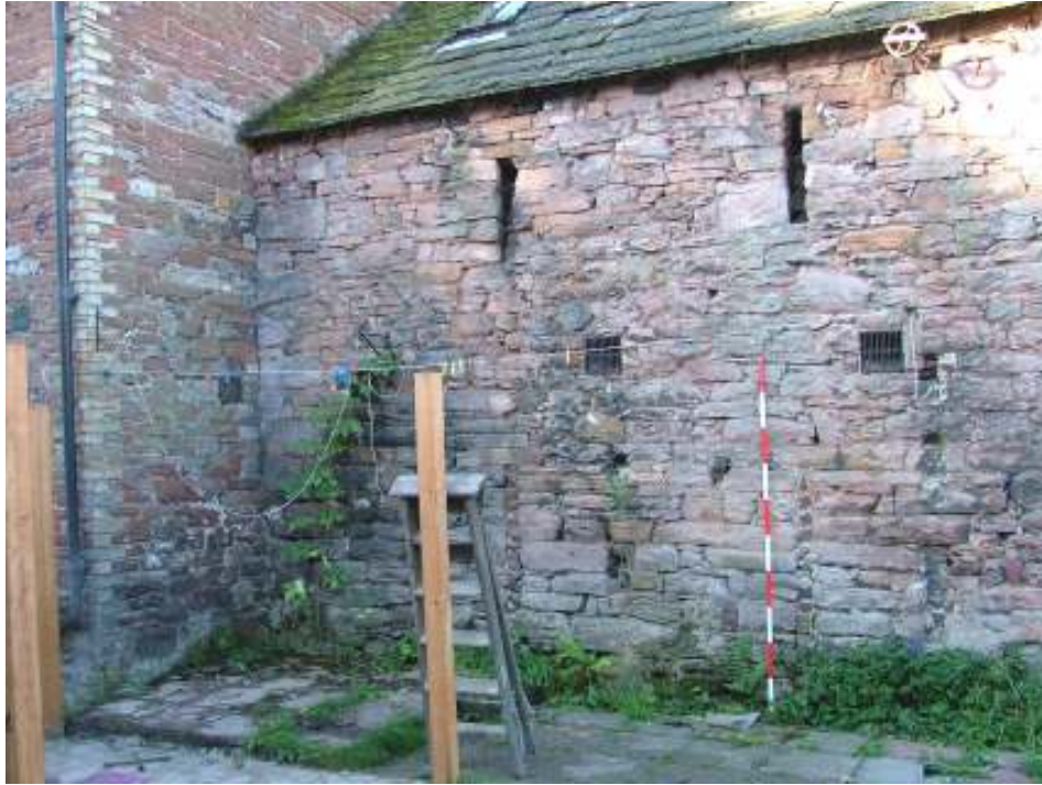
Plate 8 – South end of east elevation showing ventilation slits, square iron ventilators and vertical scarring from former lean-to? (Scale = 2m)
