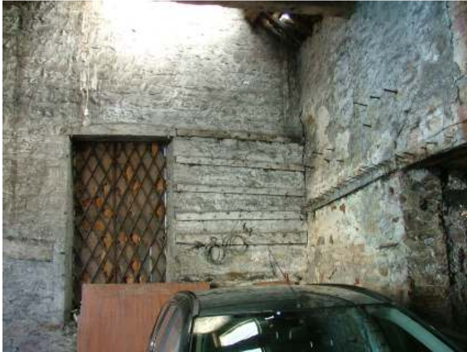
Plate 16 – Detail of iron framework in window (north elevation) and wooden battens fixed to wall
