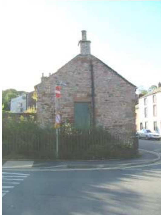
Plate 5 – North elevation showing possible former doorway with remains of blocked window above?
