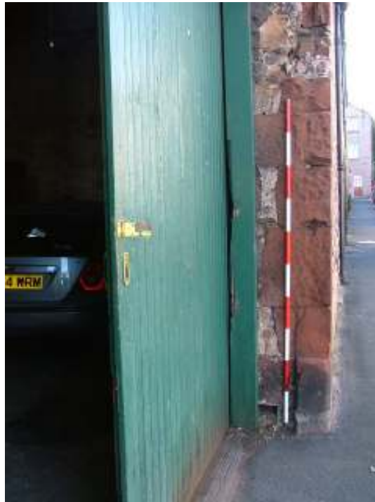
Plate 3 – Base of door jamb, west elevation, showing blocks which have been cutback, the block at the bottom of the jamb still retains its internal rebate and door hinge (Scale = 2m)
