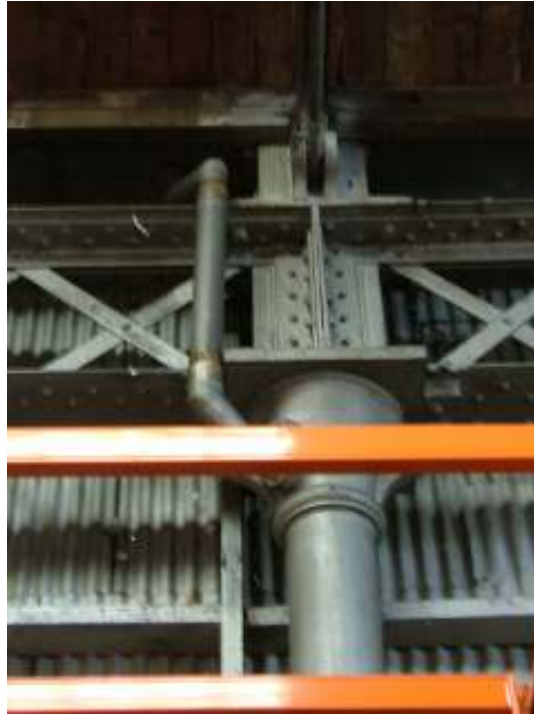
Plate 24 – Detail of the top of one of the columns showing latticework and pipe for rainwater
