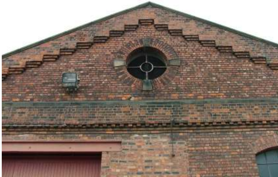
Plate 3 – Detail of circular window and decorative brickwork in south-east elevation
