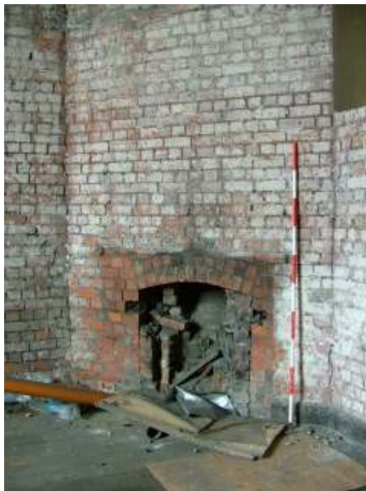
Plate 19 – Fireplace in NE office (Scale = 2m), this office still has its original floorboards
