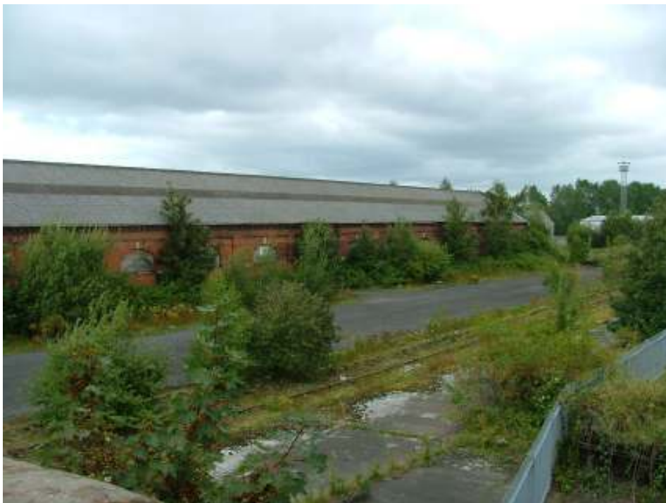
Plate 33 – South elevation of goods warehouse, view looking east
