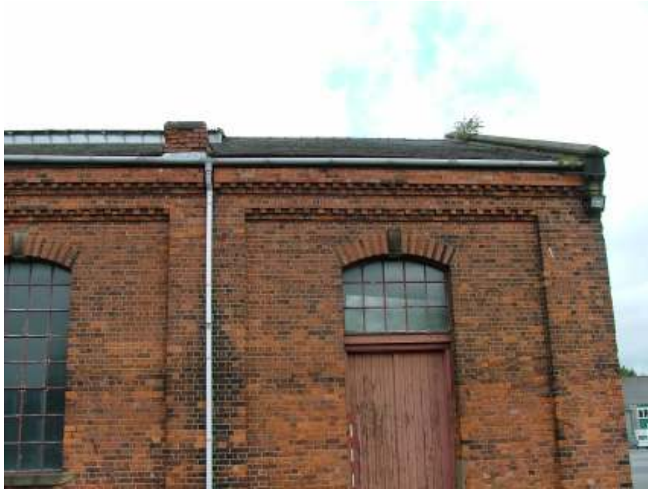
Plate 11 – Small chimney, south end of south-west elevation
