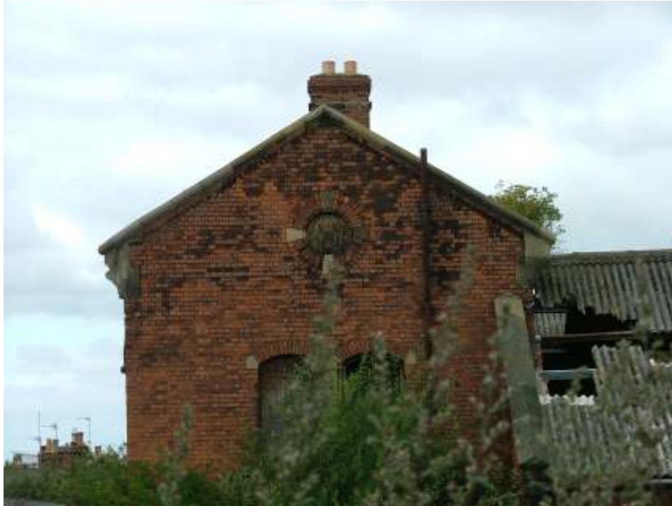
Plate 34 – South elevation of goods office building, west end of goods warehouse, with date stone '1881'
