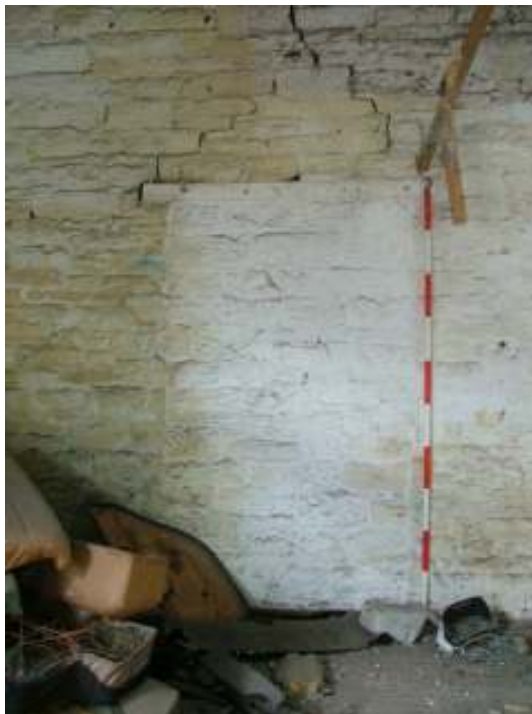
Plate 30 – Blocked doorway, south-west elevation of single-storey range (Scale = 2m)
