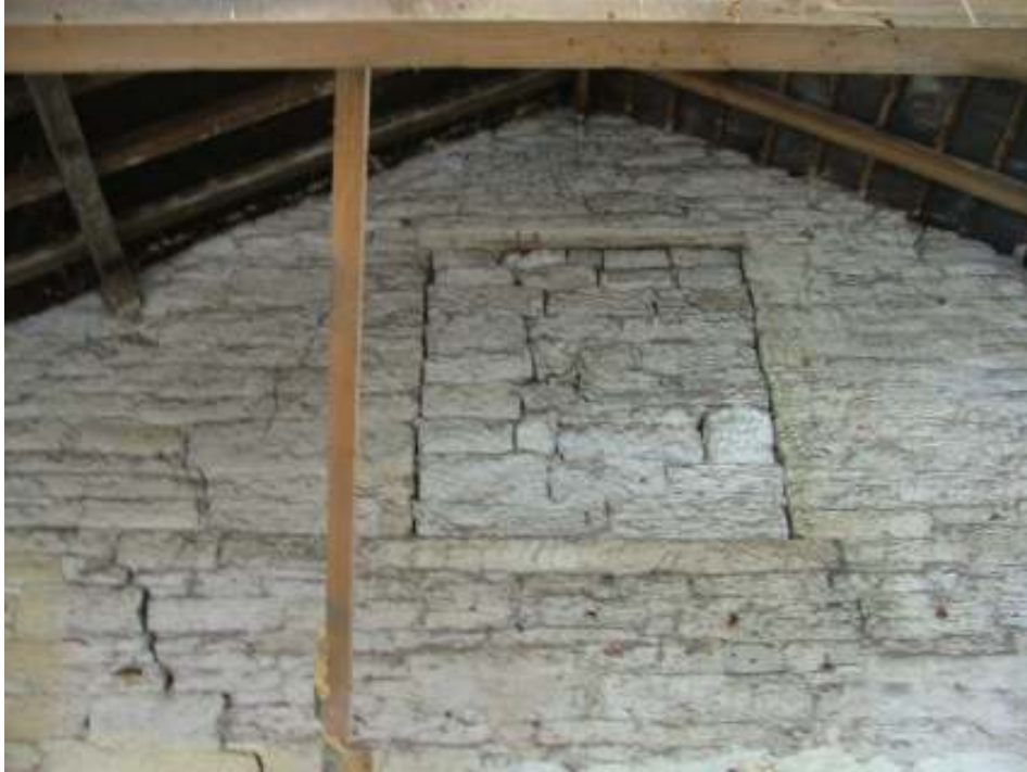
Plate 31 – Blocked-up window in south-west elevation
