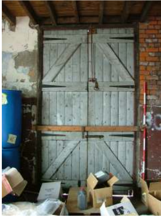
Plate 20 – Doorway to exterior, SW office in engine shed
