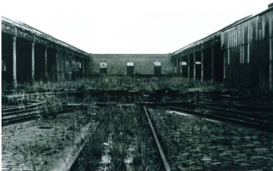
Figure 19 - View looking northwards of the interior of the engine shed in 1966 showing one of the turntables and tracks (Courtesy of Denis Perriam)
