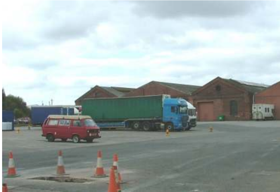
Plate 1 – The NER engine sheds as seen from the south-east
