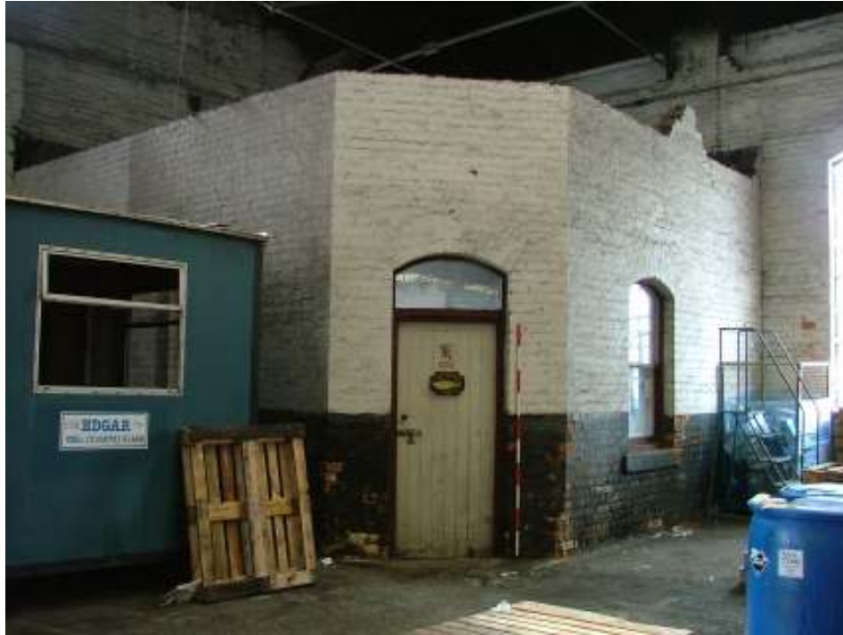
Plate 14 – Brick-built office in south-west corner of engine shed (Scale = 2m)
