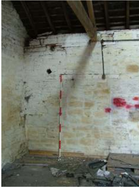
Plate 29 – Blocked-up doorway, interior of single-storey range (Scale = 2m)
