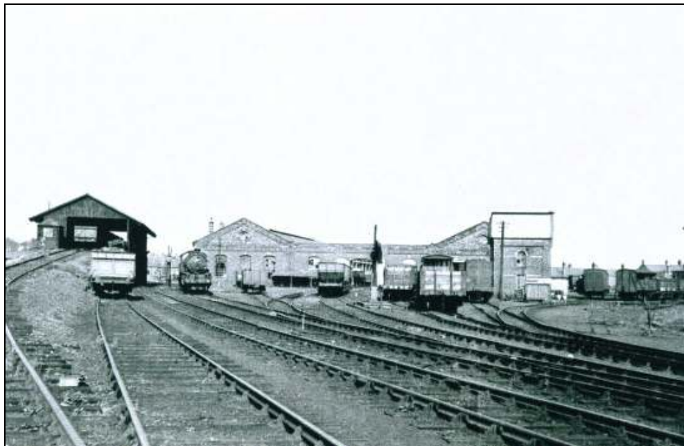
Figure 17 – 1951 photograph showing central section with roof missing, note the elevated coal depot to left of photograph and the brick-built water tower to the right (Courtesy of Denis Perriam)
