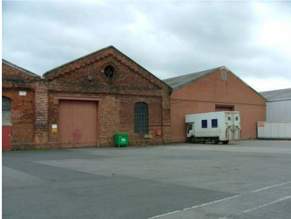
Plate 9 – South-east elevation showing modern building against eastern section of engine shed
