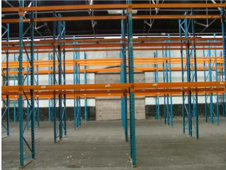
Plate 21 – Large blocked-up doorway in south-west elevation which originally provided access for the engines to the external turntable
