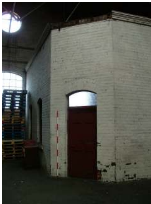
Plate 15 – Office in north-east corner of engine shed
