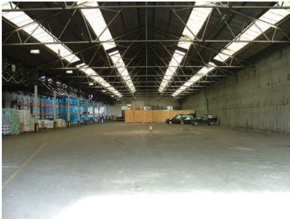
Plate 13 – View looking northwards of interior of central section of engine shed
