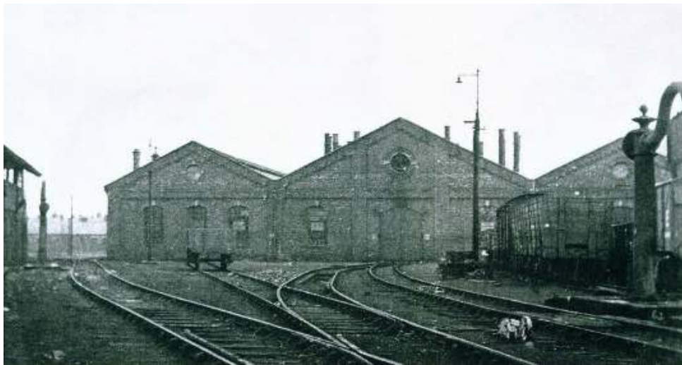
Figure 15 – Undated photograph, possibly pre-1933, showing central section with roof and projecting pipes (Courtesy of Denis Perriam)
