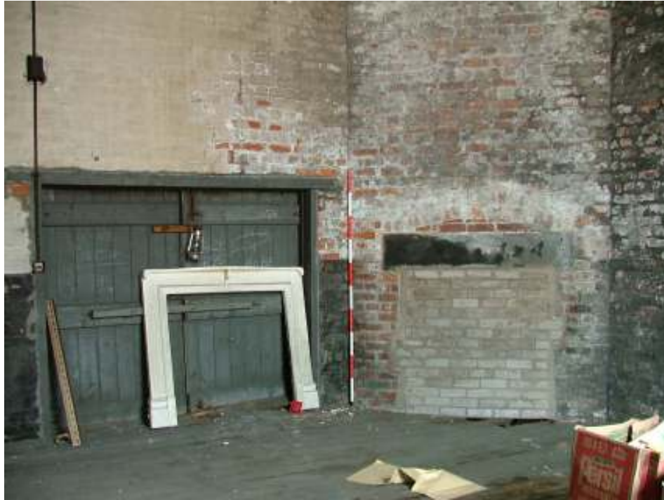
Plate 18 – Fireplace in NW office, note the insertion of a later lintel, the low doorway left of photograph and original floorboards (Scale = 2m)
