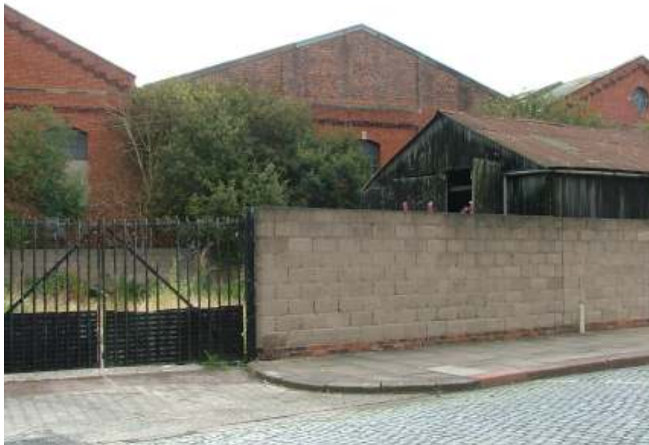
Plate 6 – North-west elevation as seen from Lindisfarne Street showing lack of decorative brickwork and circular window in central section of building
