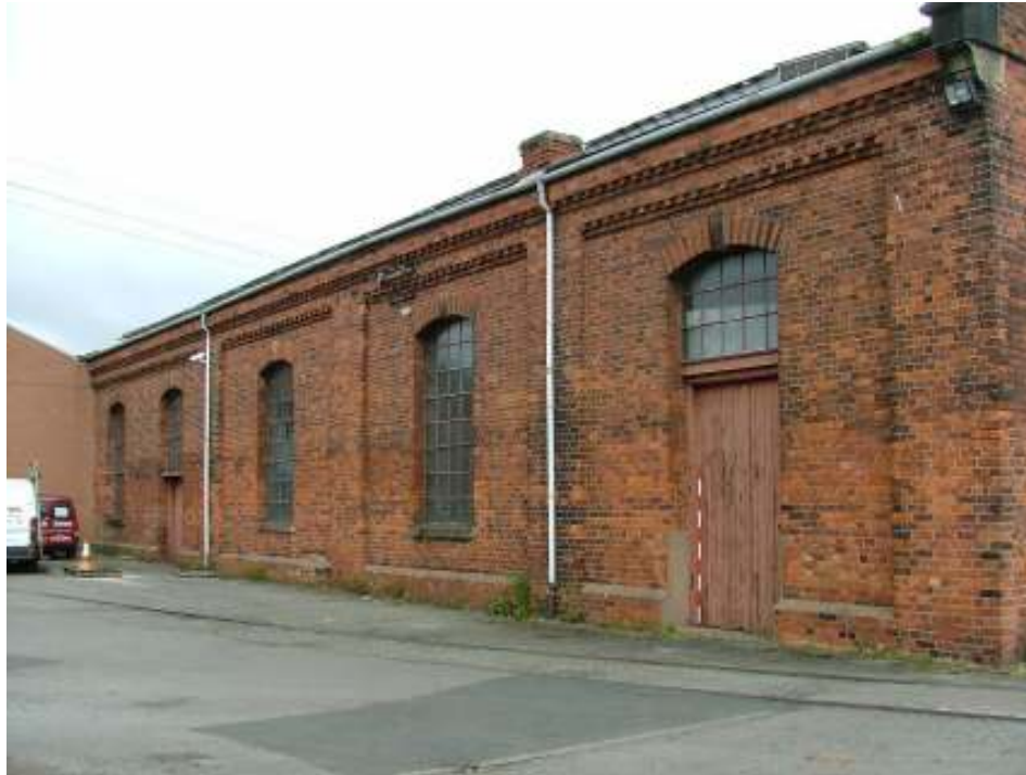
Plate 8 – South-west elevation showing modern building left of photograph and rail track in the foreground (Scale = 2m)
