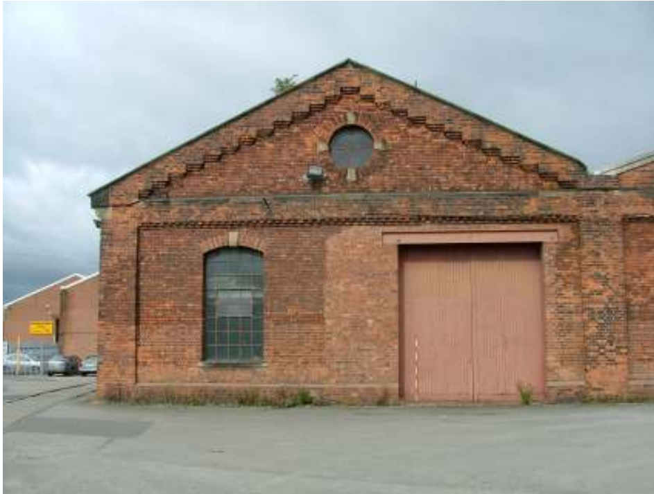
Plate 7 – Western section of south-east elevation showing inserted doorway (Scale = 2 metres)
