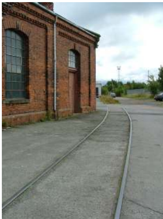
Plate 12 – View looking south-east showing rail track which runs past the south-west corner of the engine shed
