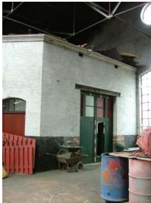
Plate 17 – Inserted doorway, office in north-west corner of engine shed
