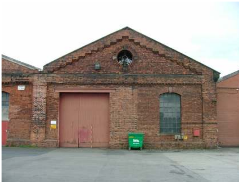
Plate 2 – South-east elevation showing one of the three gables with recessed brickwork, and decorative crow-step defining the gable which contains a circular window
