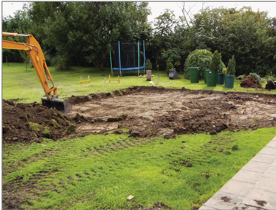
Plate 1. The site, looking south, during excavation.
