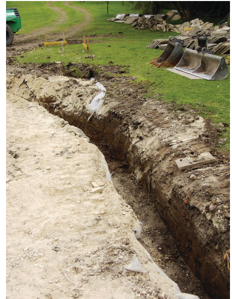
Plate 5. Foundation trench, looking east at curve of patio wall.
