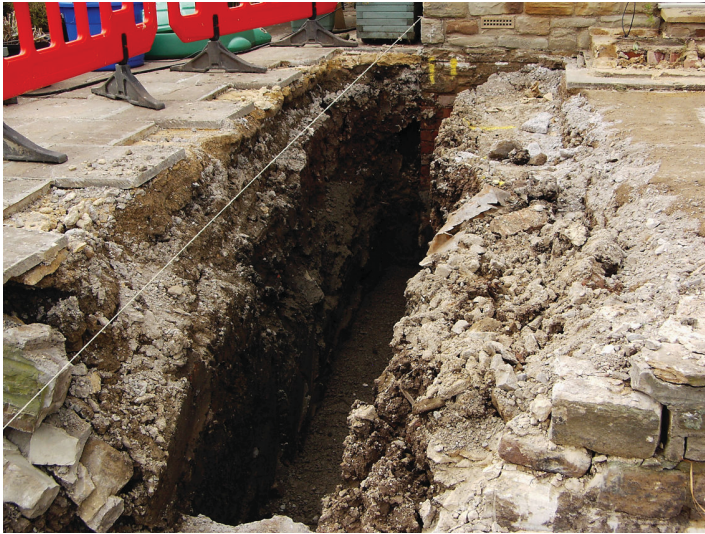
Plate 4. Foundation trench looking back west towards York House.
