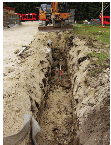
Plate 7. Looking north during foundation excavation.
