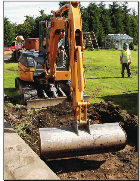
Plate 3. Site under excavation.
