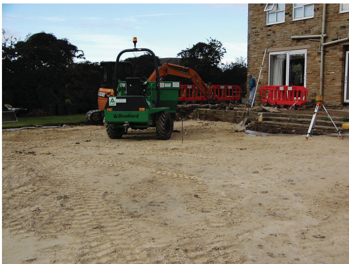
Plate 6. During excavation through current patio.
