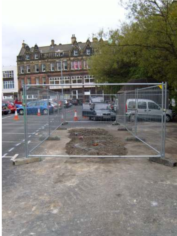
Plate 12. Trench 3 after backfilling.
