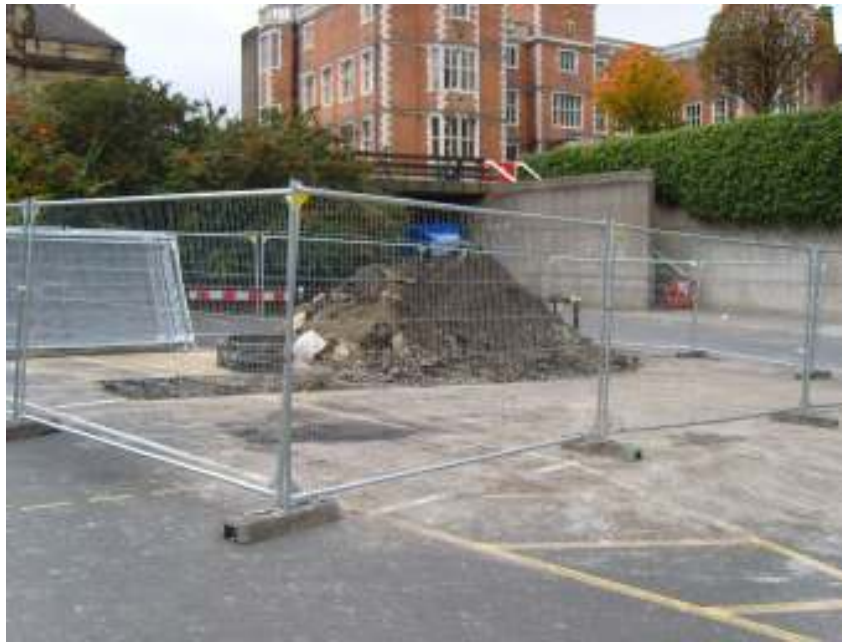
Plate 10. Trench 1 after backfilling.
