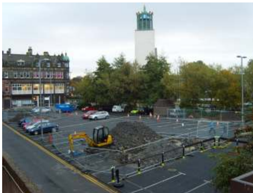
Plate 1. Trench 1 in the foreground after excavation.
