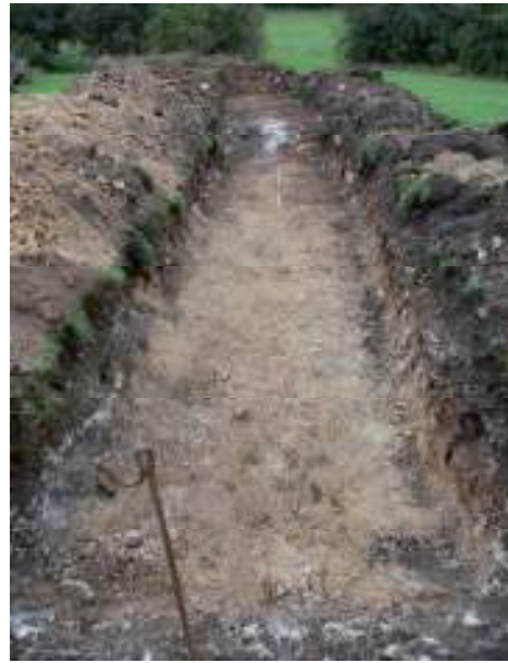
Plate 9: View of Trench 2 after machining looking northeast.
