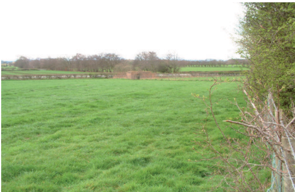
Plate 1: Small brick built building in Area A, facing west
