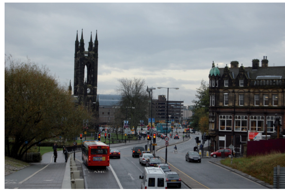
Plate 7: View of Barras Bridge from the north
