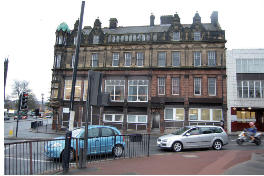
Plate 11: View of Claremont Building from north
