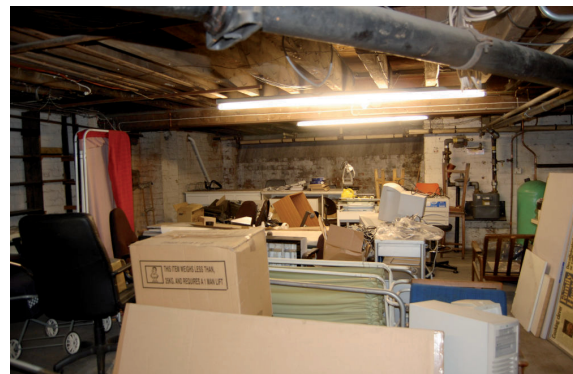
Plate 9: View of western room in cellar beneath Barras Building
