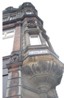
Plate 8: View of 'Eldon Place' Sign on southern turret
