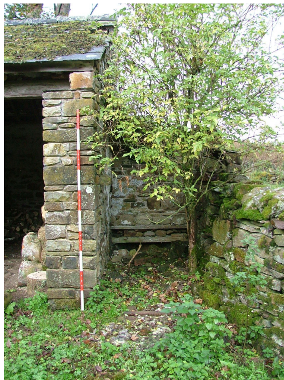
Plate 31 – Remains of privy to right of cart shed/store
