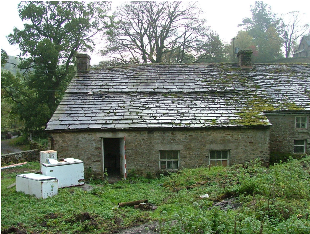
Plate 11 – North elevation of outshut
