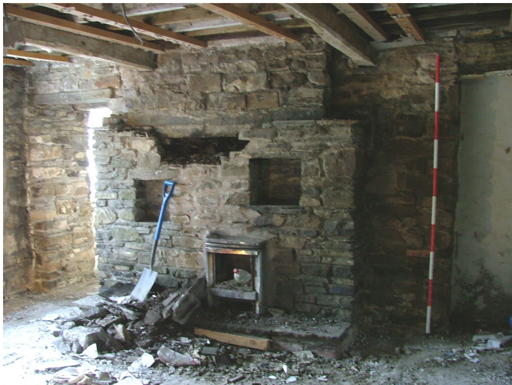
Plate 20 – Modern fireplace, Room 3, ground floor, with blocked doorway to right of ranging pole
