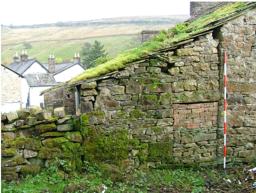
Plate 16 – West elevation, blocked aperture in outshut (Scale =2m)
