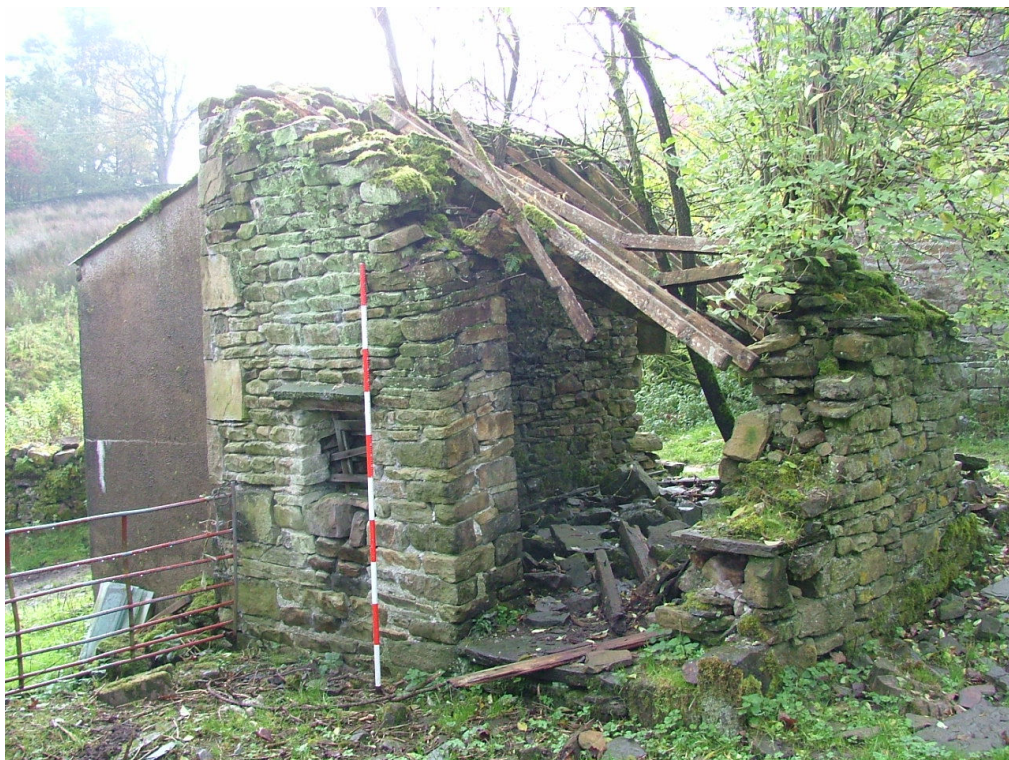
Plate 33 – Building to west of house, east and north elevations
