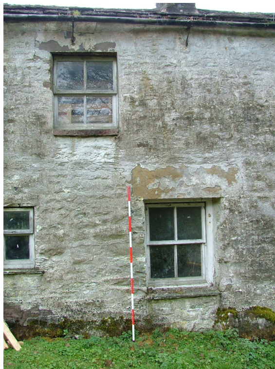
Plate 7 – Window, south elevation, was possible former doorway (Scale = 2m)
