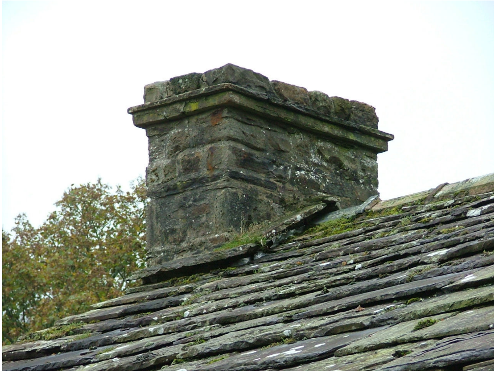
Plate 17 – Detail of chimney on eastern gable end
