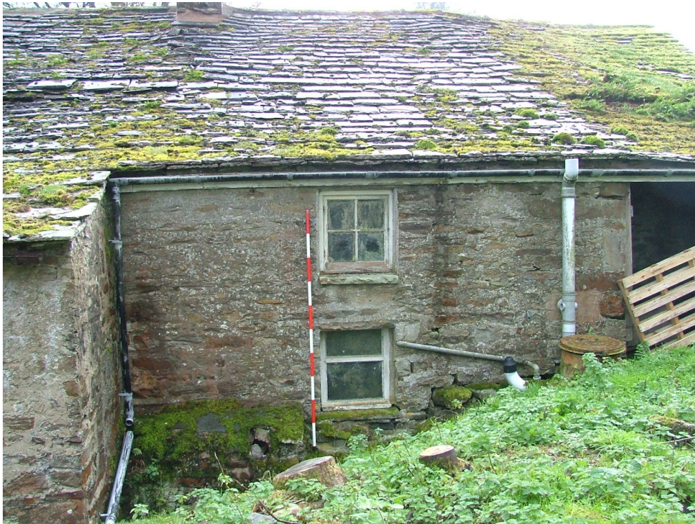
Plate 13 – North elevation of small outshut, rear of house (Scale = 2m)
