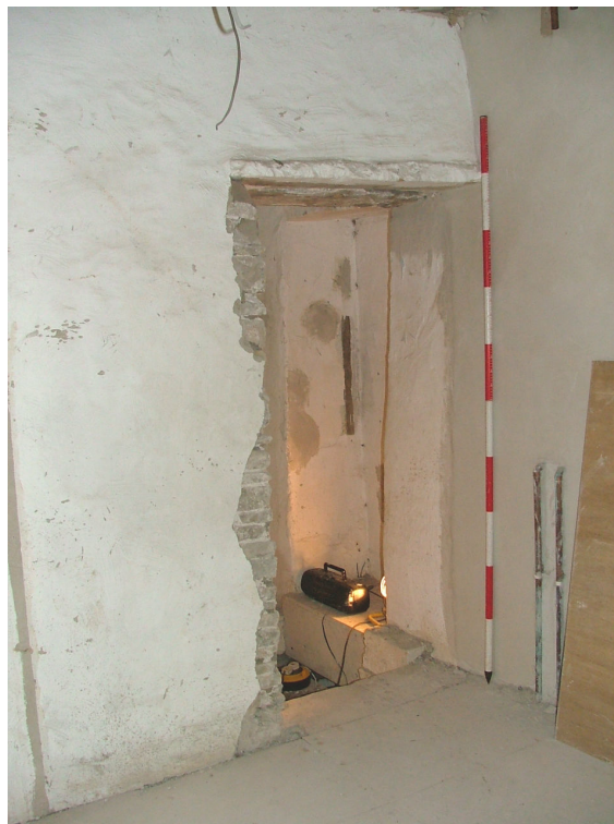
Plate 25 – Doorway between room over (2) and top of stairwell (1) (Scale = 2m)
