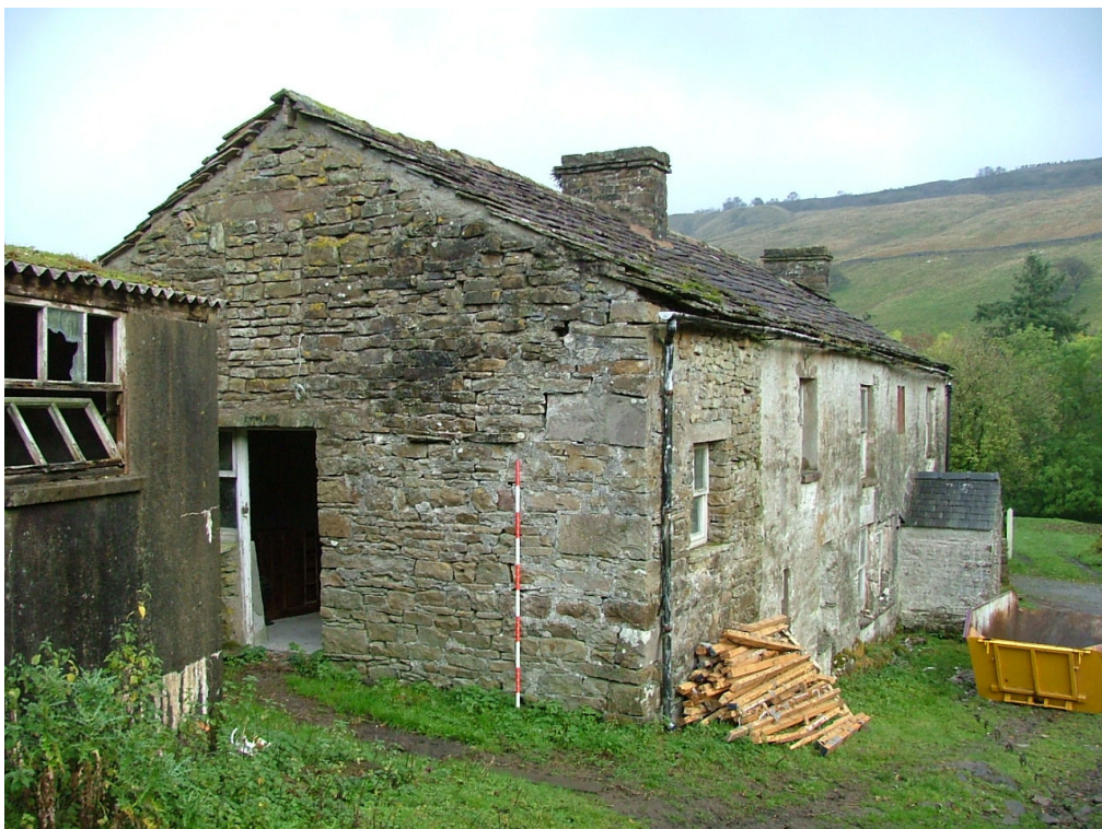
Plate 23 – West and south elevations, view showing the increased height of the western end of the property compared to the rest (Scale = 2m)
