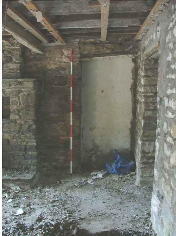
Plate 21 – Blocked doorway, beside fireplace in ground floor room (3) (Scale = 2m)
