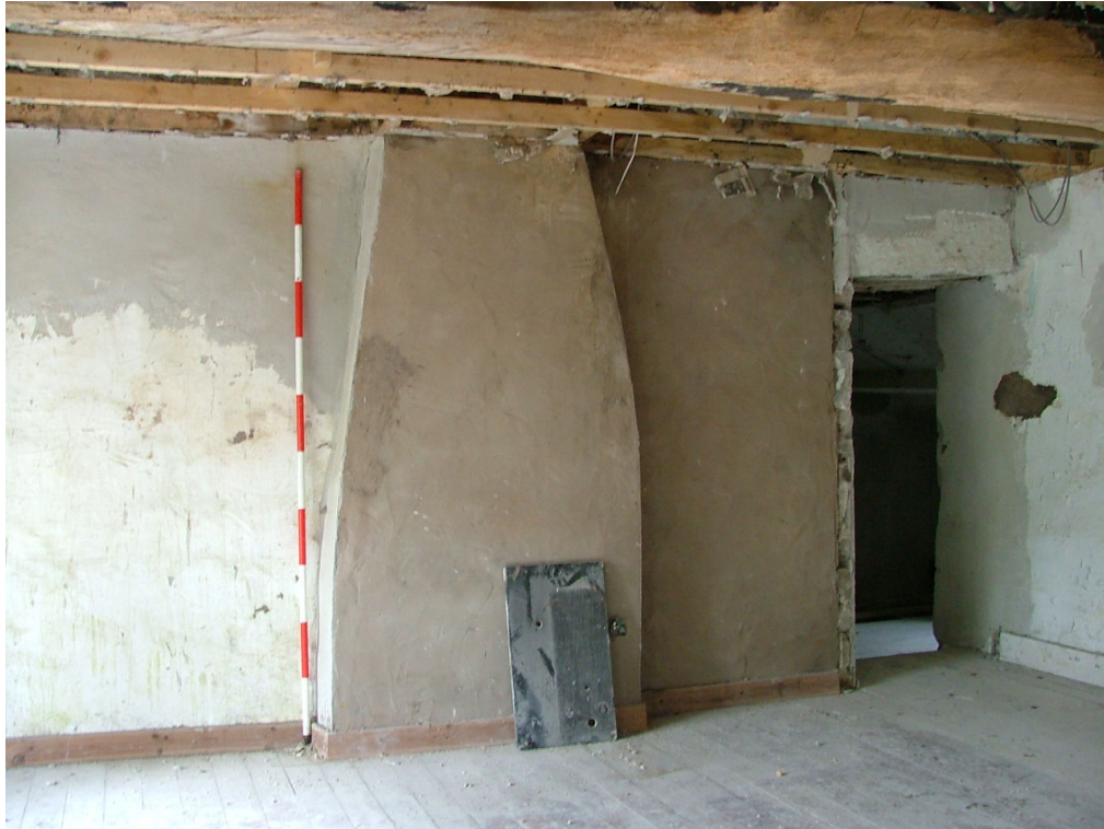
Plate 26 – Chimney breast, first floor over Room (3), view looking west
