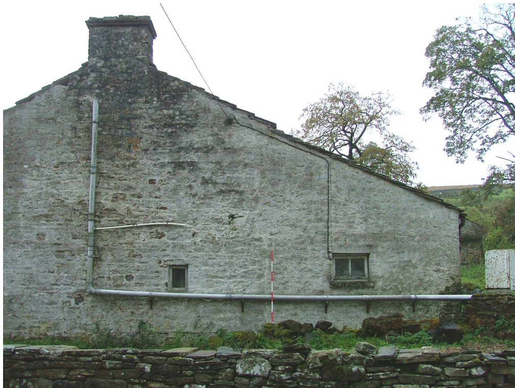
Plate 10 – East elevation showing main body of house to left, and addition of outshut to right. The vertical construction break between the two is just to the left of the ranging pole
