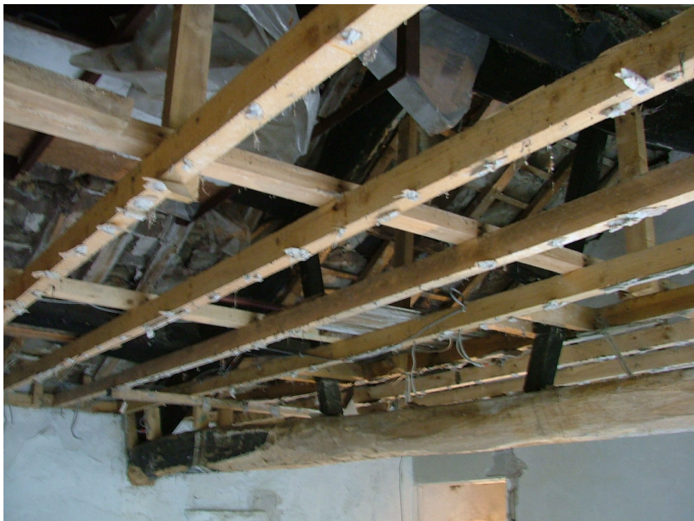
Plate 29 – Roof truss, first floor room over (3)
