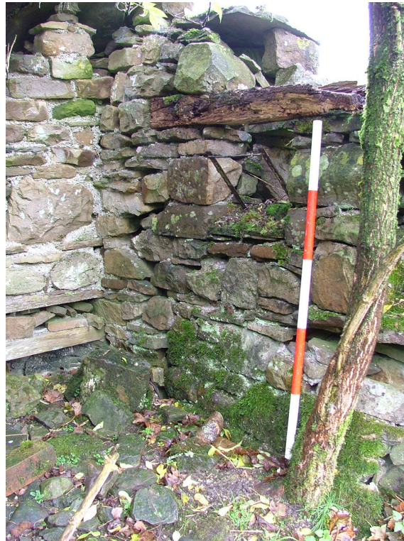
Plate 32 – Eastern wall of privy showing iron window frame and timber lintel (Scale = 1m)
