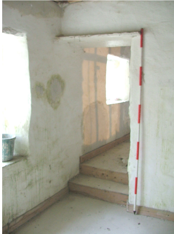
Plate 24 – Doorway between rooms over (2) and (3), first floor
