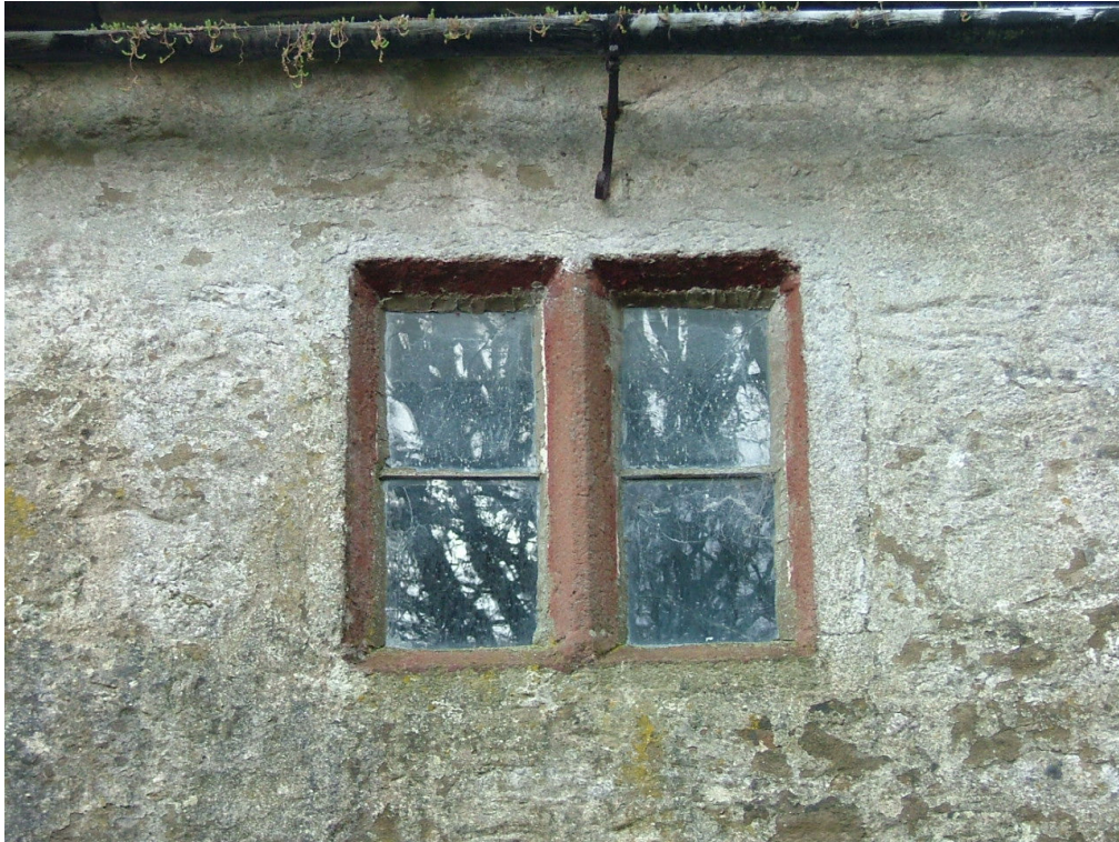
Plate 8 – Two-light, chamfered mullion window, first floor, south elevation
