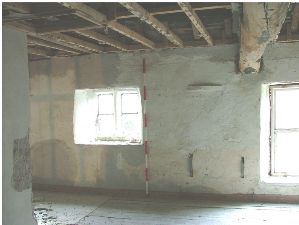
Plate 27 – Windows and through-stone in south elevation, first floor
