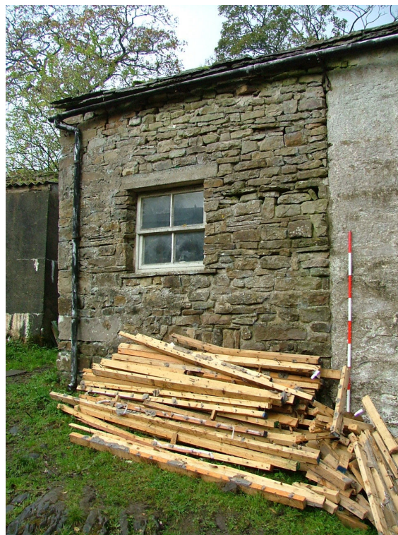
Plate 9 – West end of house, south elevation
