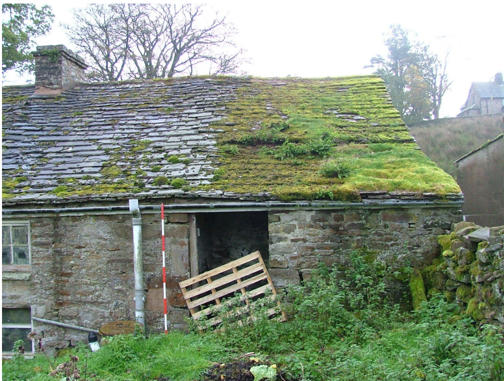
Plate 14 – North elevation, western end showing door to possible turf house?
