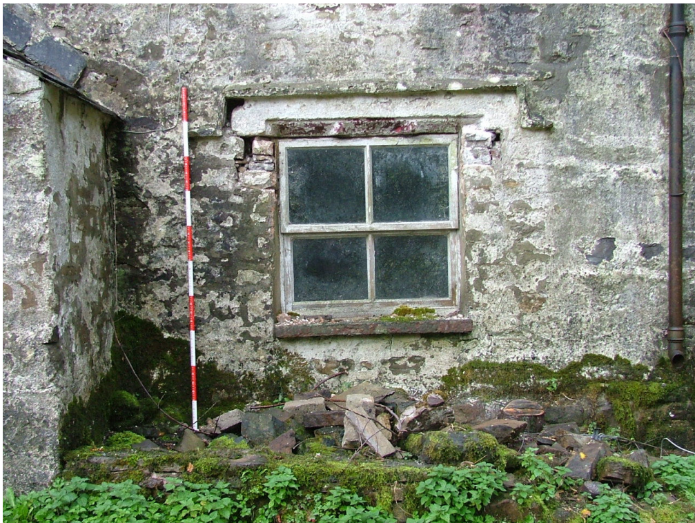
Plate 5 – Ground floor window to right of porch on south elevation, showing earlier 3-light mullioned window and hoodmould (Scale = 2m)
