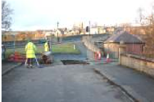
Plate 3: Trench location, facing northwest
