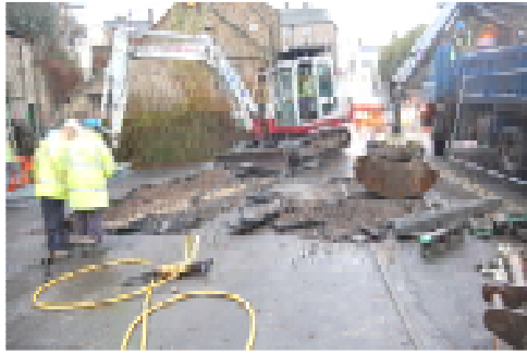
Plate 5: Excavation of trench, facing north
