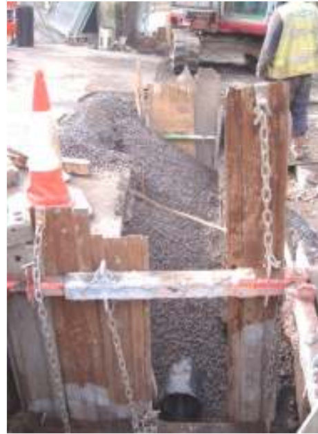
Plate 22: Trench backfill, facing south
