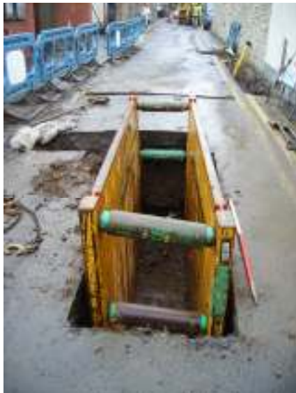
Plate 1: Test pit 1, facing north
