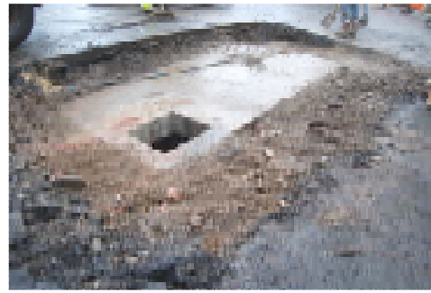
Plate 6: Existing concrete tank
