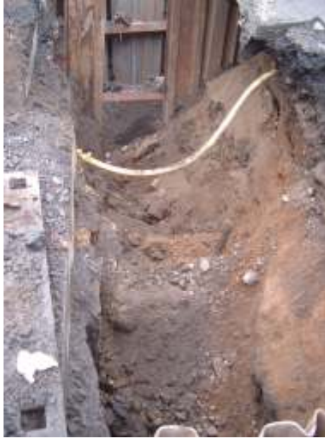
Plate 21: Trench excavation, facing north
