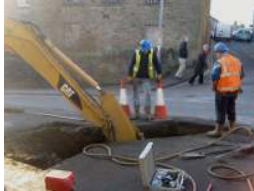
Plate 8: Excavation of trench, facing east
