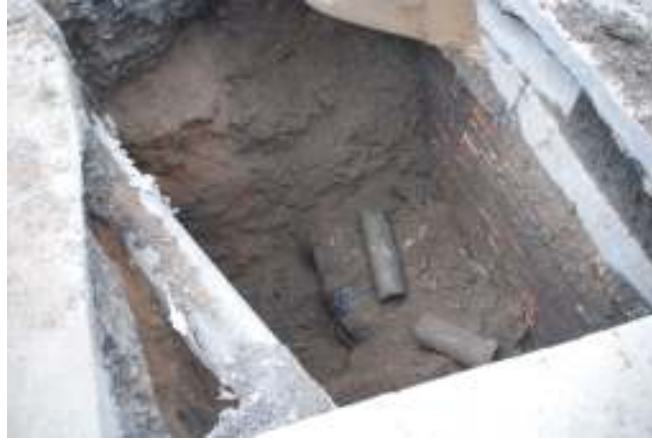
Plate 15: Excavation trench, note brick and concrete structure
