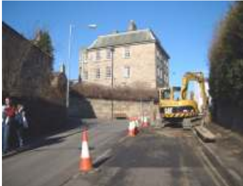
Plate 7: Trench location, facing north
