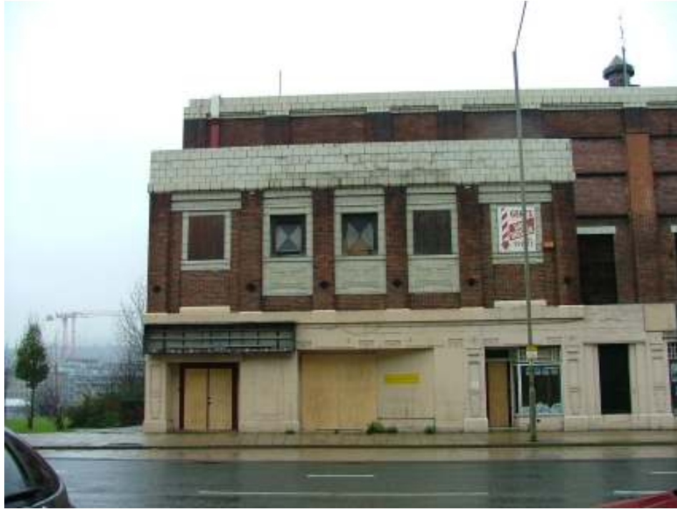
Plate 7 – South elevation showing coloured glass within the first floor windows
