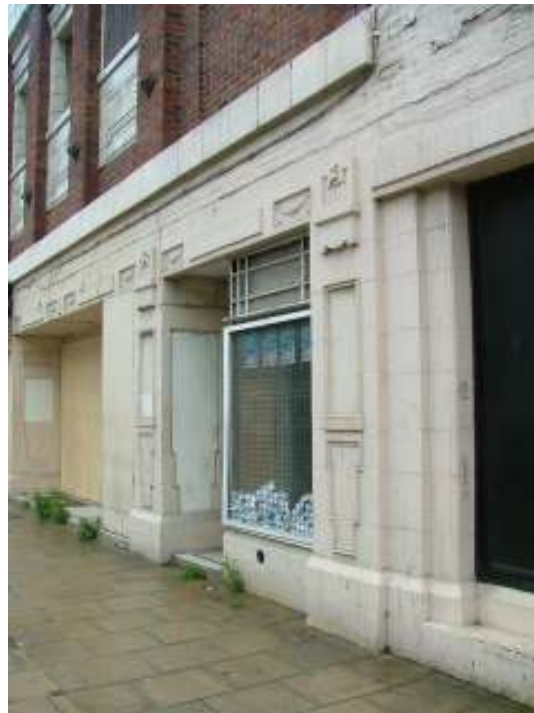
Plate 4 – South elevation, view of the cream, faience tiling and architectural detail such as the 'swags' over the windows and doors
