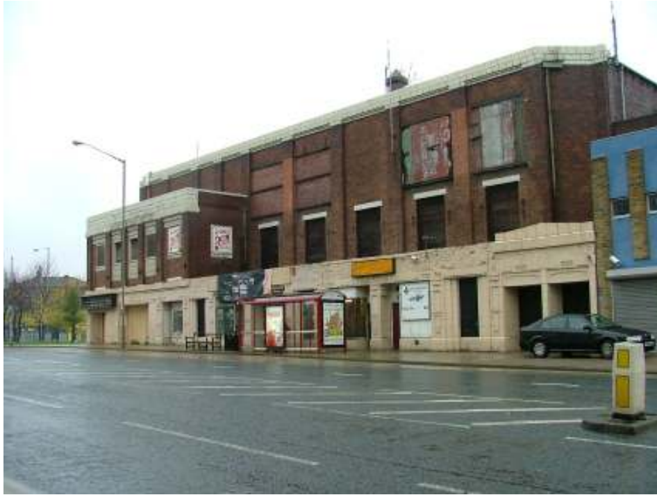
Plate 1 – South elevation facing Briggate
