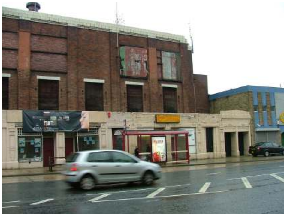
Plate 13 – View looking north-east showing the east end of the south elevation and the two-storey projection from the east elevation
