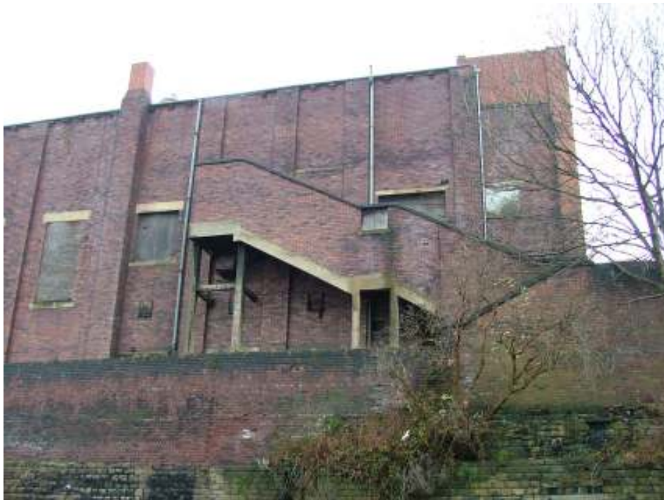
Plate 11 – External staircase, north elevation
