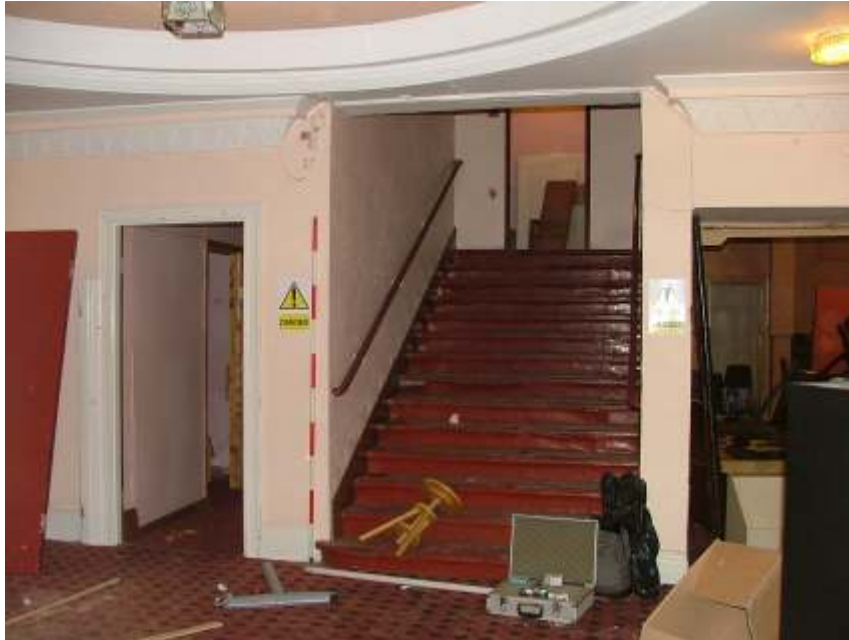
Plate 14 – View from the ground floor foyer of the staircase to the balcony, the doorway to the right provided access to the main auditorium and the door to the left provided access to an office and storage space beneath the stairs
