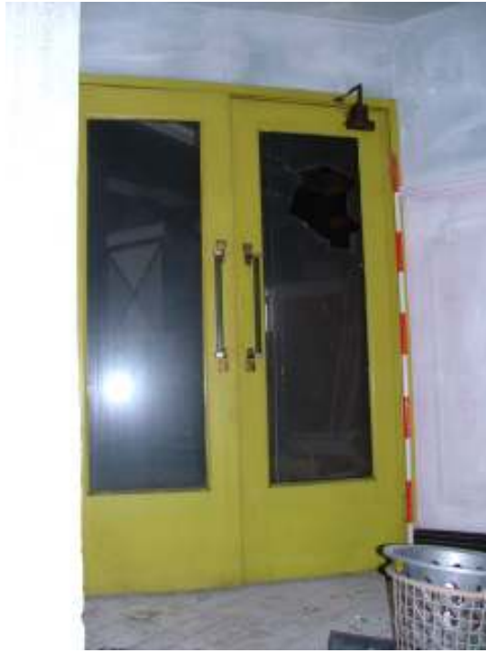
Plate 28 – Double doors at top of stairs to balcony foyer (Scale = 2m)
