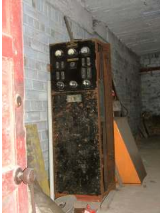
Plate 47 – Machinery remaining in-situ in the basement, note the concrete ceiling
