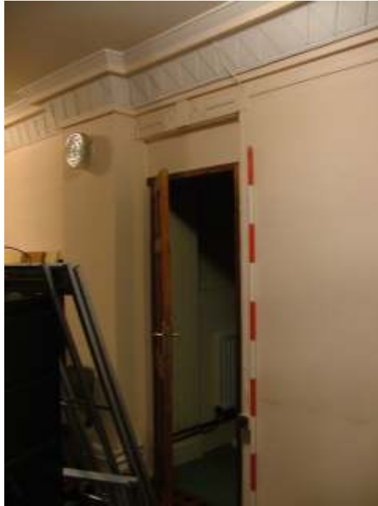
Plate 18 – Door to former sweet/tobacco shop from foyer
