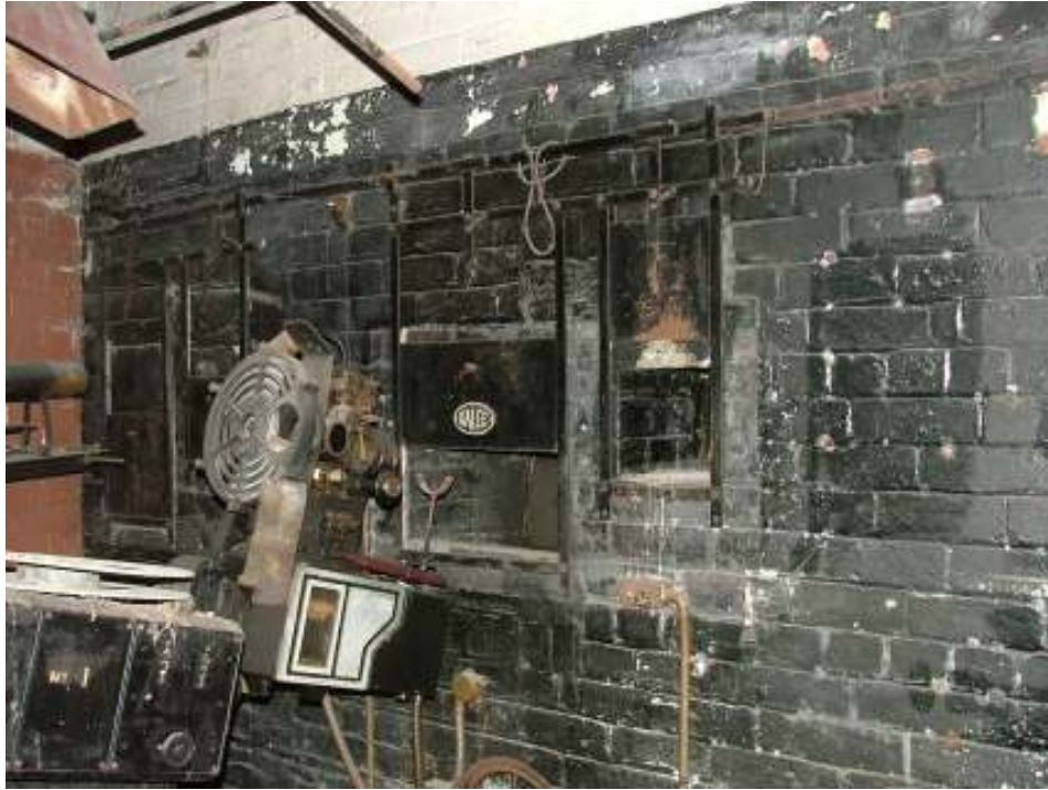
Plate 44 – Holes with shutters within the brick wall for projecting the films and observing the audience
