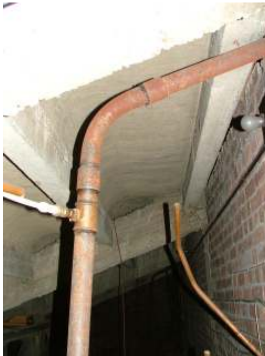
Plate 41 – View of the underneath of the balcony showing the curved concrete
