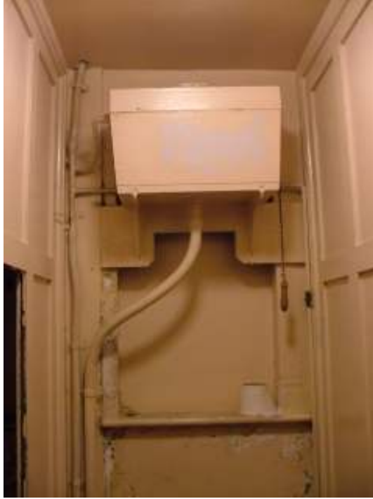
Plate 26 – Detail of cistern, ladies toilets, ground floor
