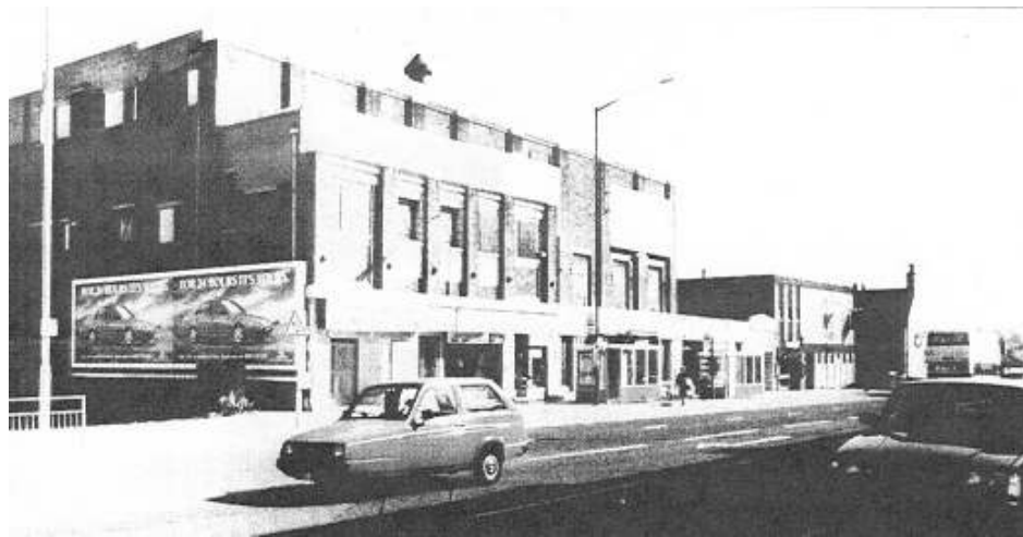
Figure 10 – Glenroyal Buildings 1983 (Source: Firth 1996)
