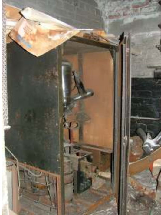
Plate 45 – Machinery in room to south of the projection room
