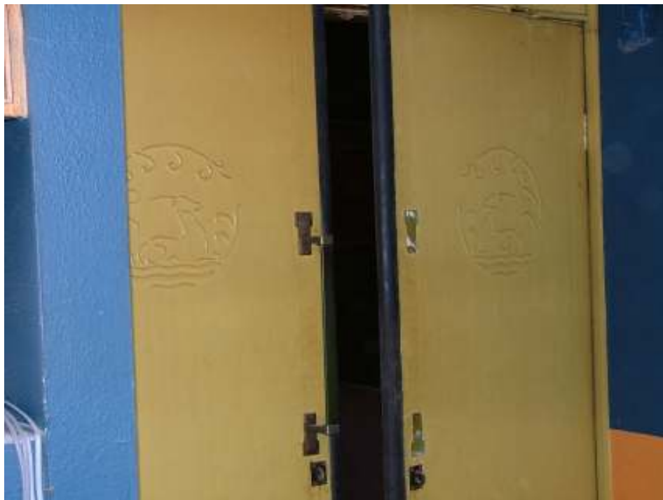
Plate 33 – Doors to balcony with circular motifs containing a deer
