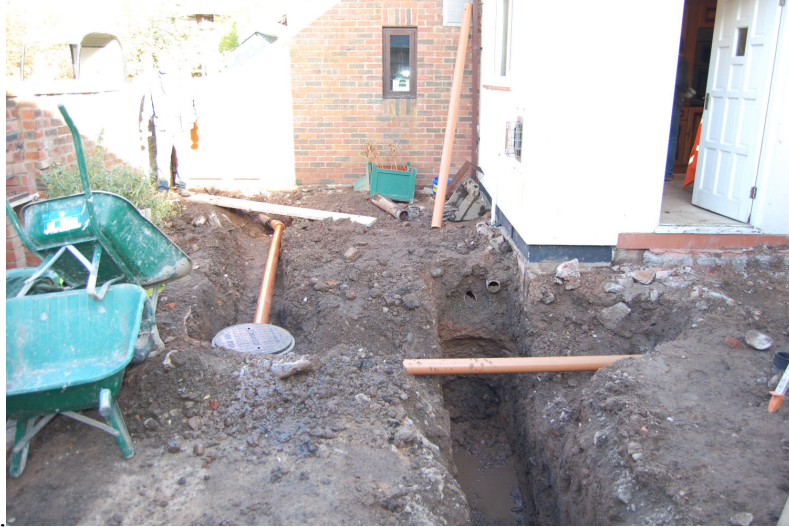
Plate 6: Trench 3 (on the left), with new waste pipe installed.
