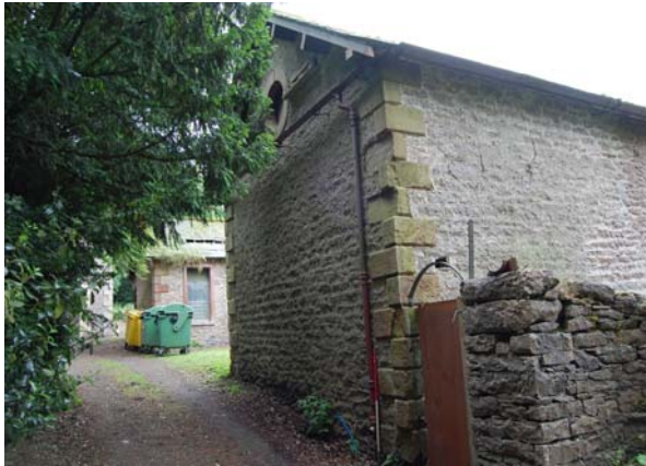
Plate 11: Stable building, facing west
