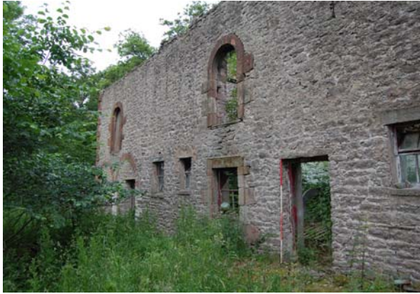
Plate 17: External elevation, facing east
