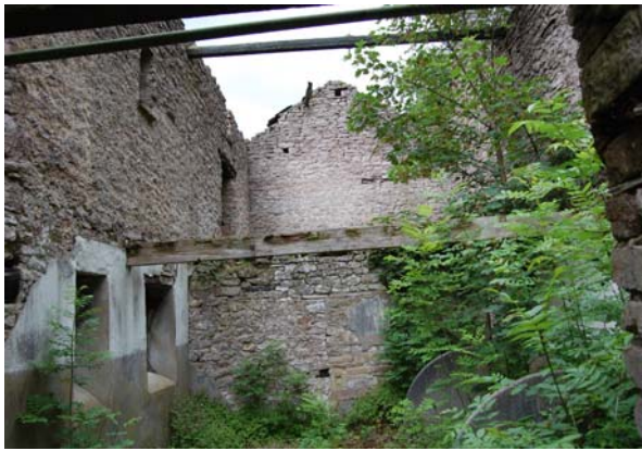
Plate 19: Internal walls, facing east
