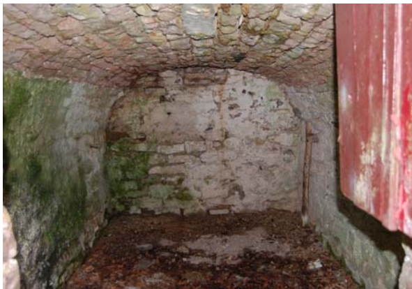
Plate 15: Stable building, internal arched ceiling
