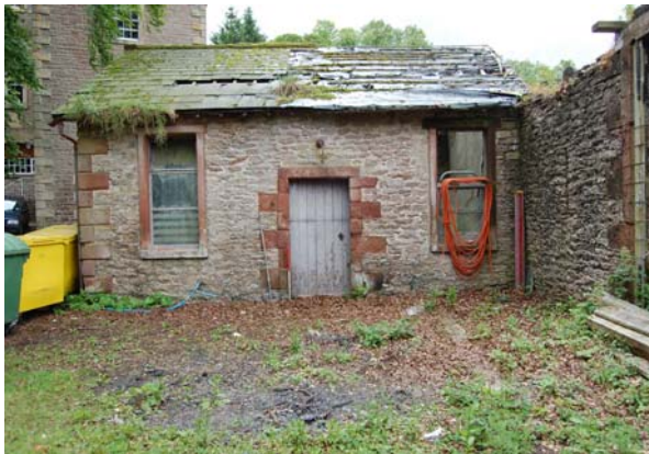
Plate 13: Stable building, facing west
