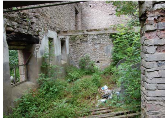
Plate 20: Internal walls, facing east
