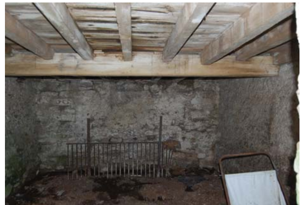
Plate 16: Stable building, internal room
