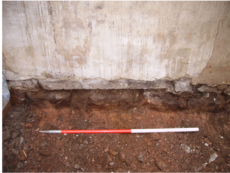
Plate 9: Internal foundation stones lying on the natural substrata
