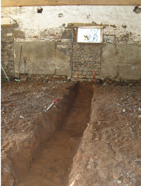
Plate 1: Barn A, foundation trench 2 inside the building
