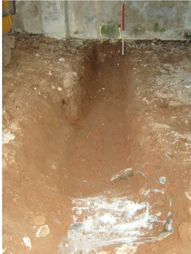
Plate 4: Excavation of trench 4, inside Barn A
