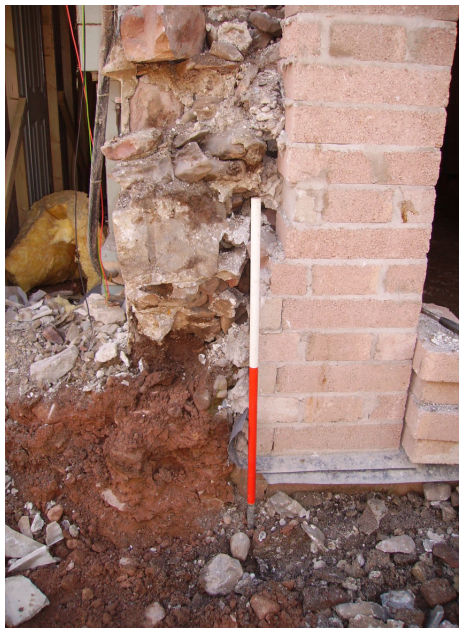
Plate 8: Barn A, an original stone dividing wall (on left) lying on the light brown/orange natural soil horizon
