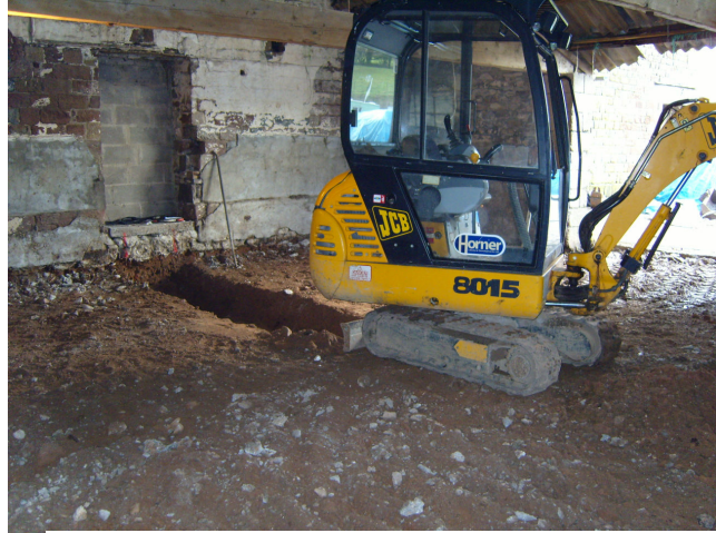
Plate 2: Excavation of trench 2, inside Barn A
