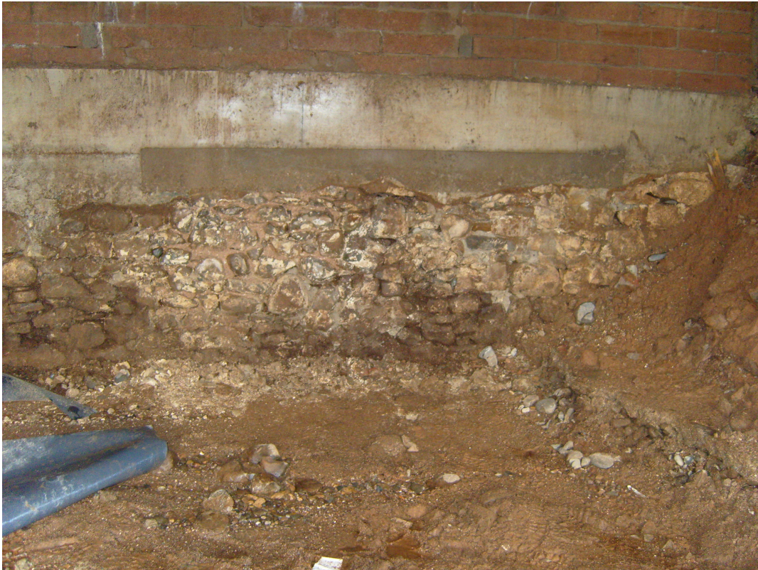
Plate 11: Original dividing wall, in Barn B
