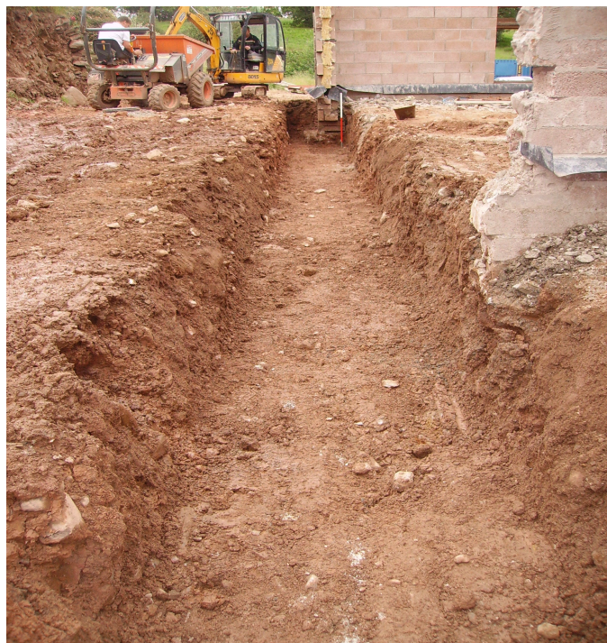
Plate 10: Foundation trench 5 along the line of the rear wall
